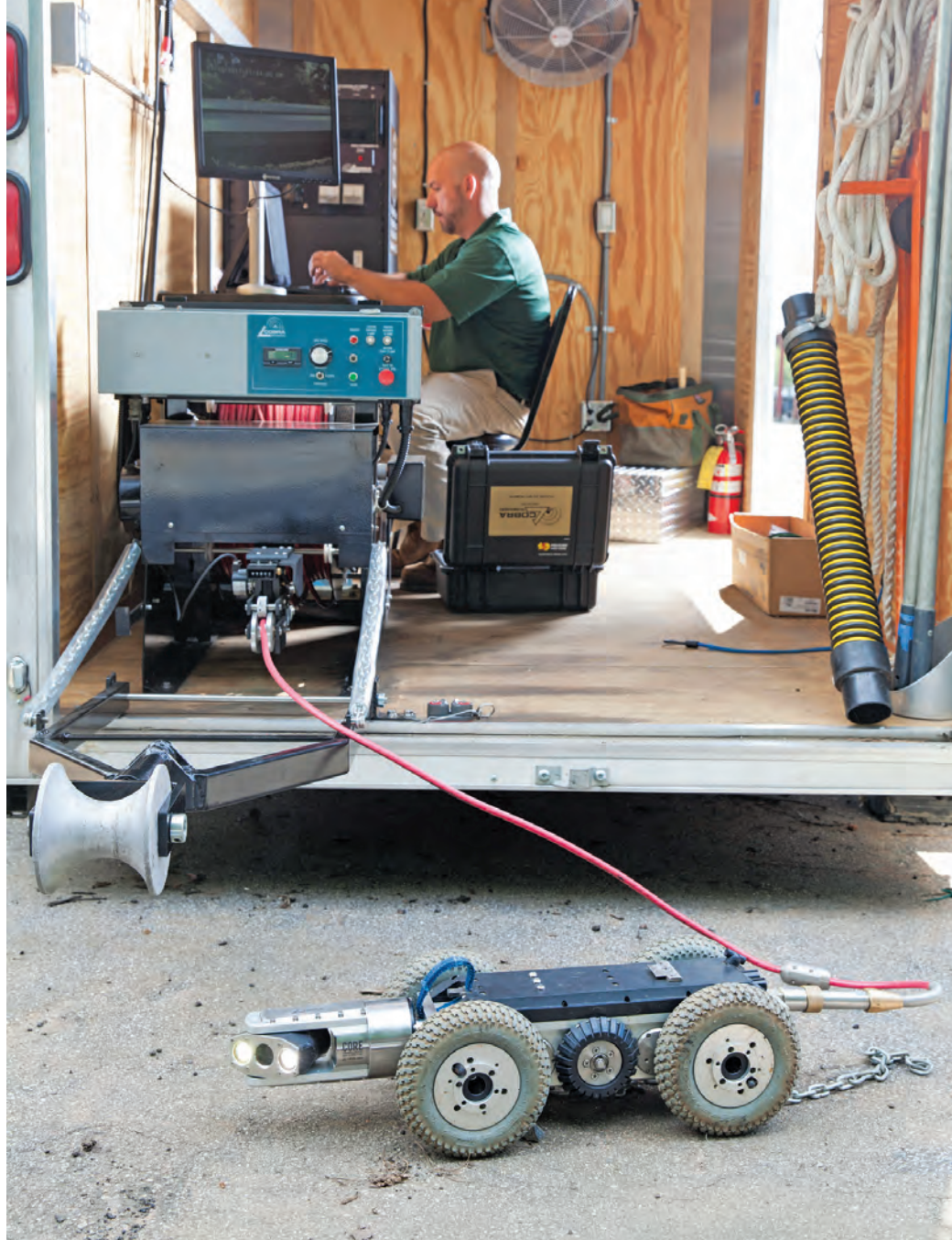
Public Works Supervisor Dennis Roland works in an inspection trailer designed by Cobra Technologies equipped with a V9 pan/tilt/zoom camera attached to an 806 steerable crawler and 500 feet of cable. The new camera and crawler can get over more obstacles in pipes than the division’s previous equipment.
