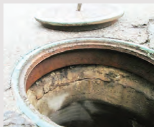
Concrete ADJ Rings Installed 1997
