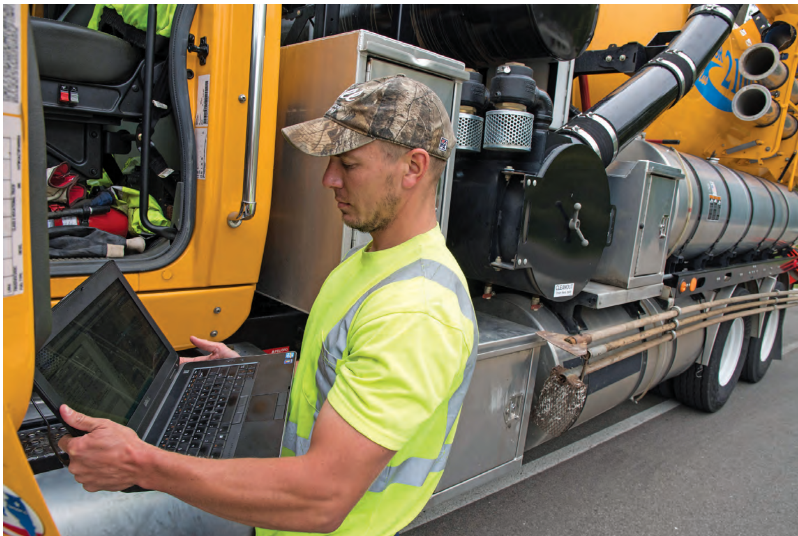
Technician Kyle Kelley checks asset information on his laptop while setting up to clean a sewer line with a Vactor 2100 Plus combination truck.
