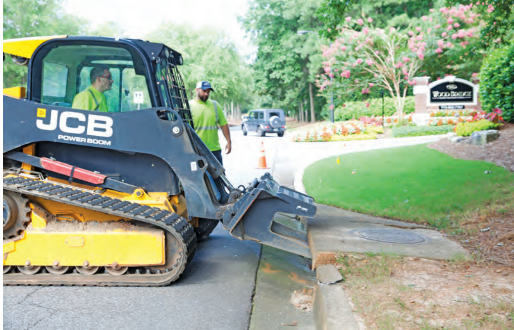
Public Works technician Louis Perriello uses a JCB PowerBoom to remove a damaged storm drain cover while crew leader Jared Wilson directs.
