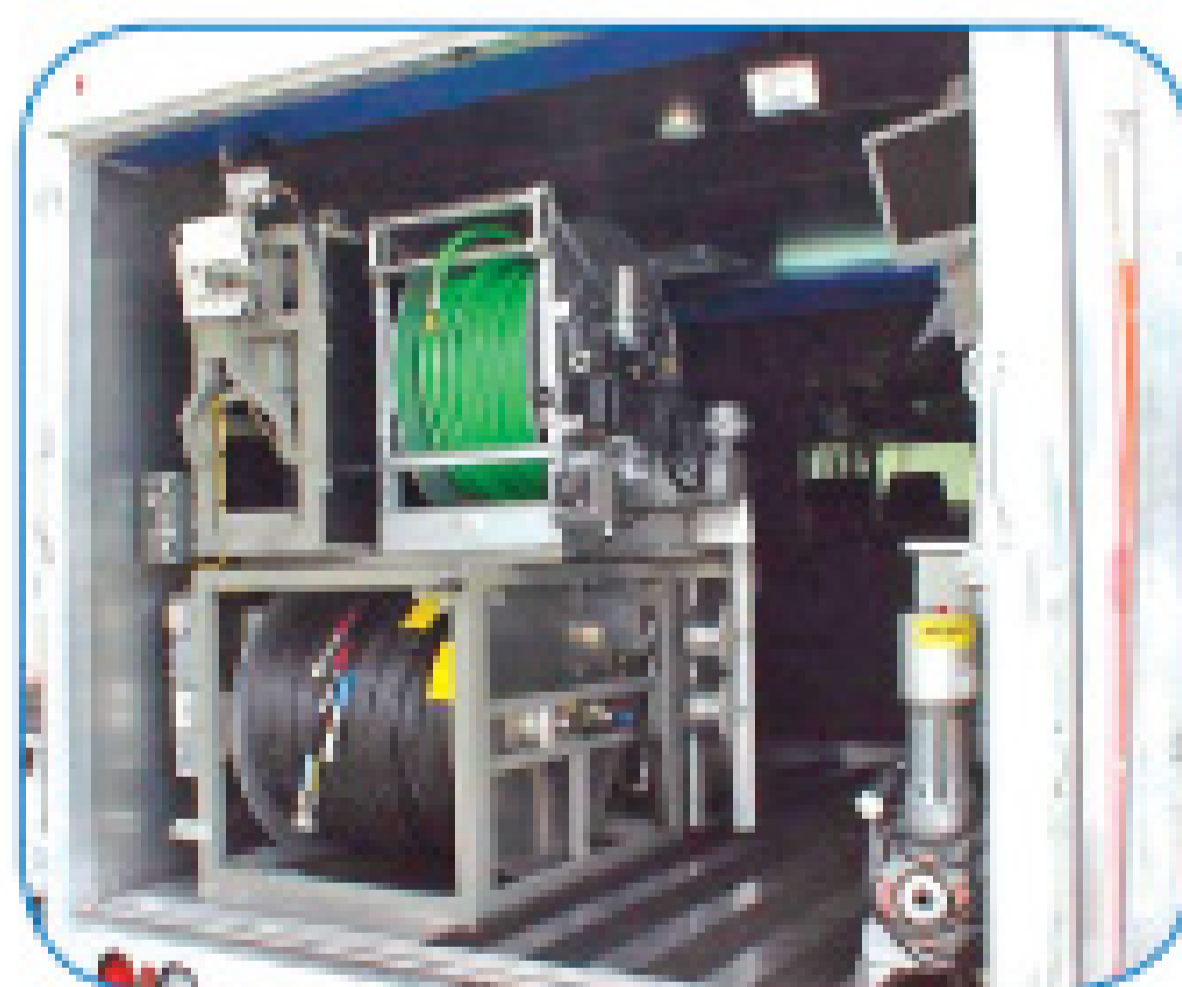
TV CUTTER GROUT
