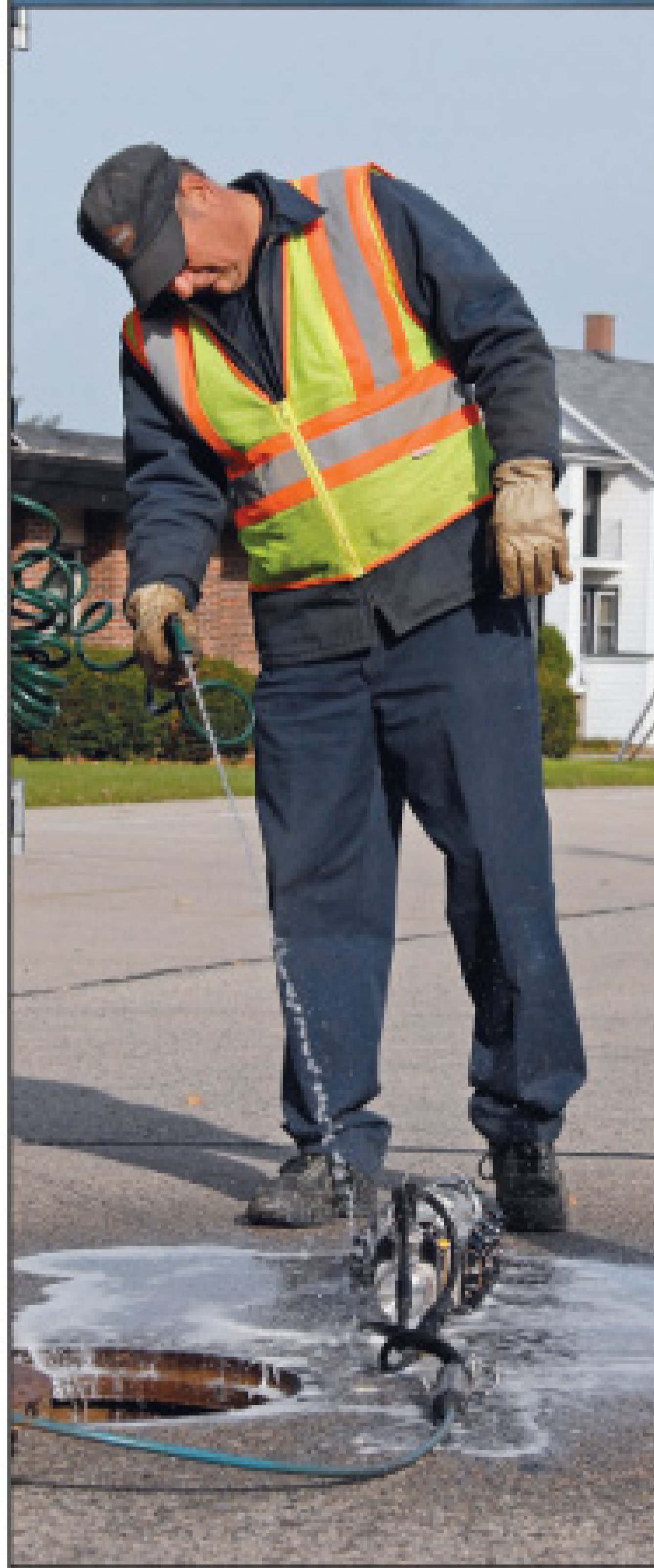
Gary Kmiecik sprays a disinfectant bleach solution on the UEMSI Prowler tracker with Cobra pan-and-tilt camera after an inspection.
