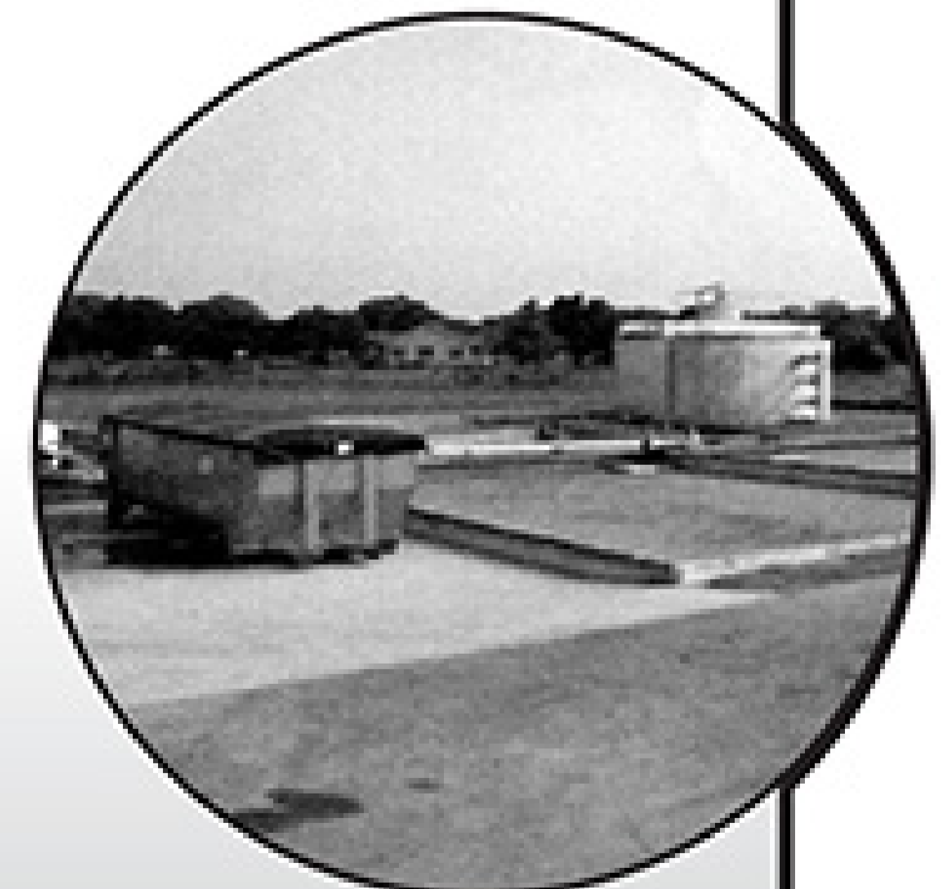
One of six drying beds converted to concrete to accommodate entire dewatering system.
