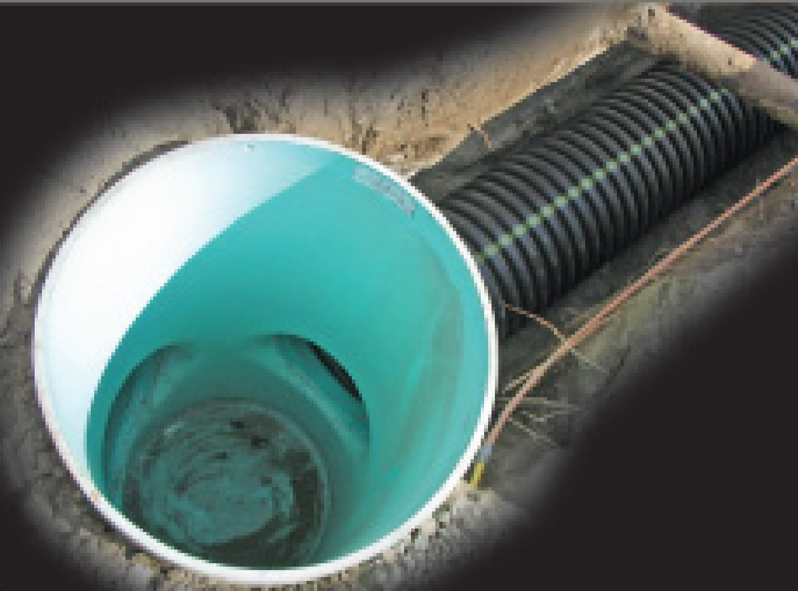
Nyloplast catch basin in place.
