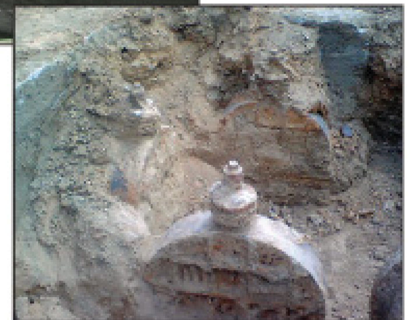
A very old and atypical valve found in the oldest section of Wilmington's system.
