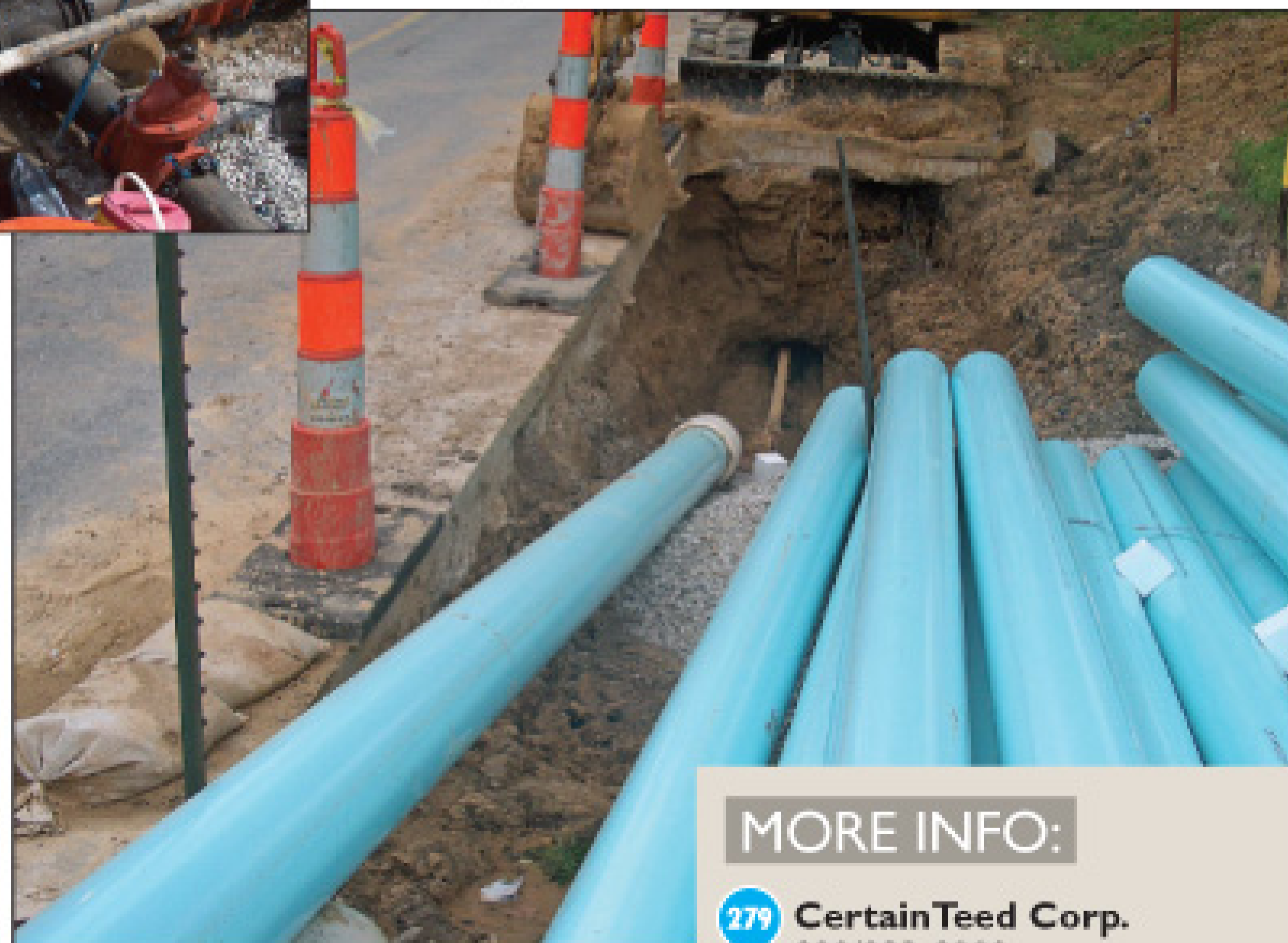
Left, a water main replacement project placed Certa-Lok C900/RJ pipe with a combination of Mueller gate valves on ductile iron. Below, pipe is stacked and ready to be pulled into the pit on a main replacement.
