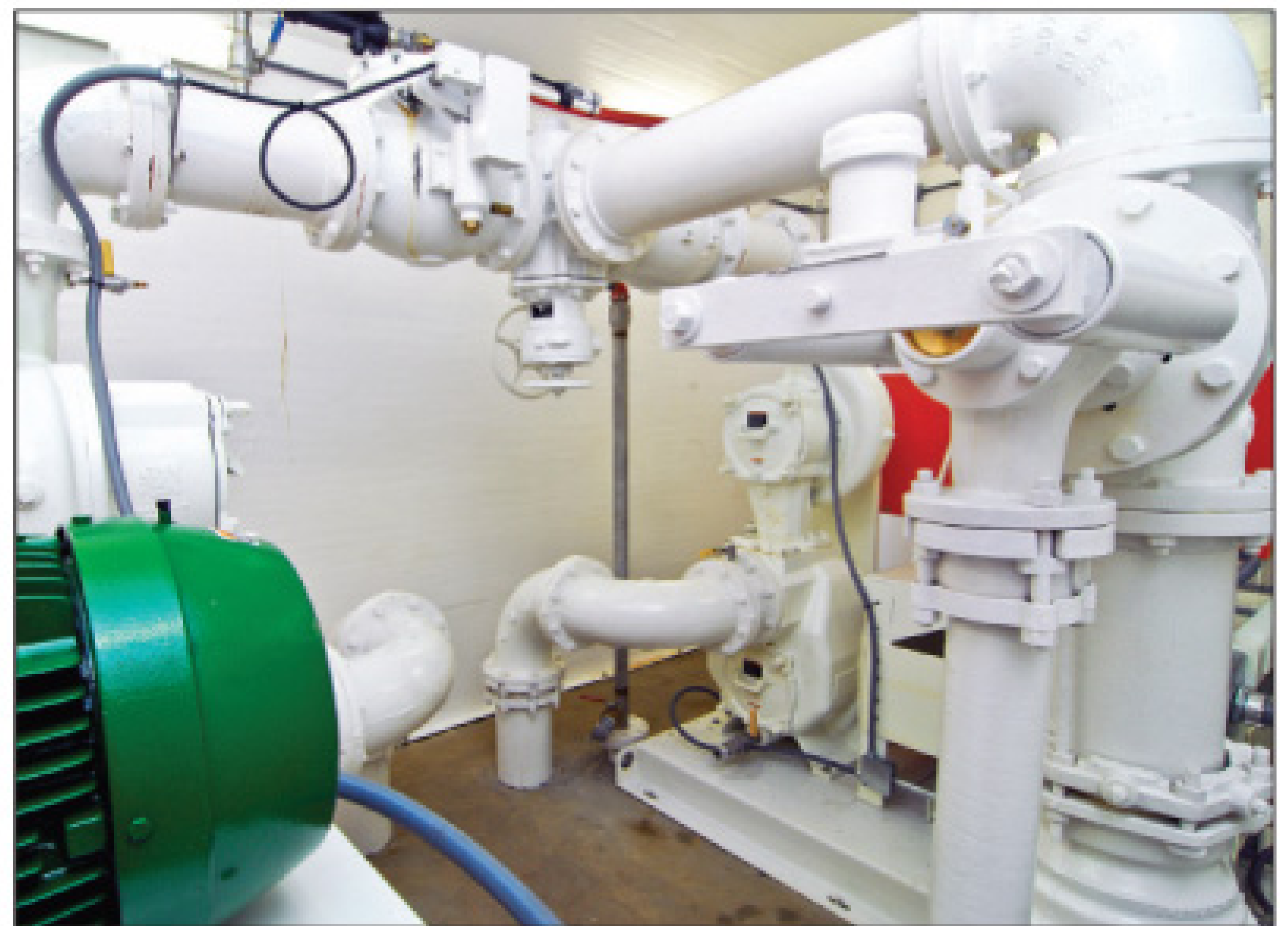
Above, a set of pumps showing the inspection covers on both Ultra V units. Left, a full view of a complete set of Ultra V pumps from the belt drive side.
