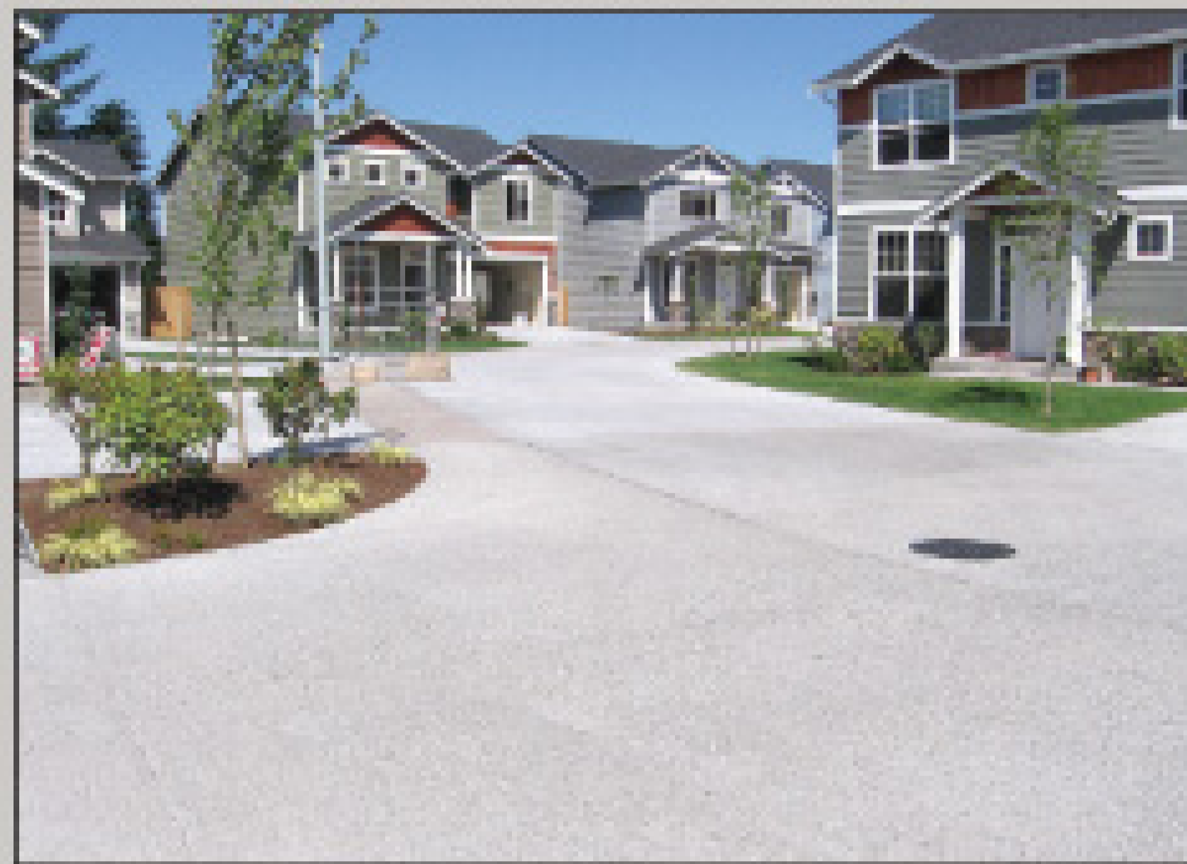
Pervious concrete streets and driveways on Stratford Place in Sultan, Wash.
