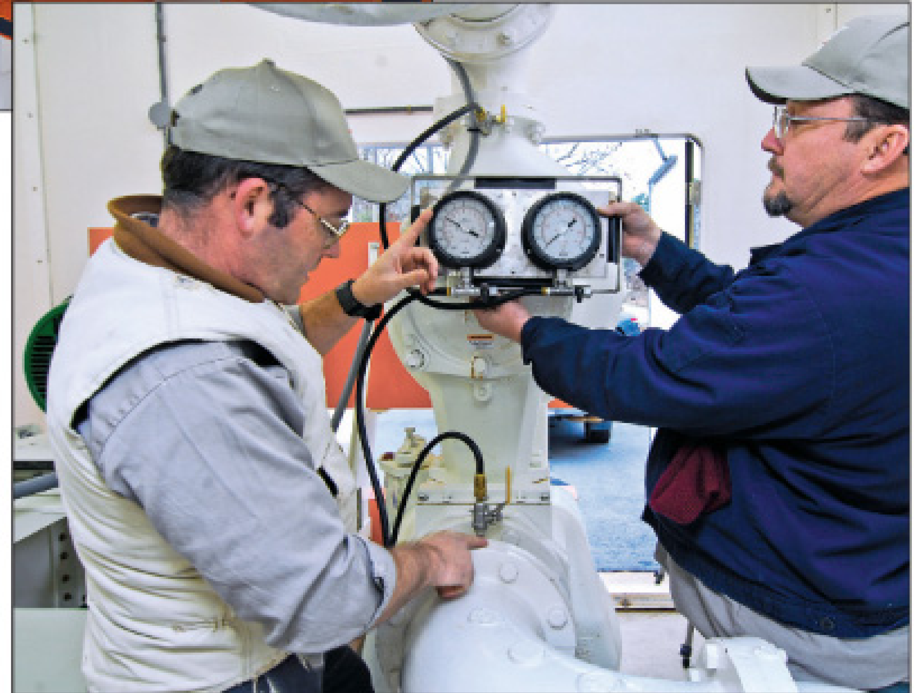
John Schafer (left) and Scott Tate take gauge readings with a mobile gauge set.
