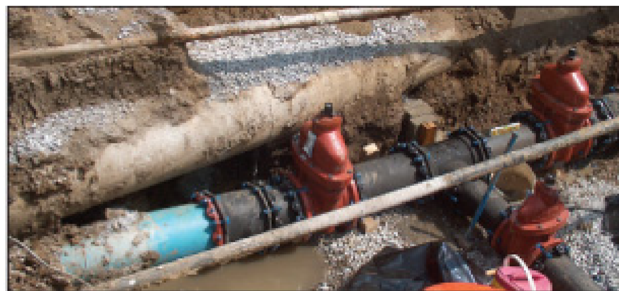
Left, a water main replacement project placed Certa-Lok C900/RJ pipe with a combination of Mueller gate valves on ductile iron. Below, pipe is stacked and ready to be pulled into the pit on a main replacement.
