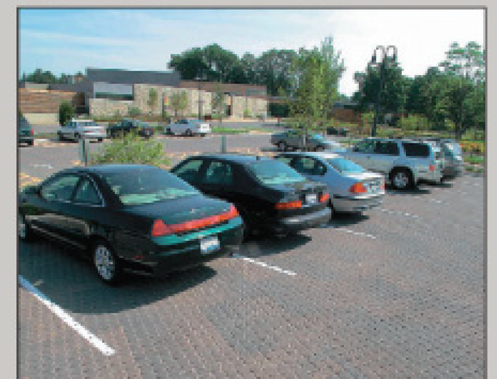
A permeable parking lot surface supports a "green" approach at Morton Arboretum.
