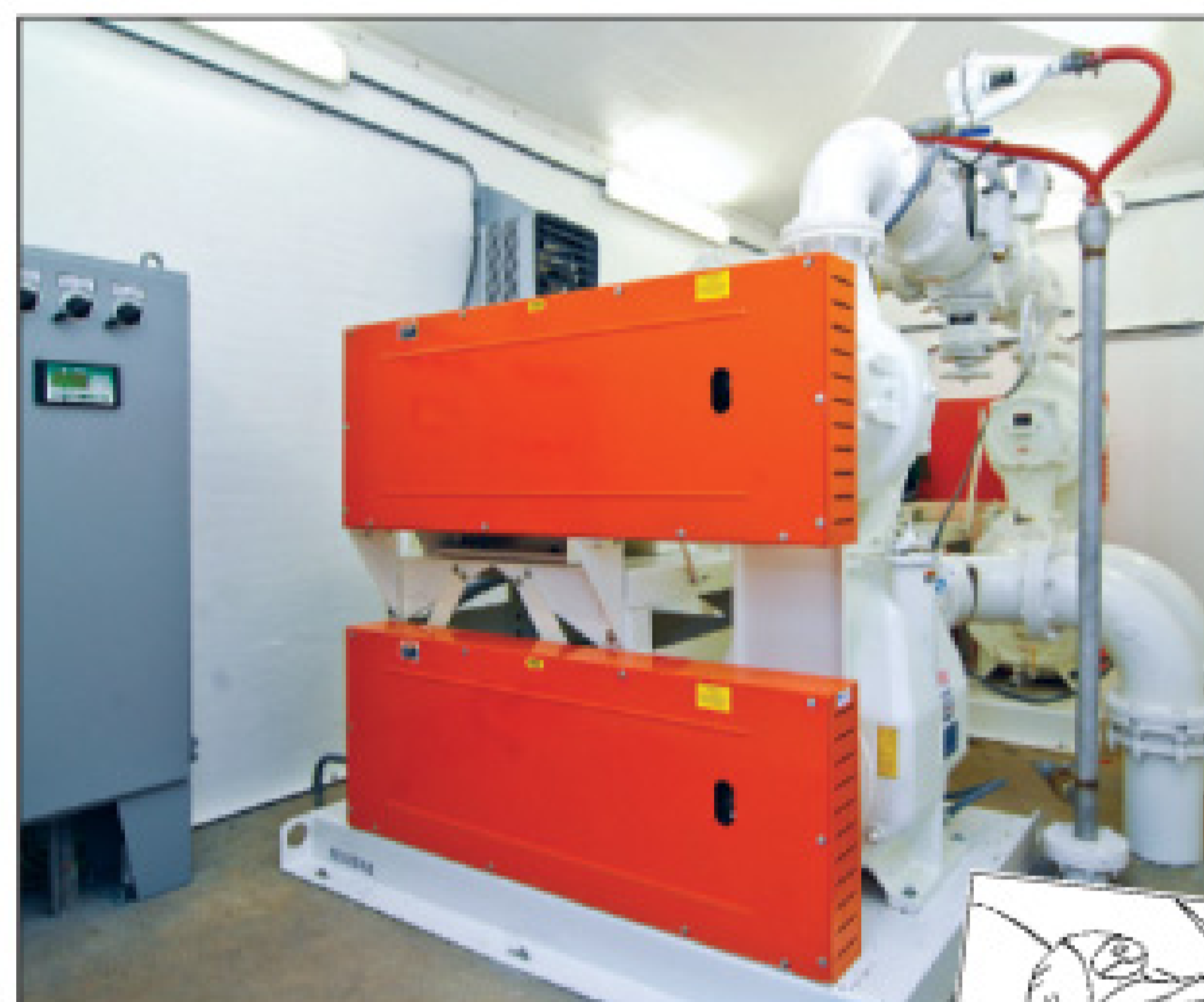
Above, a set of pumps showing the inspection covers on both Ultra V units. Left, a full view of a complete set of Ultra V pumps from the belt drive side.
