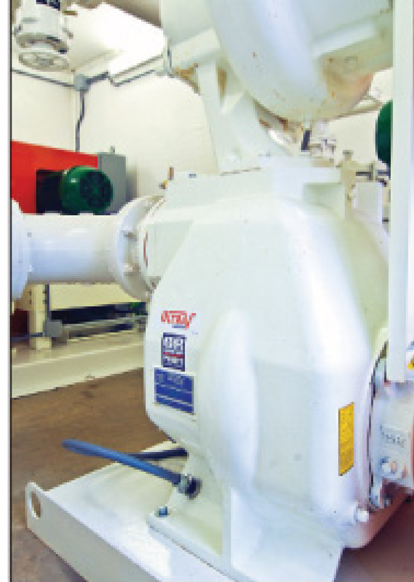
A Gorman Rupp Ultra V pump (first stage).
