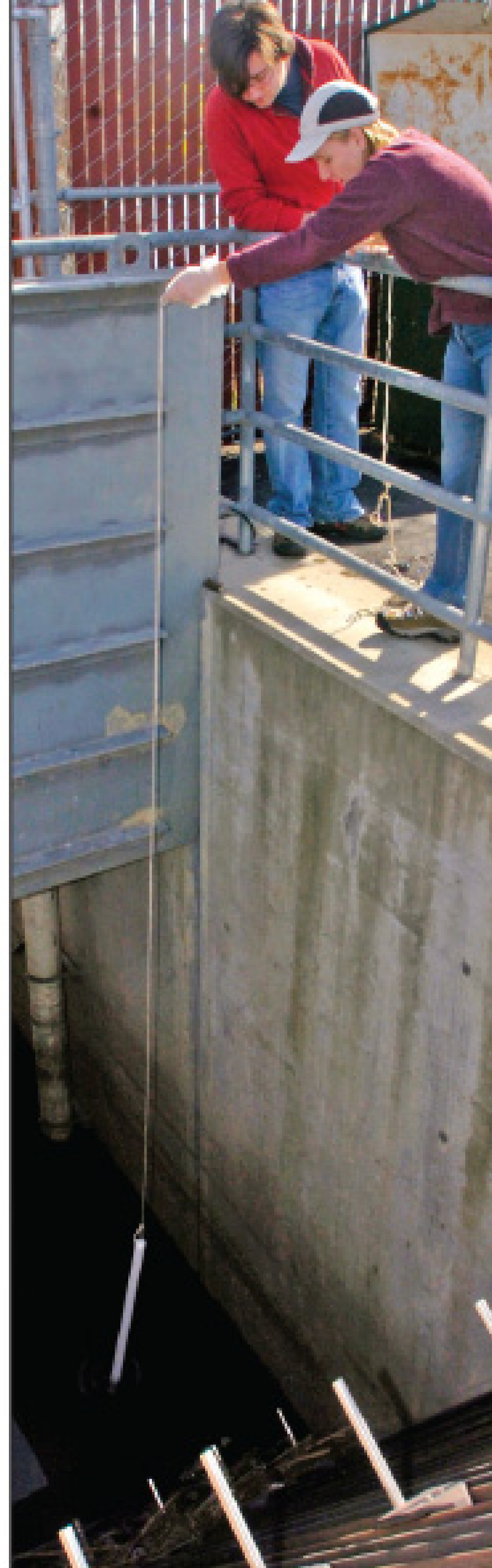
Damien Charley and Roxanne Dilley use a rope bailer to collect a water sample from a wet well at a pump station.
