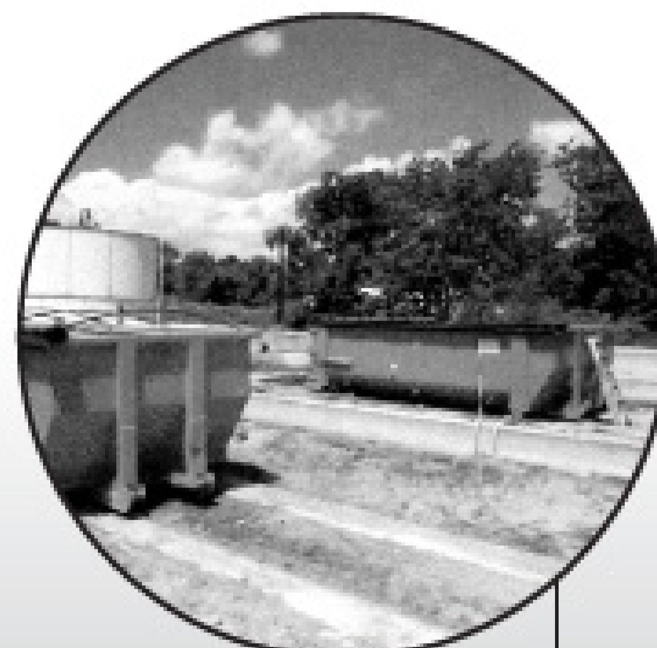
Concrete runners installed in existing drying beds for placement of roll-off dewatering box.
