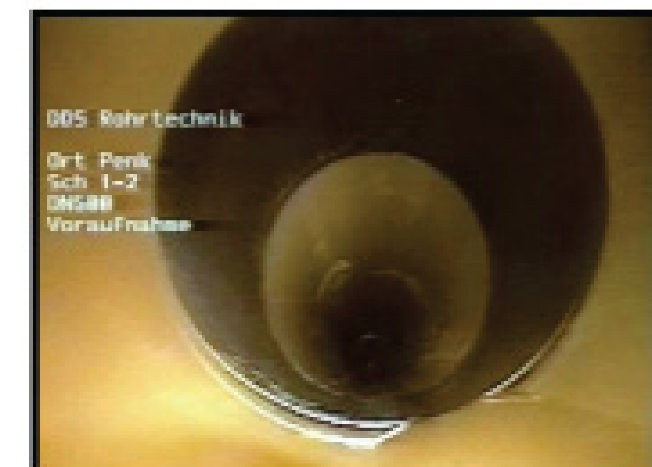
COMPLETE SEAL WITH QUICK LOCK GASKET INSTALLED
