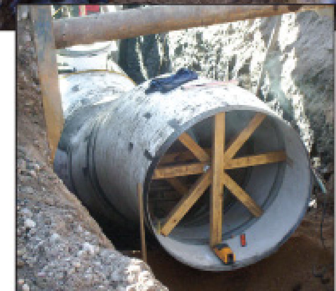
Wood stulls keep the cement-lined transmission pipe in shape until assembly.
