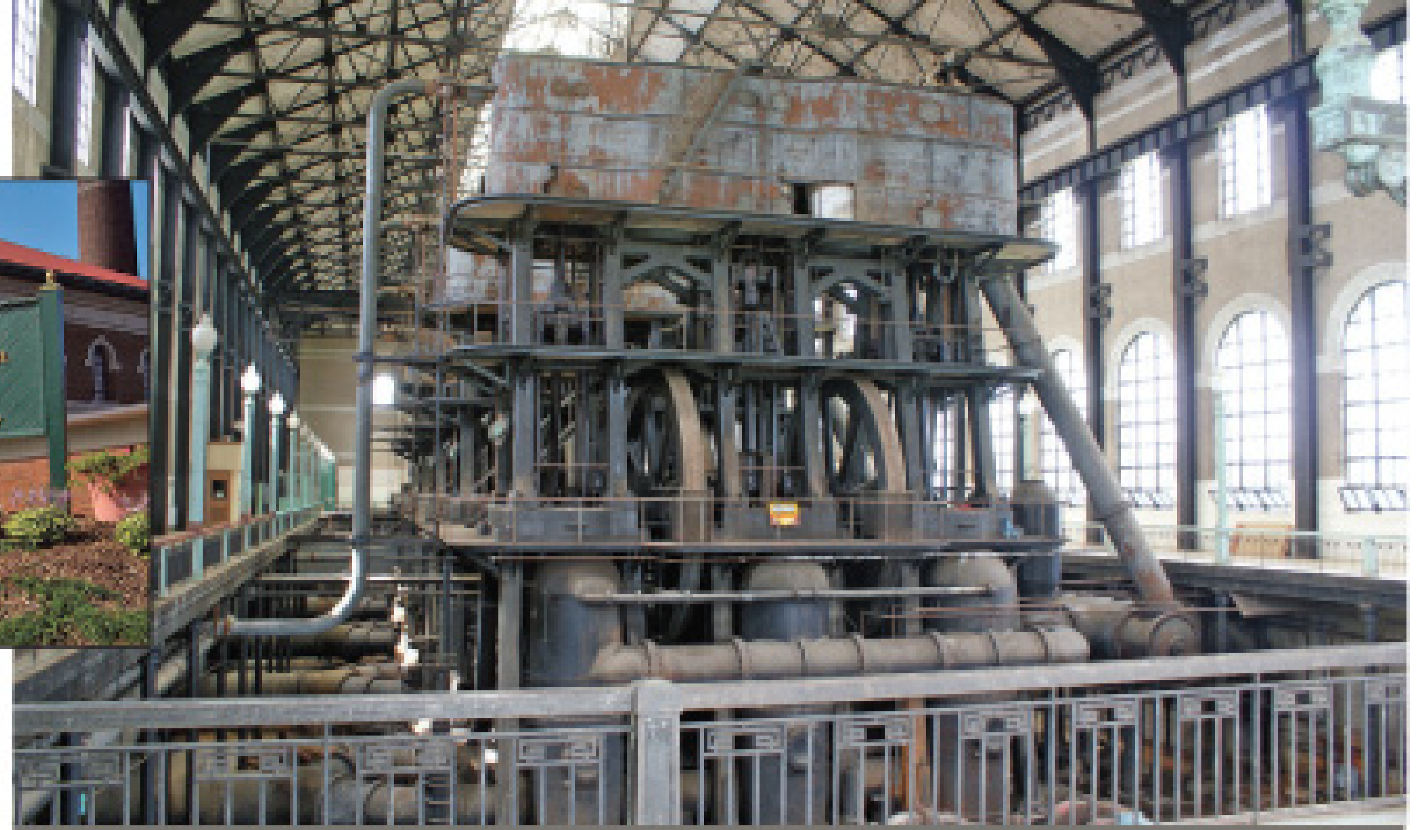
Buffalo's Ward Pumping Station (above) houses five original steam pumps (right photo) installed almost a century ago. Each pump is four stories tall and weighs more than 1,000 tons. They are no longer in use.
