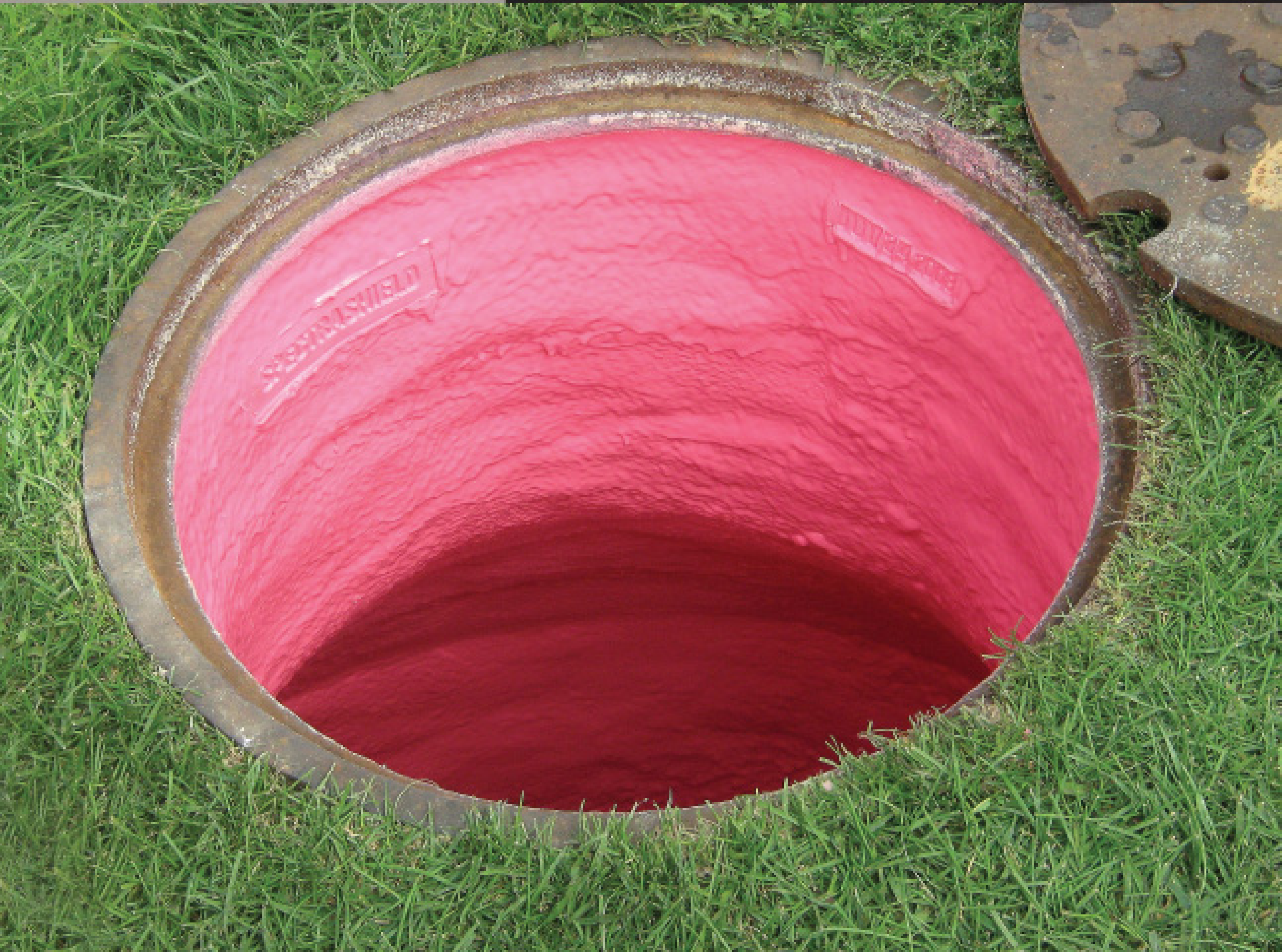
The manhole after application of the final corrosion barrier.
