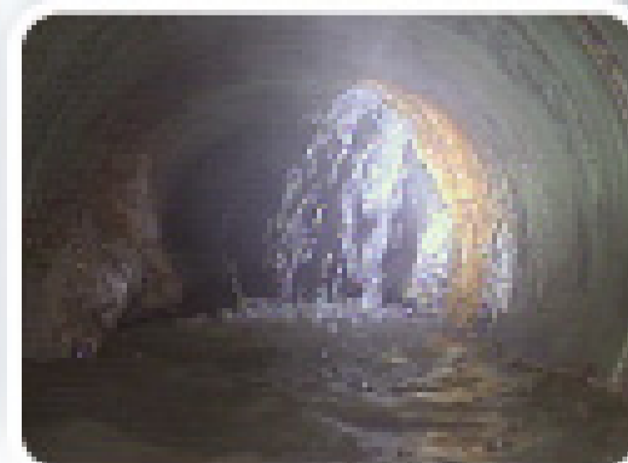
Gushing Infiltration
