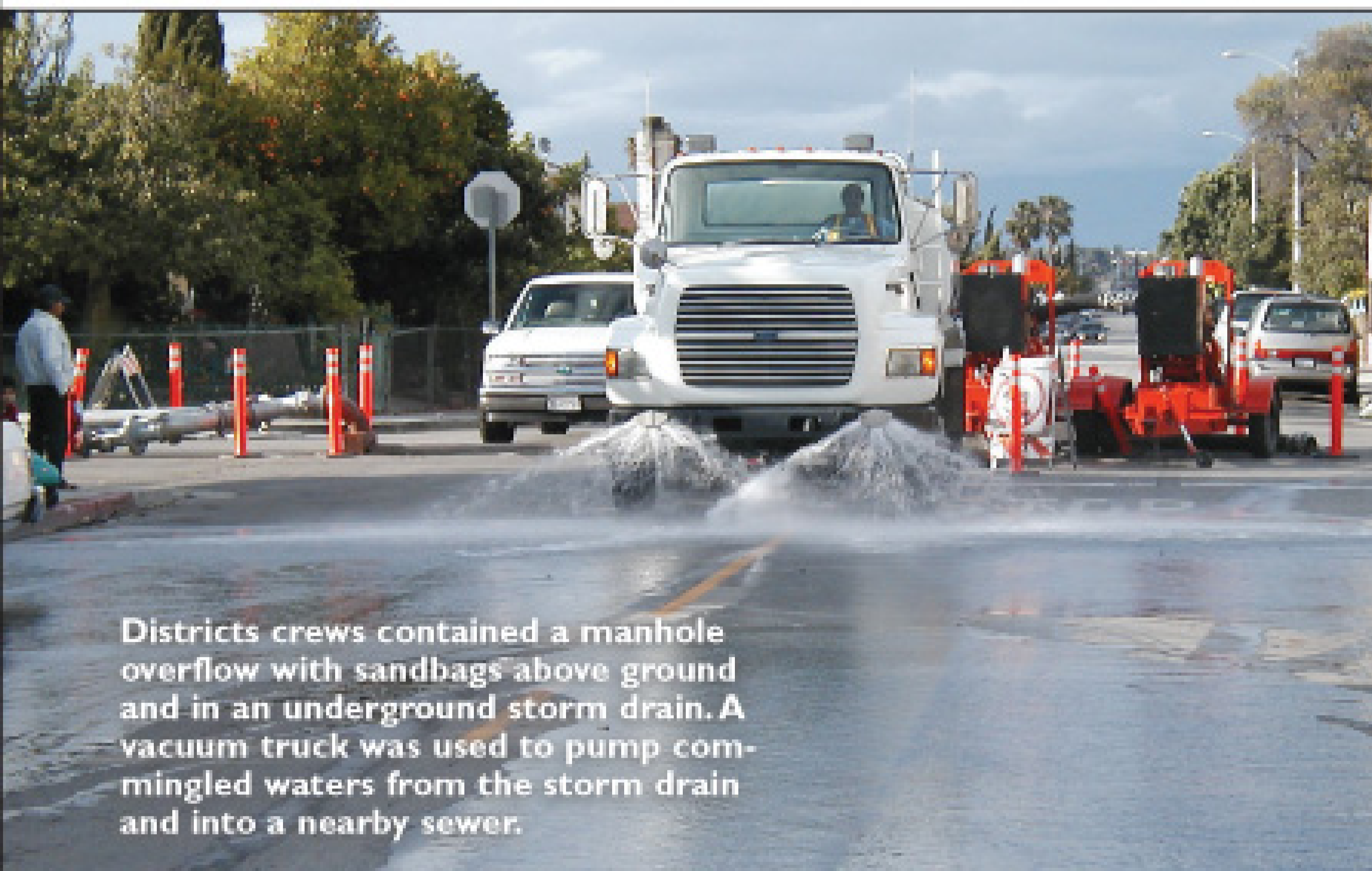
In an overflow situation in the City of Glendora, Sanitation Districts crews set up a pumping system to bypass the majority of the flow. A second bypass was placed into service to bypass remaining flow. Crews drained the excavation using two vacuum trucks and cleaned debris from the manhole and sewer pipe to clear the blockage.
