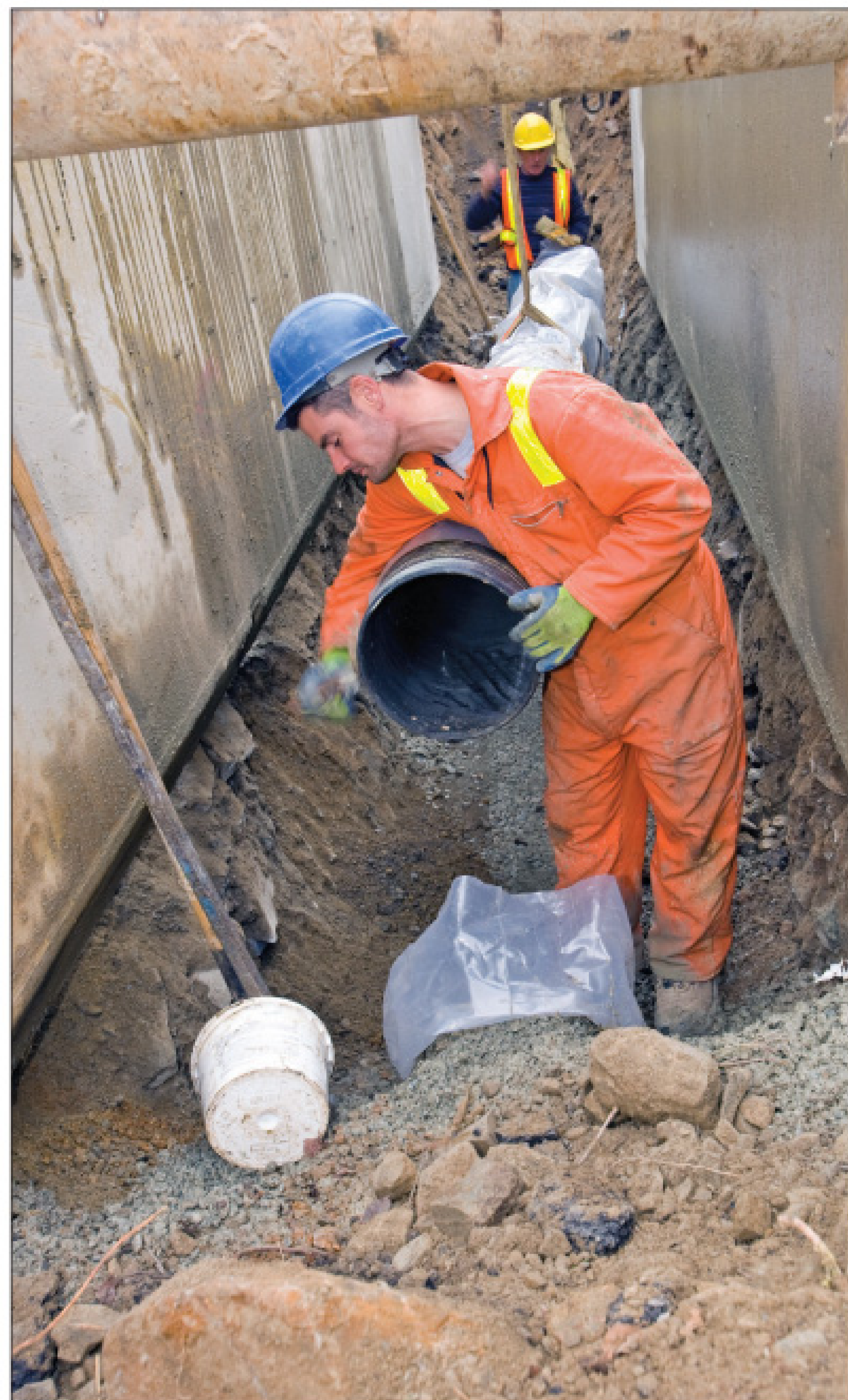
Taylor Cook applies grease to help join two pipe sections.
