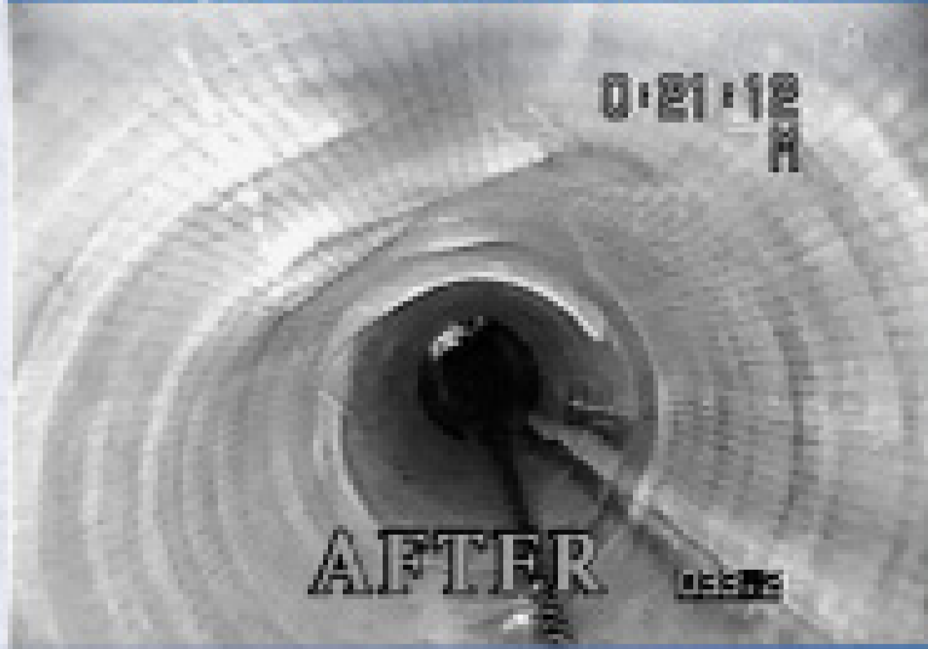
Missing piece of host pipe repaired.
