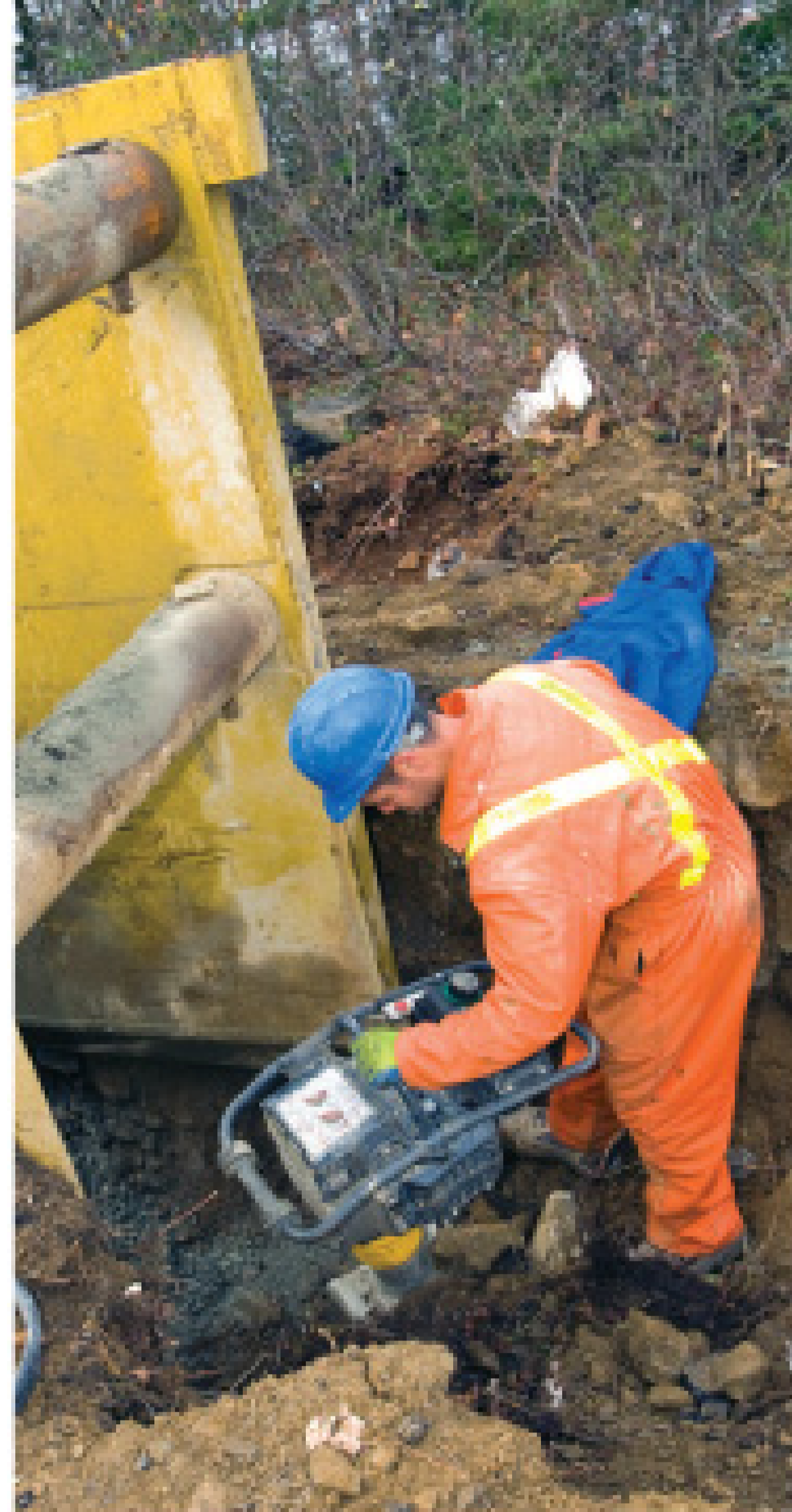
Taylor Cook works with a soil compactor on a pipe installation.
