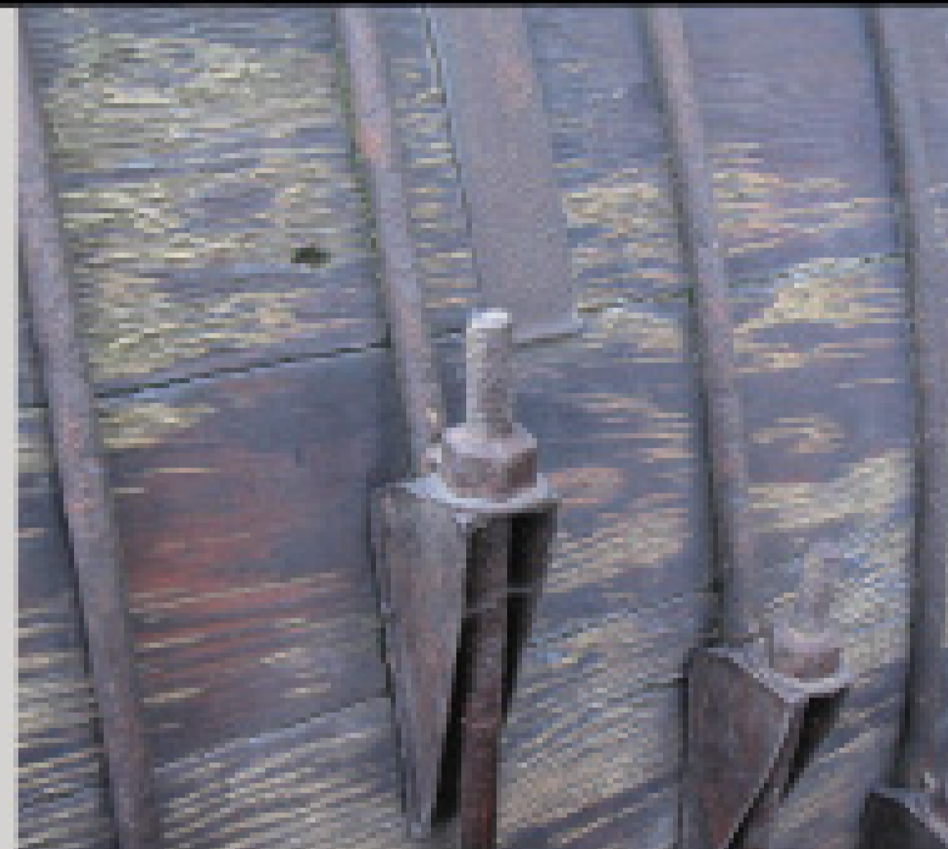
Old wooden pipes are a unique feature of the King County sewer system.
