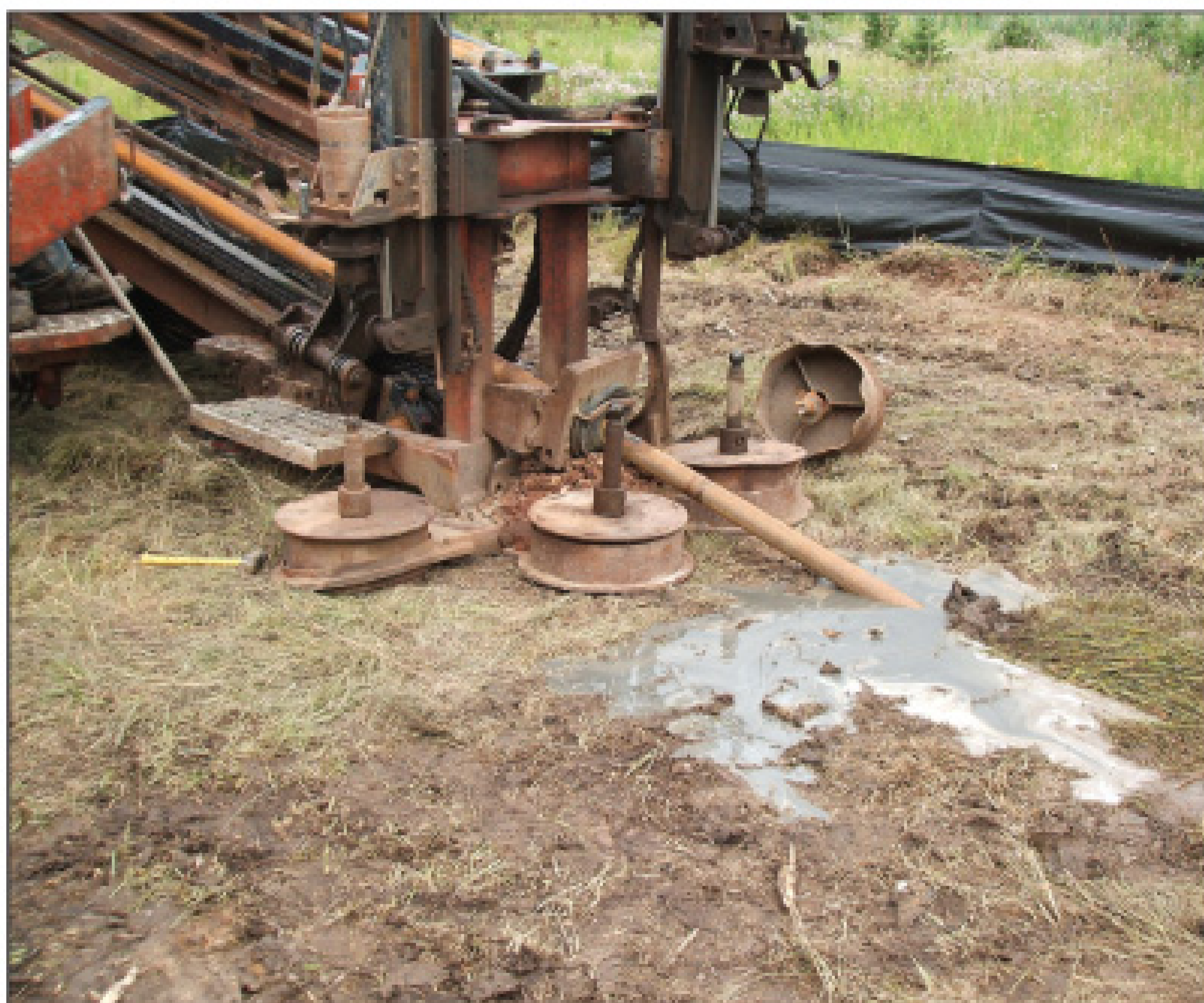
The drill head penetrates the ground at a low angle.
