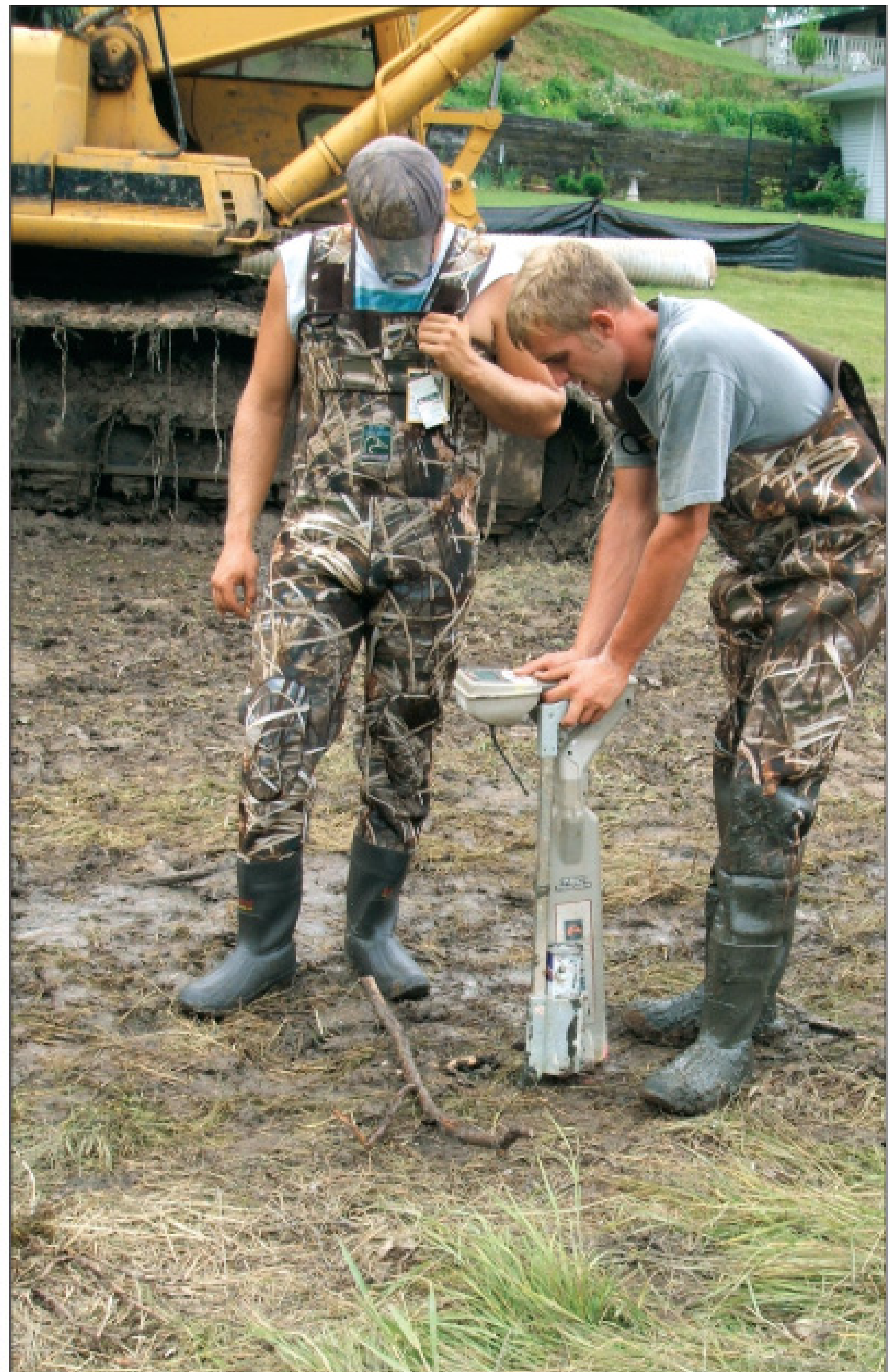
Above: The view west across the marshy area under which the boring is to be done. The bore will be completed from the opposite side. Right: Ramco employees Micah Frost (left) and Glen VandeHey track the drill head. VandeHey uses a Subsite 750 Tracker from Ditch Witch to follow a sonde in the drill head.
