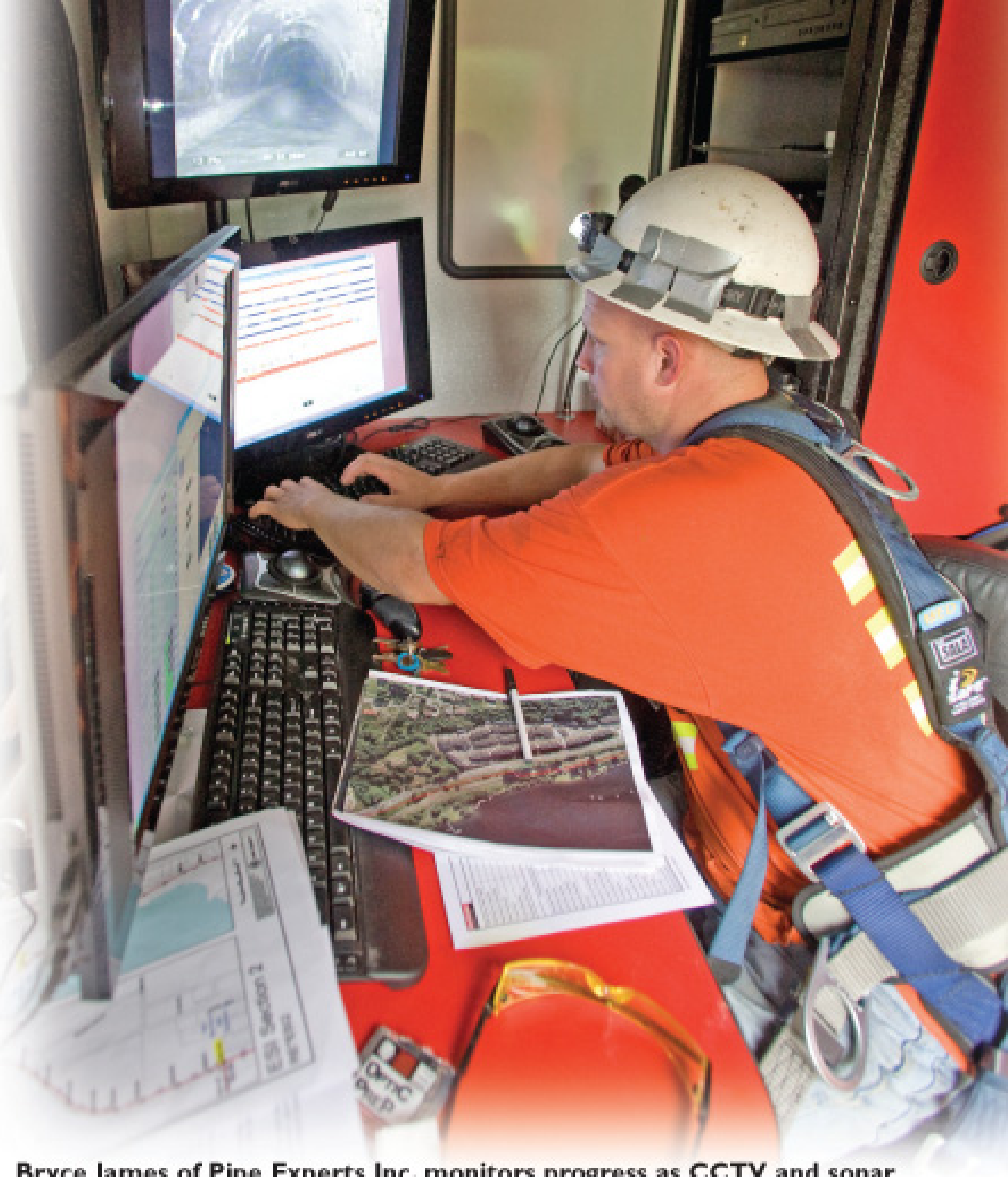
Bryce James of Pipe Experts Inc. monitors progress as CCTV and sonar check out a 96-inch interceptor in King County, Wash. (Photography by Ned Ahrens, King County)
