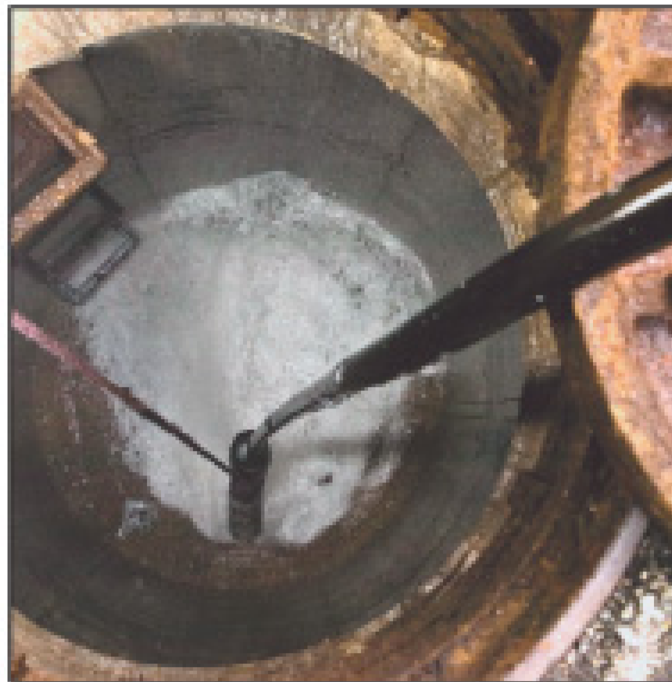
Top left: A map generated by Geomedia GIS software in the city TV truck shows a neighborhood in which a crew is doing root control work. Bottom left: A foaming pipeline root control formulation kills roots in the City of Fairfield's sewers. Right: Assistant foreman Jason Turner controls a remote camera as he views live video of sewer lines from the TV truck.
