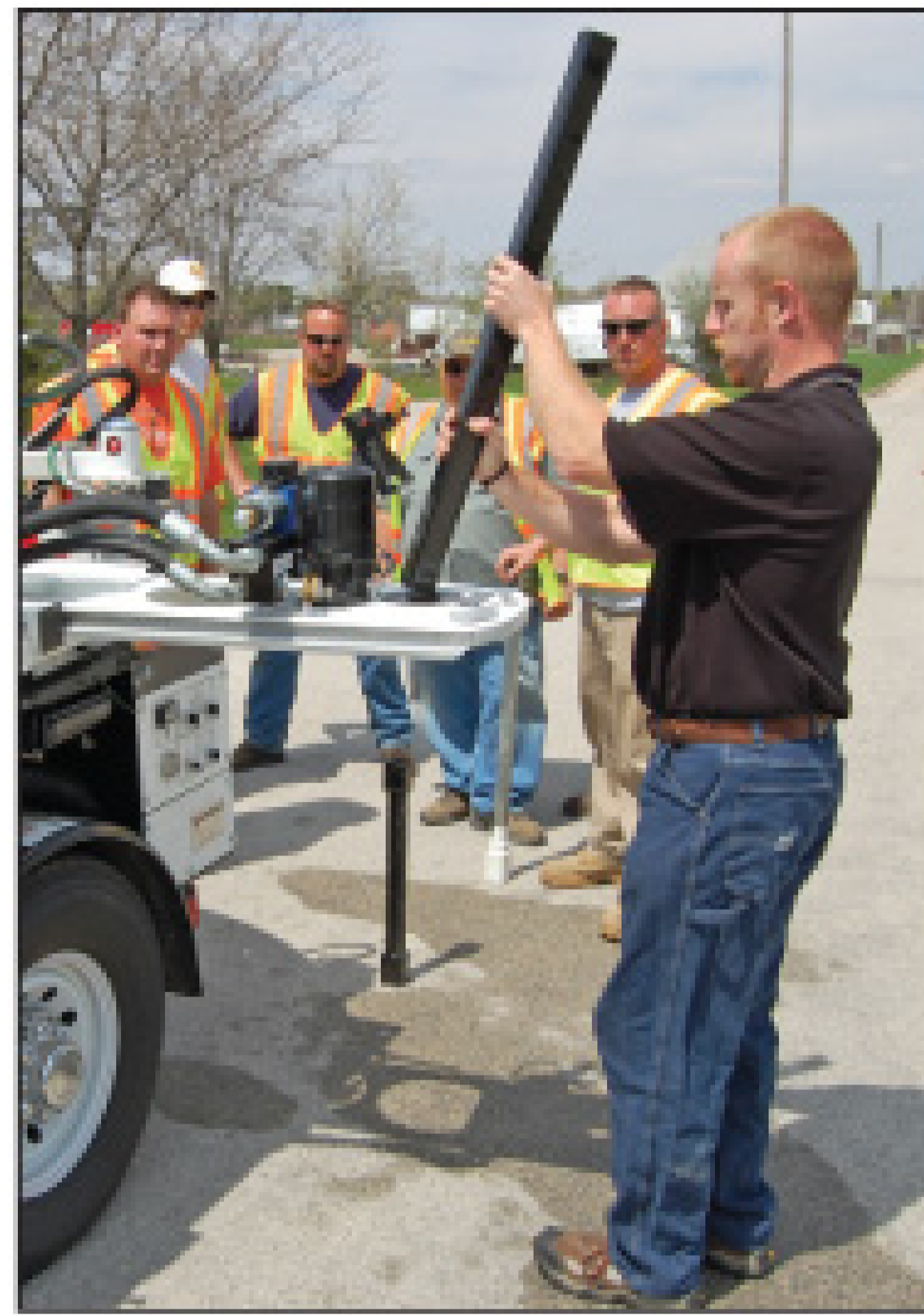
Bertrand places a valve key into the TM-7 exerciser, which delivers up to 1,500 foot-pounds of torque for turning large or stubborn valves.
