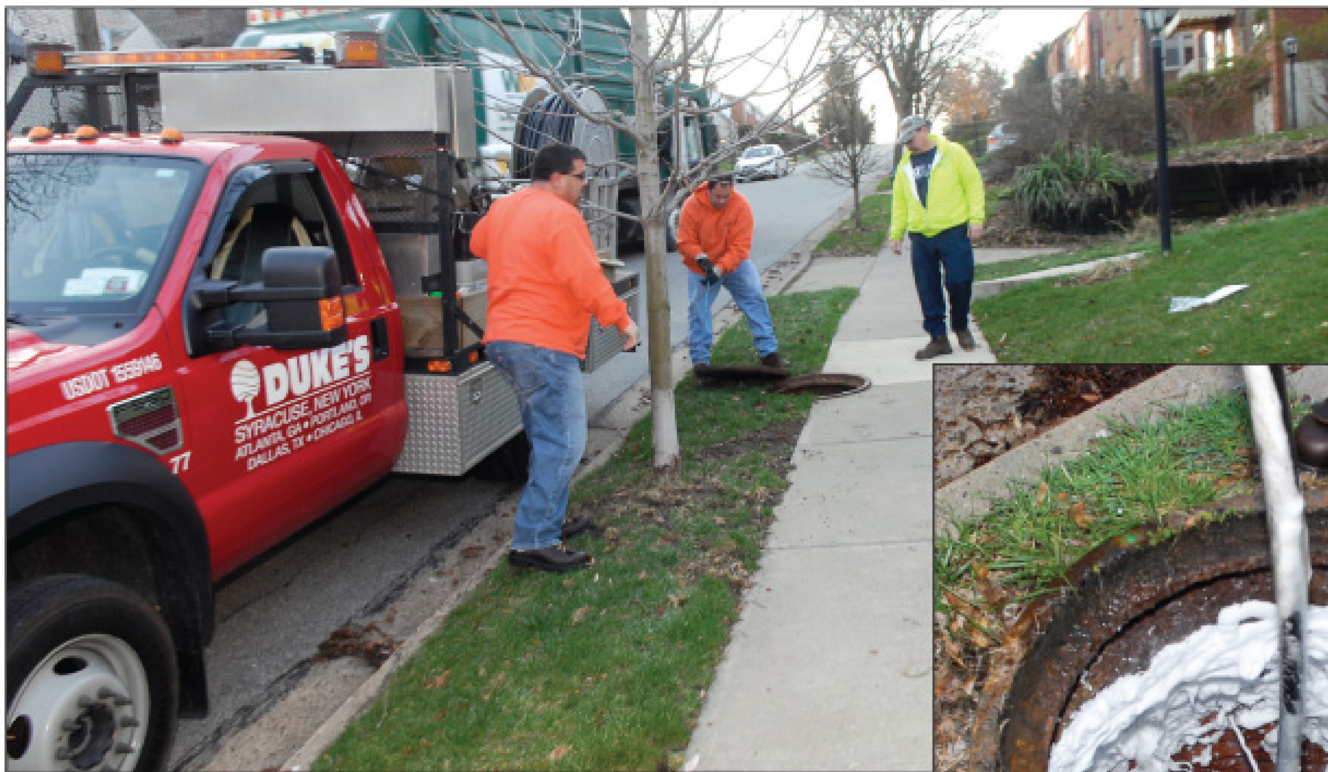
Left photo: Dave Wall (left) and Josh Amo of Duke's Root Control prepare for a root treatment in a Mt. Lebanon sewer, as public works staff member Rick Virgi observes. Lower photo: A mixture of diquat and corn foam is applied to kill roots and prevent growth.
