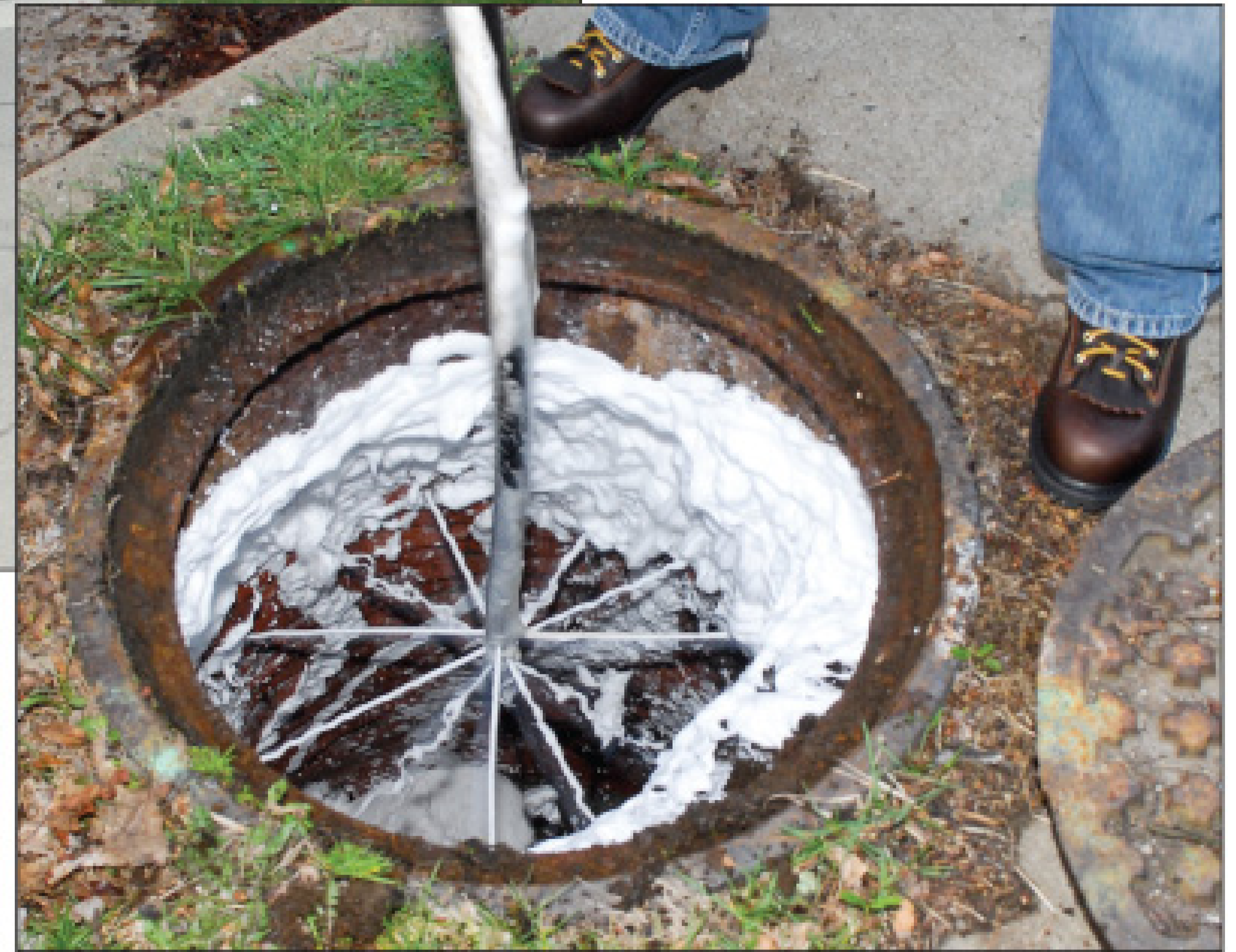
Left photo: Dave Wall (left) and Josh Amo of Duke's Root Control prepare for a root treatment in a Mt. Lebanon sewer, as public works staff member Rick Virgi observes. Lower photo: A mixture of diquat and corn foam is applied to kill roots and prevent growth.
