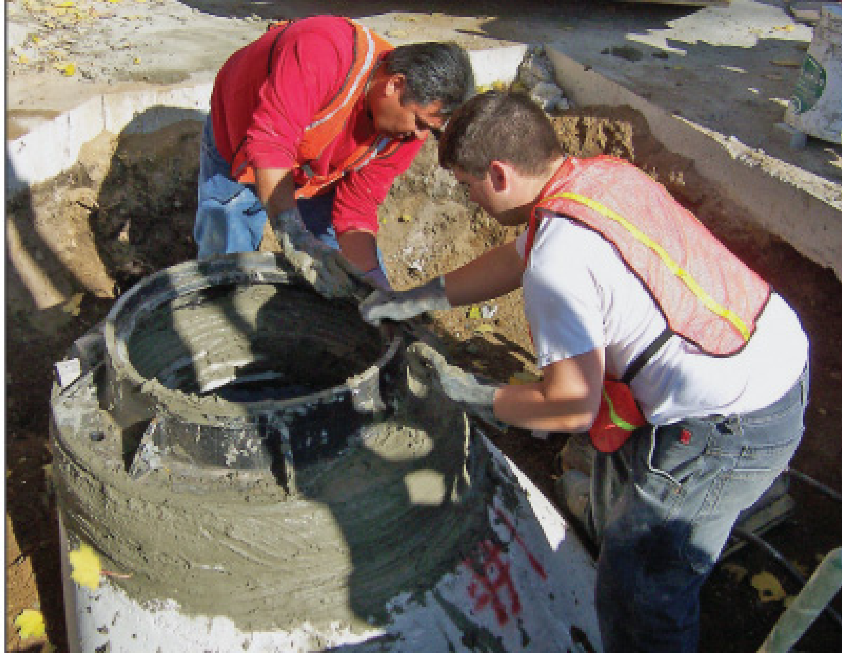
Above, Corunna's manhole rehabilitation project involved various sealing, grouting and rebuilding methods. At right, the city's sewer rehabilitation program included cured-in-place lining for mains. Insituform Technologies cleaned and inspected 30,967 feet of 6- to 18-inch mains before installing the CIPP liner.
