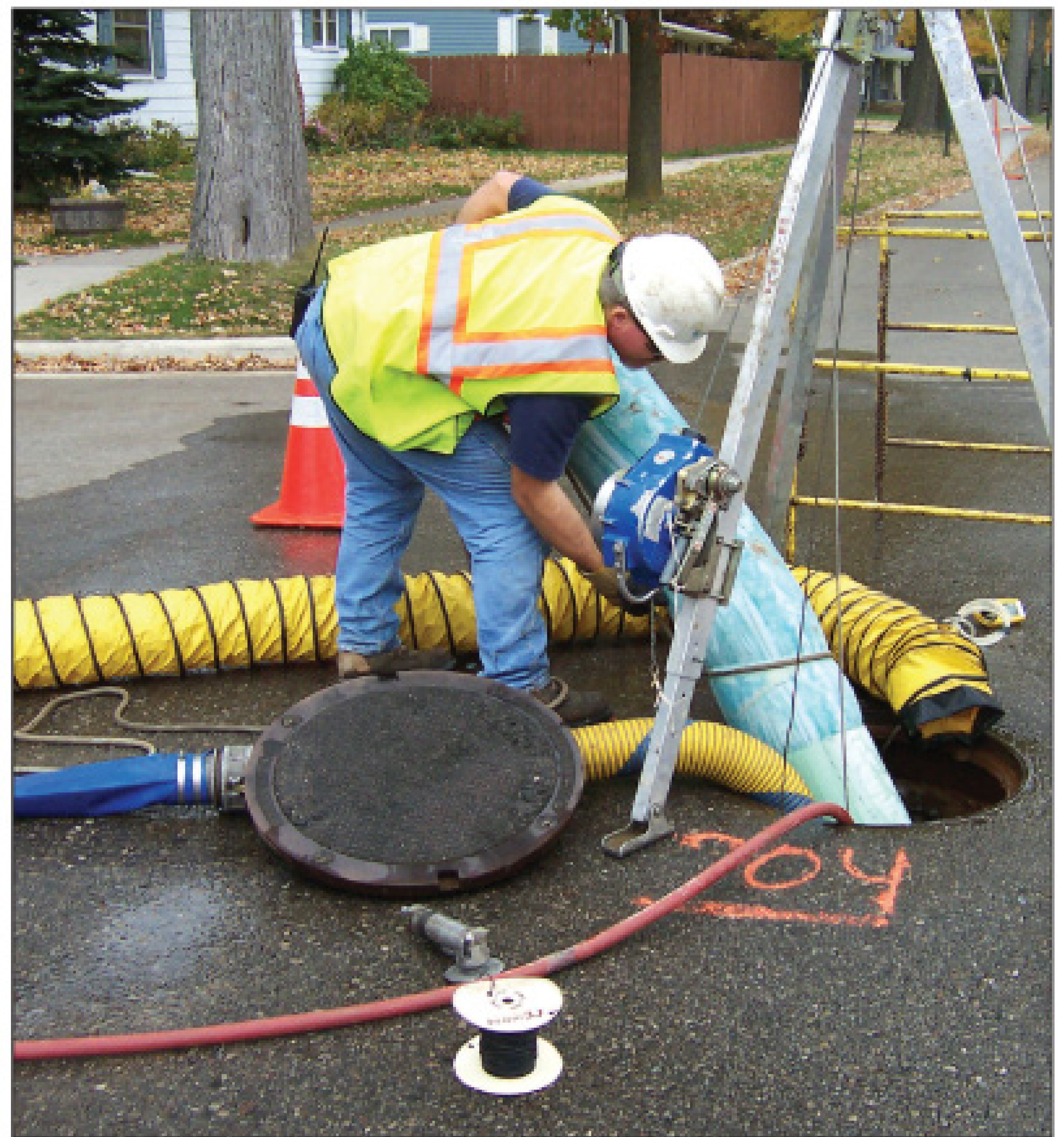
Above, Corunna's manhole rehabilitation project involved various sealing, grouting and rebuilding methods. At right, the city's sewer rehabilitation program included cured-in-place lining for mains. Insituform Technologies cleaned and inspected 30,967 feet of 6- to 18-inch mains before installing the CIPP liner.
