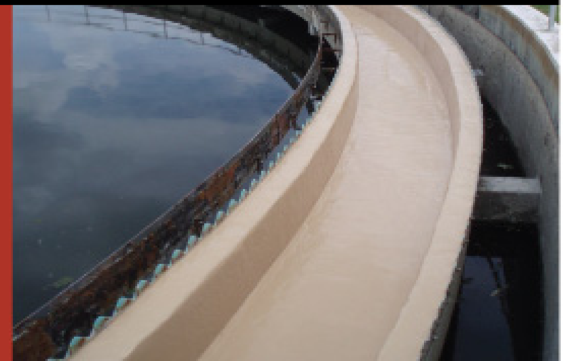
"Over 2-million square feet coated with Miami-Dade Water & Sewer"
