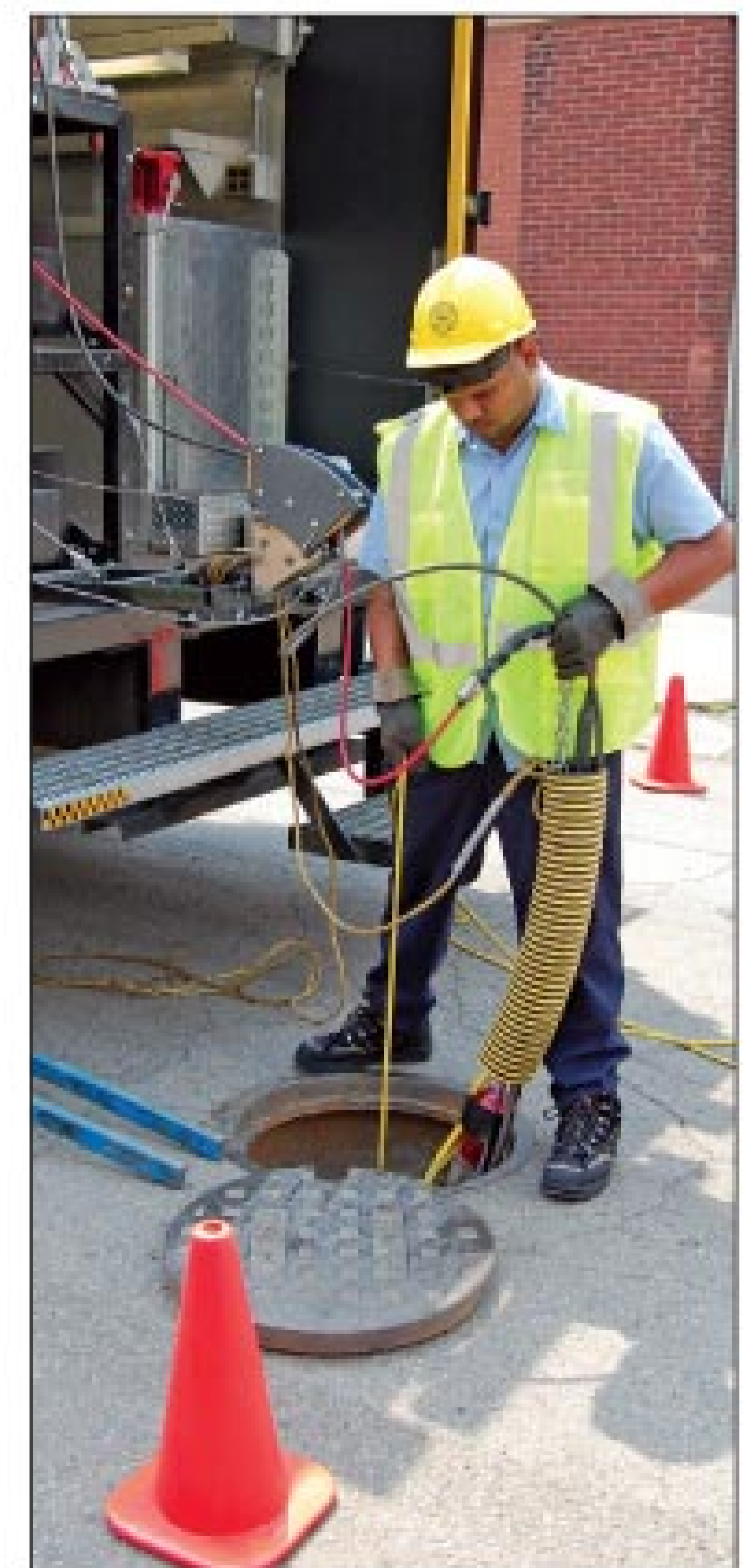
The system is deployed in the same manner as a traditional crawler camera. The crawler is connected to multi-conductor cable (red) and pushrod (black).
