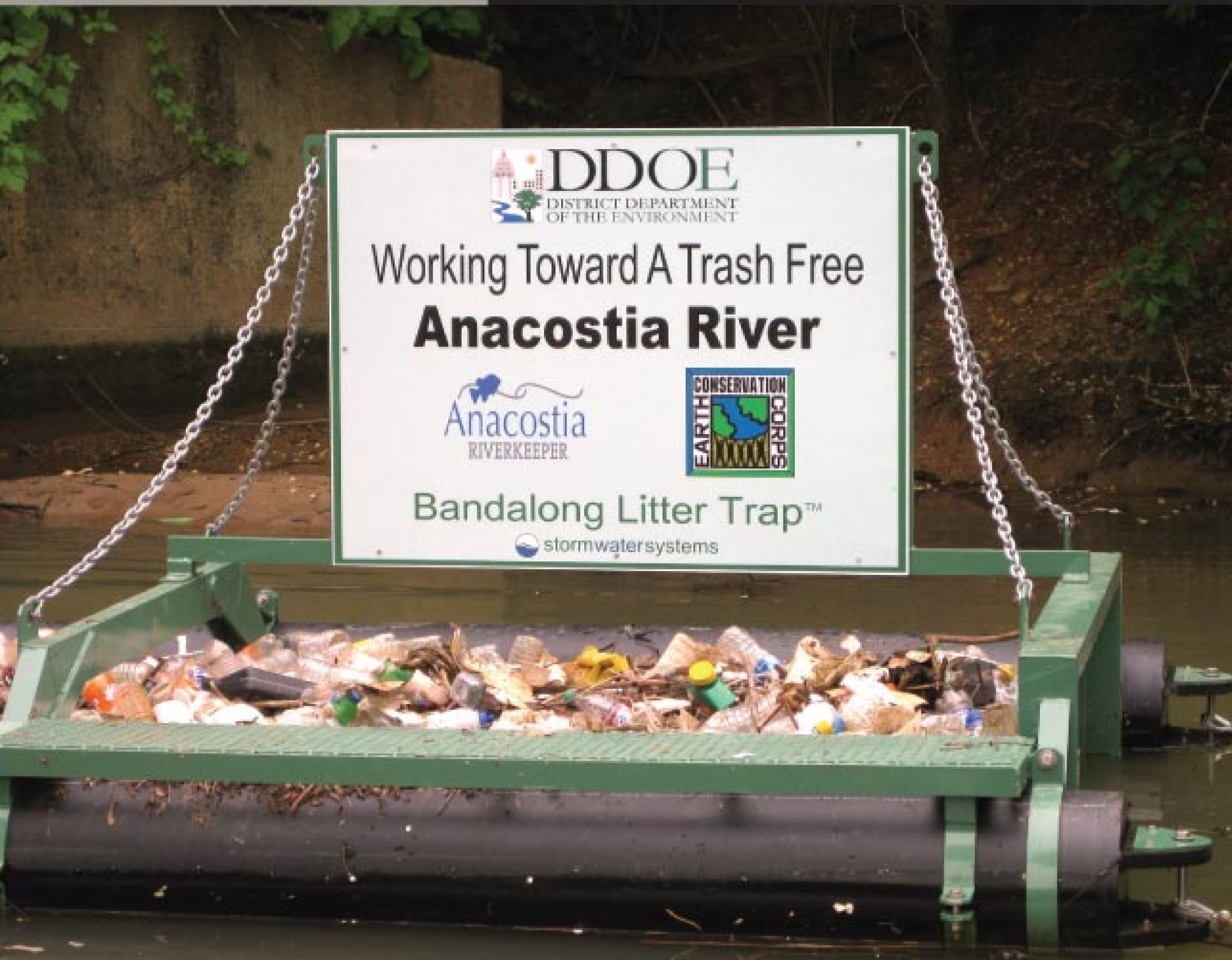
In the Bandalong Litter Trap, debris is corralled by flotation booms, while a gate prevents the litter from escaping. (Photos courtesy of Storm Water Systems Inc., Cleveland, Ga.)
