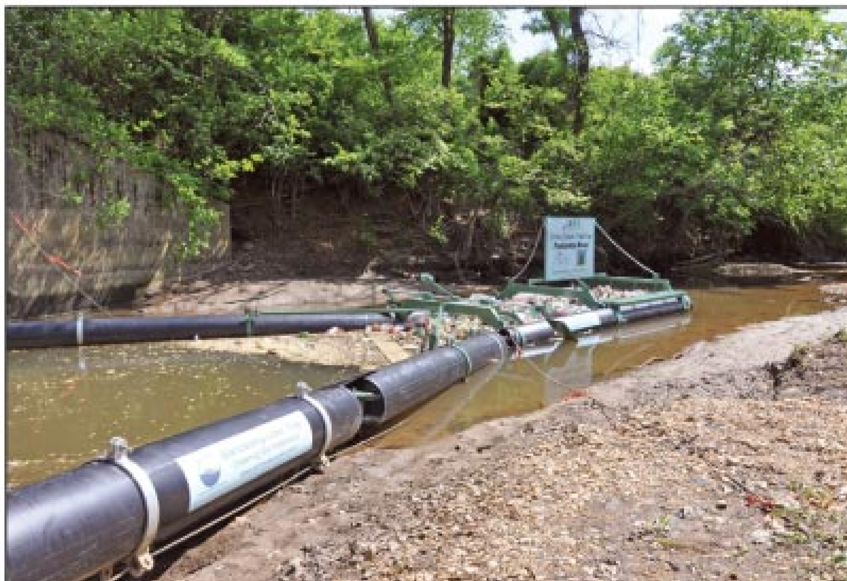
The litter trap fits in the lower tidal reach of Watts Branch in the deepest and widest part (40 feet) of the channel.
