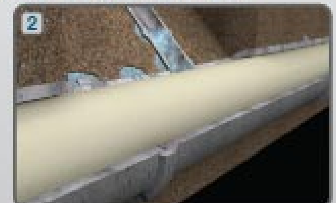
Liner installed
