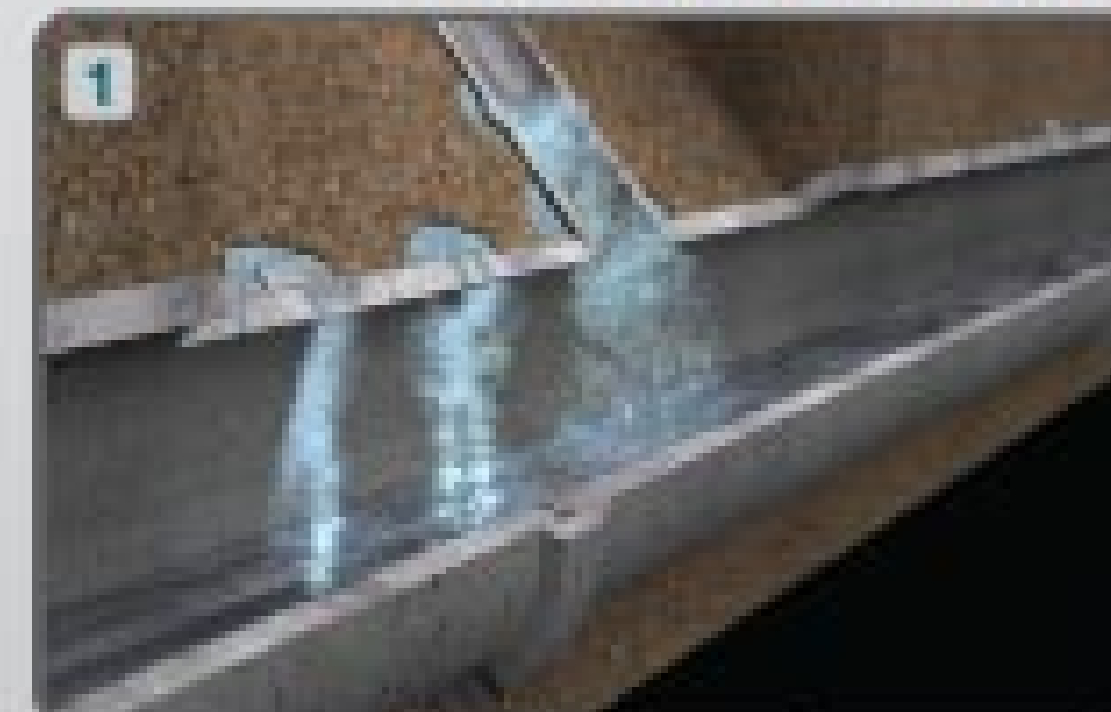
Leaking lateral
