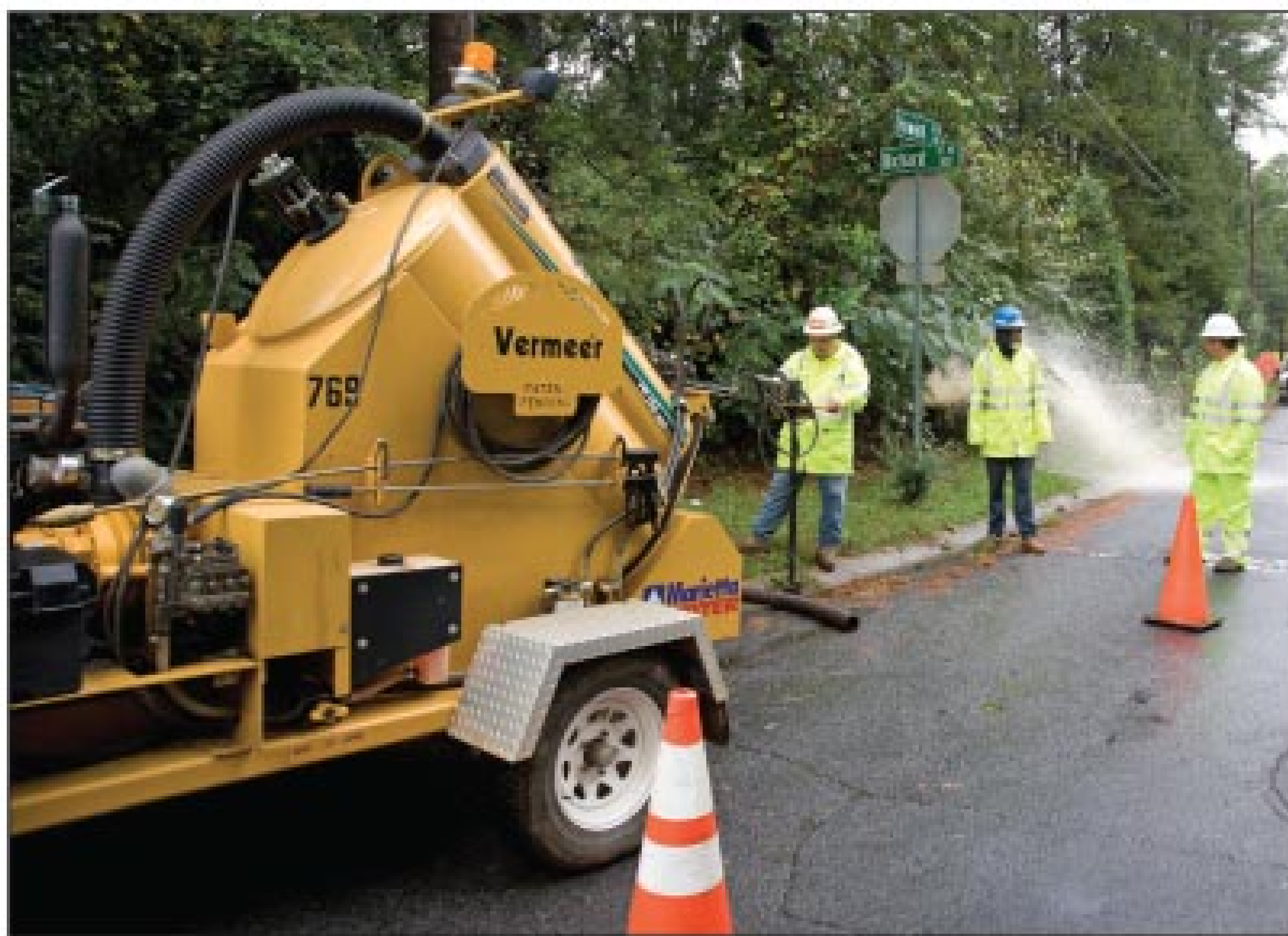
Maintenance and repair foreman David Sharp; system operator 2 Danny Ferrell; and distribution supervisor Troy Huebner use Vermeer equipment to perform valve exercising and hydrant flushing.
