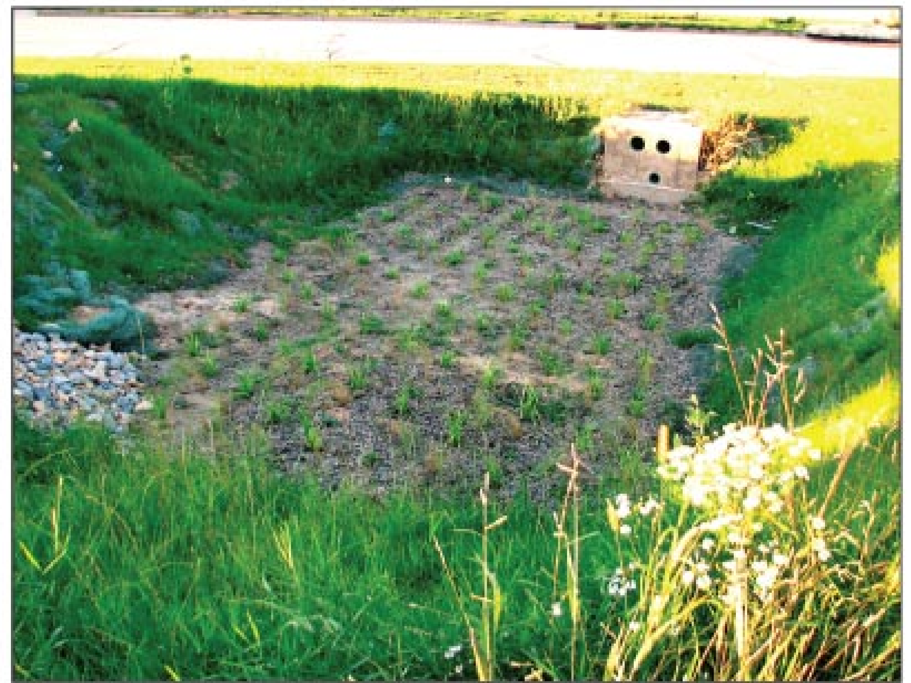
Bioretention basins are 10- to 12-foot-deep excavations filled with sand and topped with 3 feet each of clear stone and engineered soil, and a mix of compost, sand, and a little topsoil. The county plants native prairie vegetation in the basins because their deep roots retain more runoff than turf grass would.
