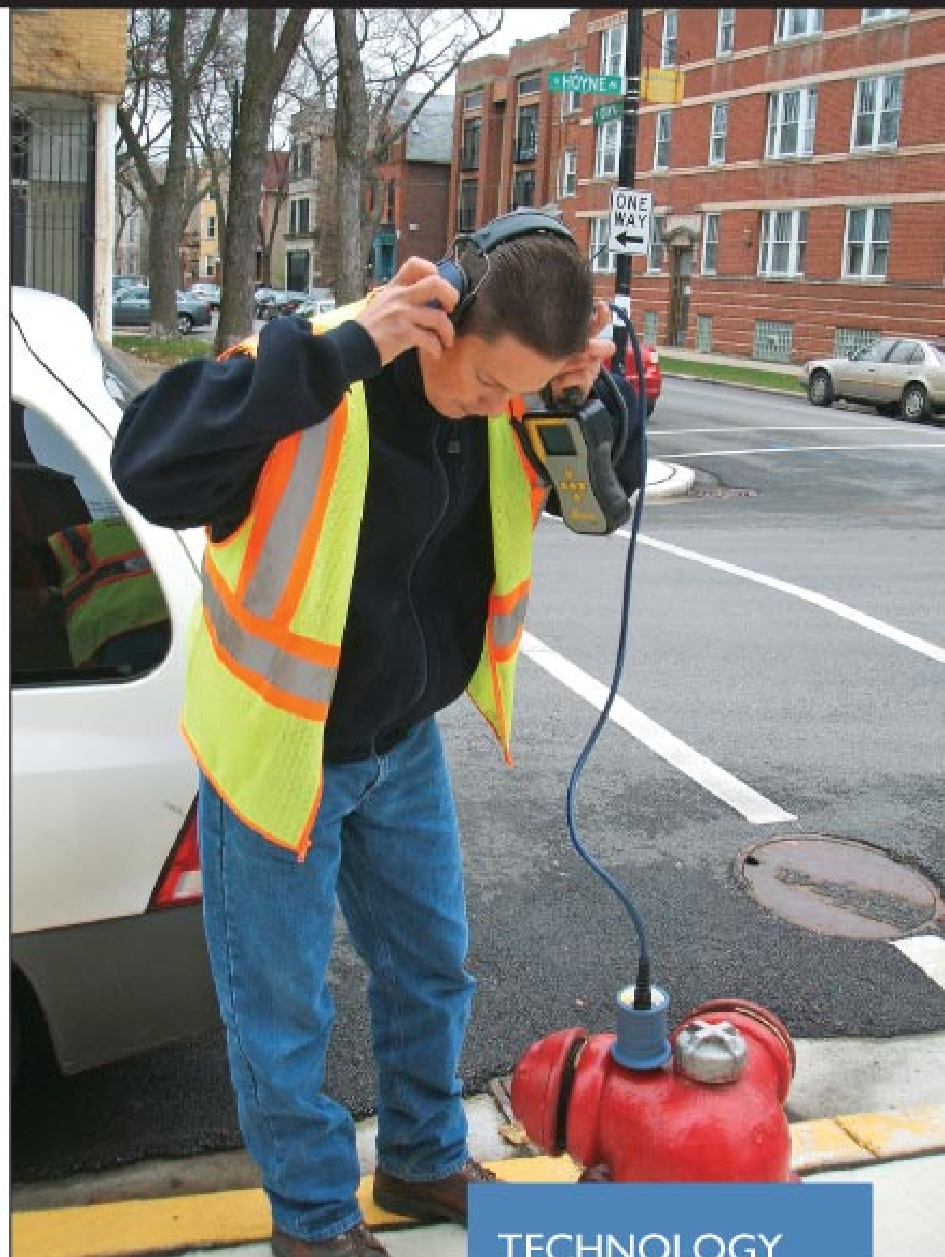
Bill Doyle of ADS Environmental Services listens through headphones to the sound being picked up by a Mikron Alpha as it picks up noise from a nearby leak through the fire hydrant connected to the water system. (Photos by Erik Gunn)
