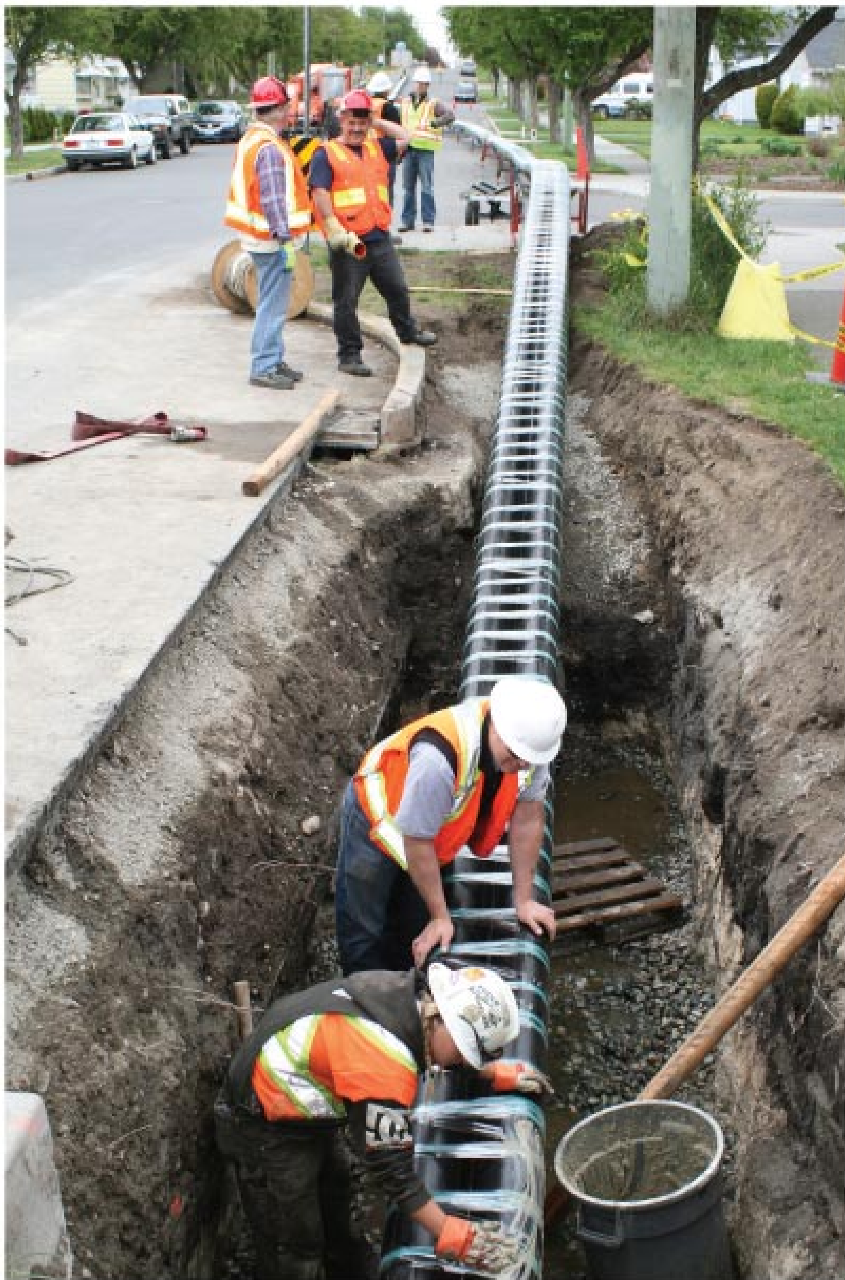
The folded liner is inserted into the entry pit.
