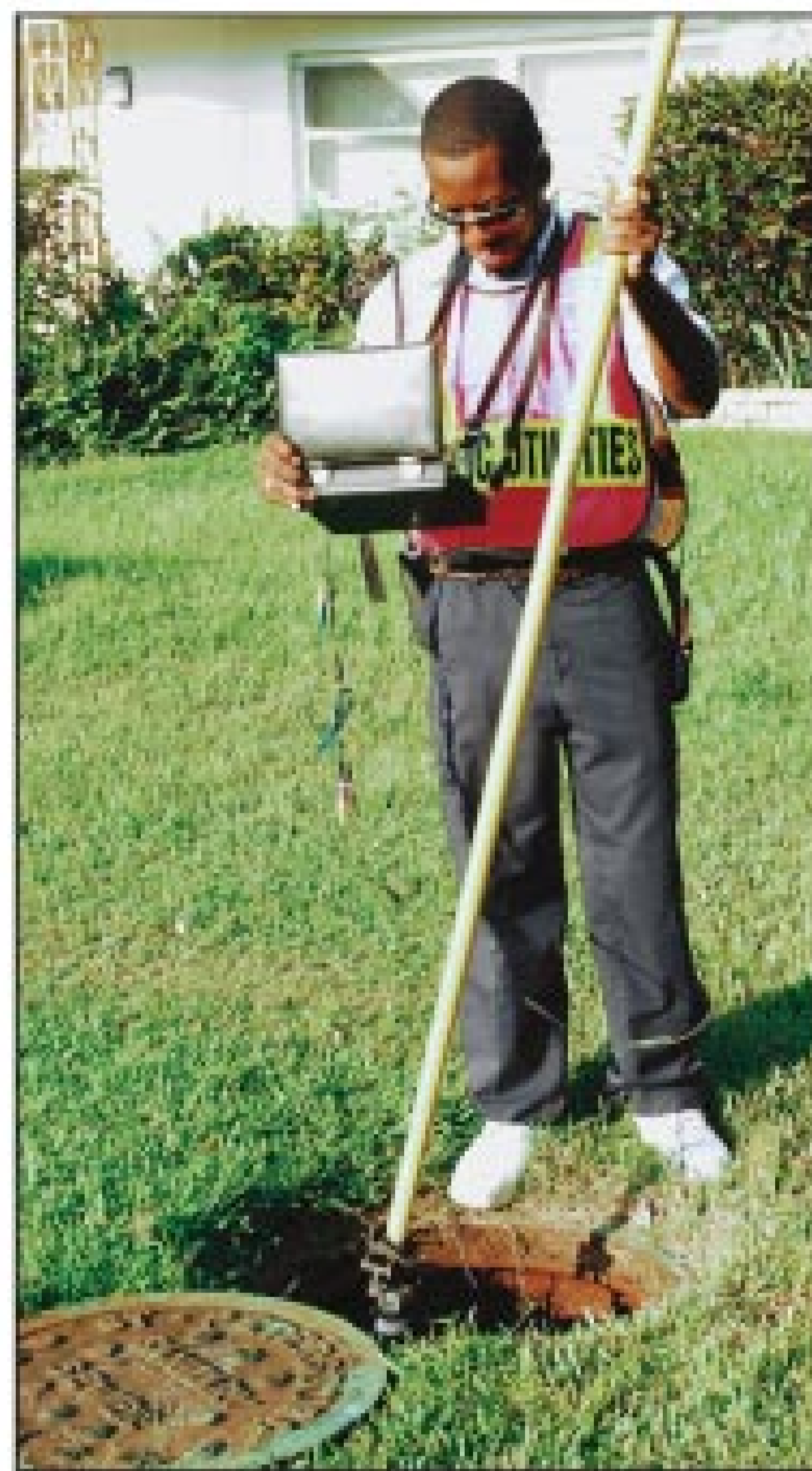
Above, the Quick Television crew from the city's Preventive Maintenance Section uses a pole camera to inspect sewers. Operating the camera is wastewater technician DiMario McKenzie. Right, wastewater technician John Martin cleans a line as wastewater collections system maintenance division manager Lane Longley observes.
