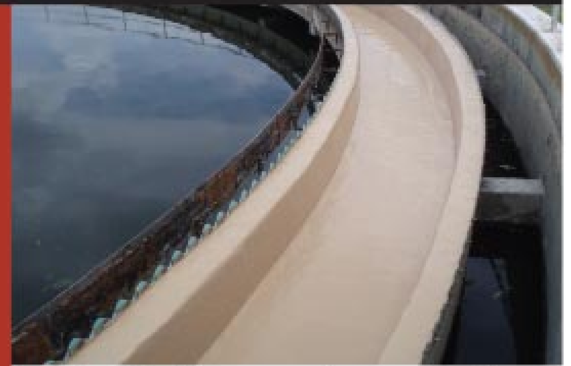
"Over 3-million square feet coated with Miami-Dade Water & Sewer"
