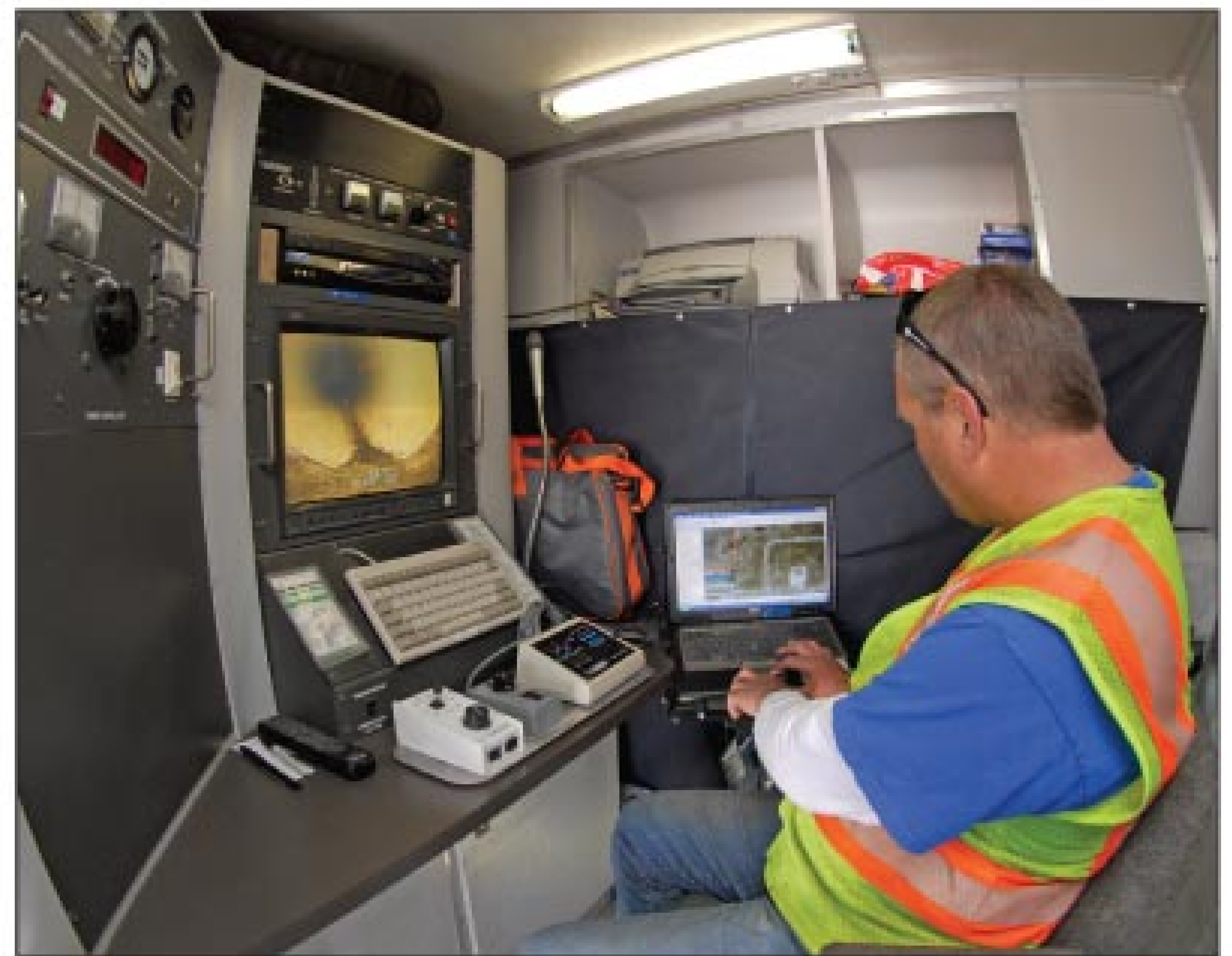
Maintenance worker Brian Hurd and colleagues perform in-house line inspections that are helping the City of Ames improve customer service and save money.
