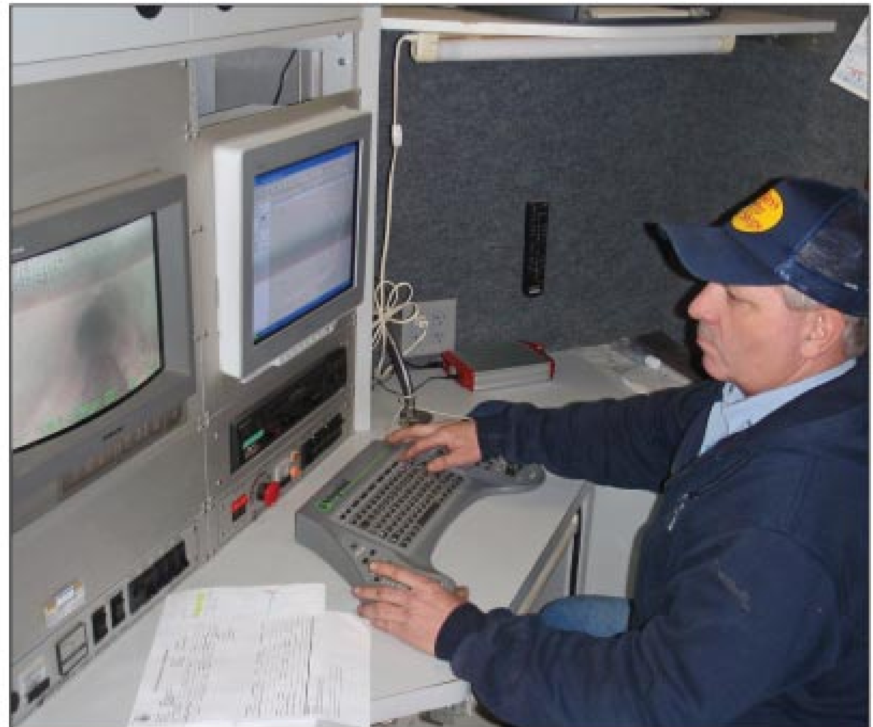
The inspector on the Lee's Summit video truck has two monitors: one to watch video and one to enter pipe conditions into flexidata survey software. Equipment operator Kenny Moore controls the camera and records observations. (Photo courtesy of Lee's Summit)
