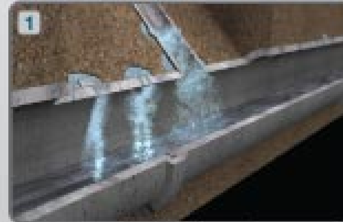
Leaking lateral
