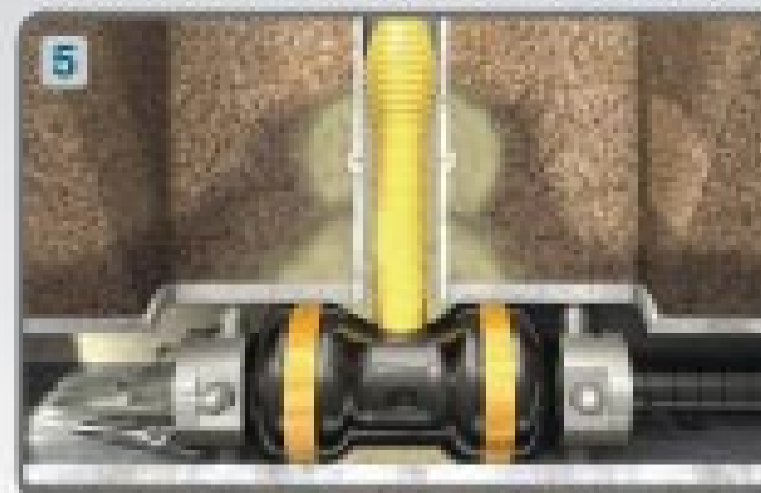
Lateral packer injecting grout
