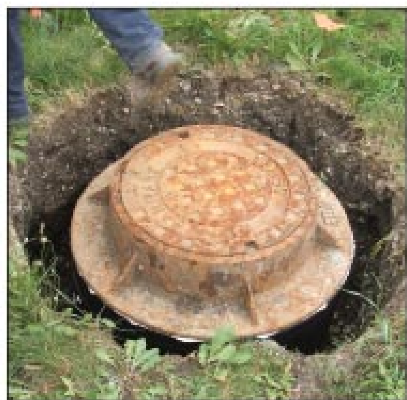
The frame in place.
