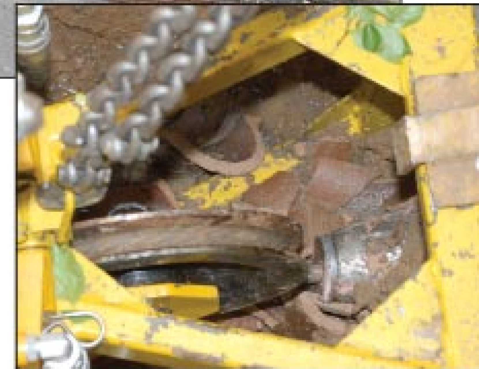
The bursting head appears in the exit pit amid shards of the old terra cotta pipe.
