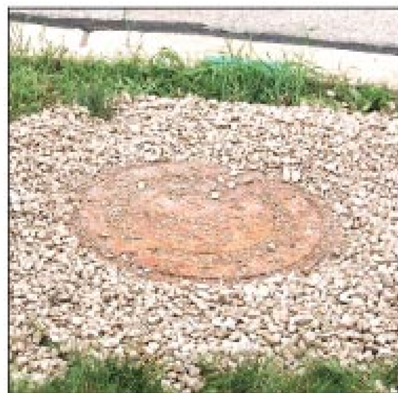
A repaired manhole with gravel fill around it.
