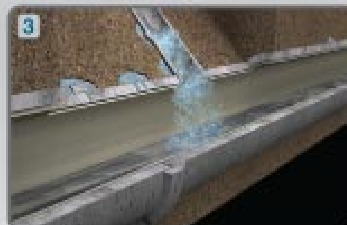
Continues to leak in annular space
