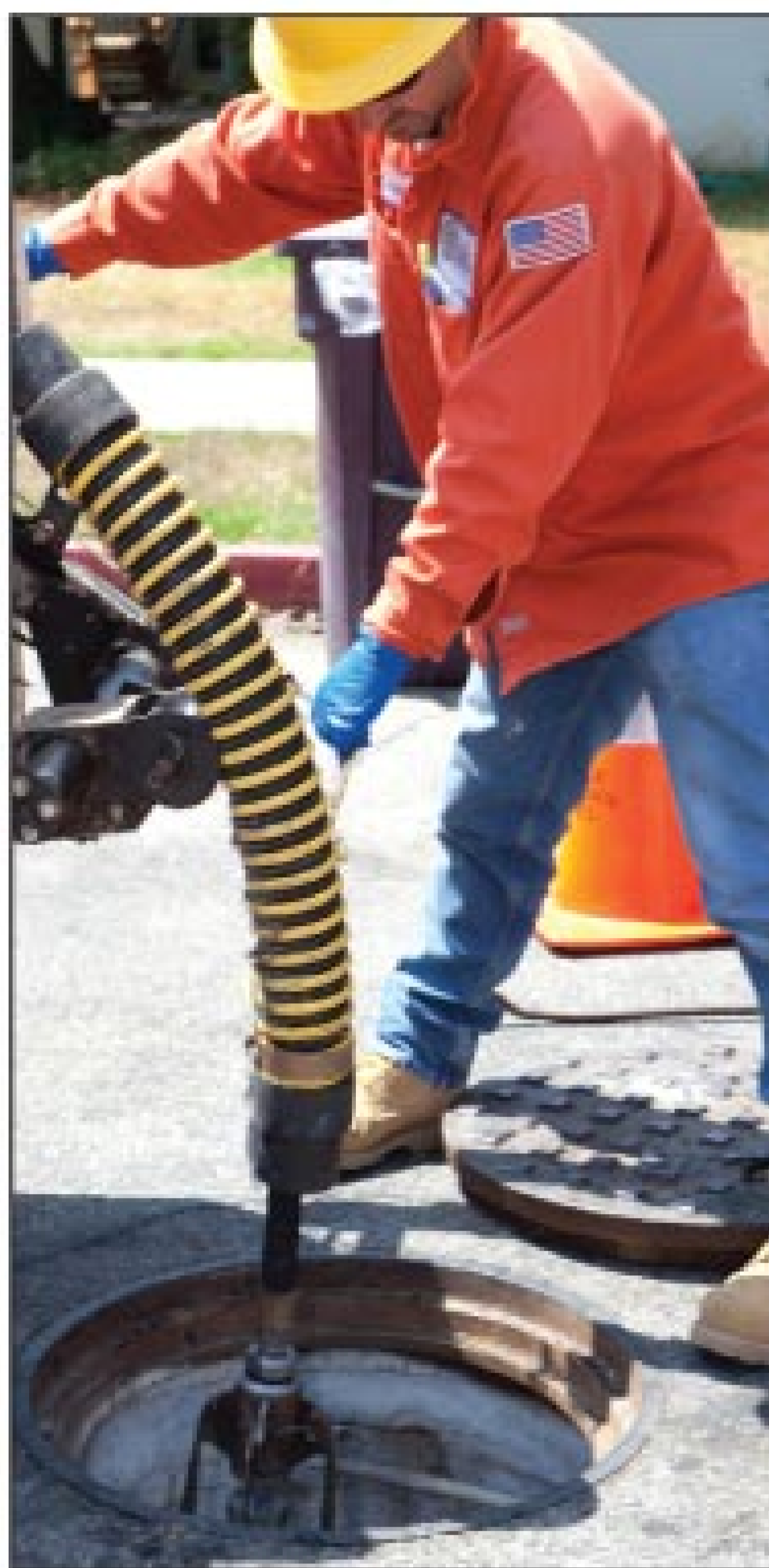
Wastewater maintenance worker Jason Badgley lowers a cleaning nozzle into a manhole.
