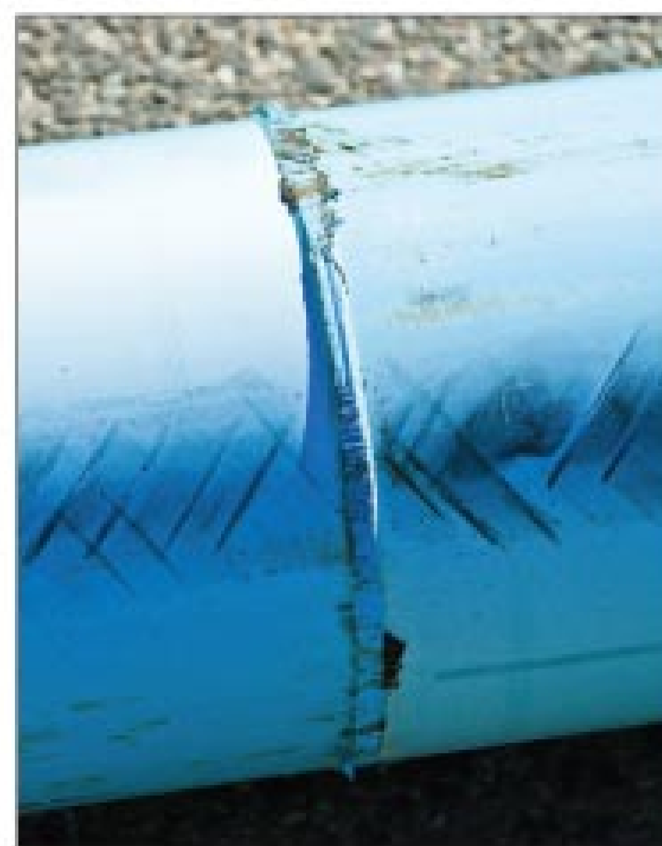
A finished fused joint between two sections of fusible PVC pipe.
