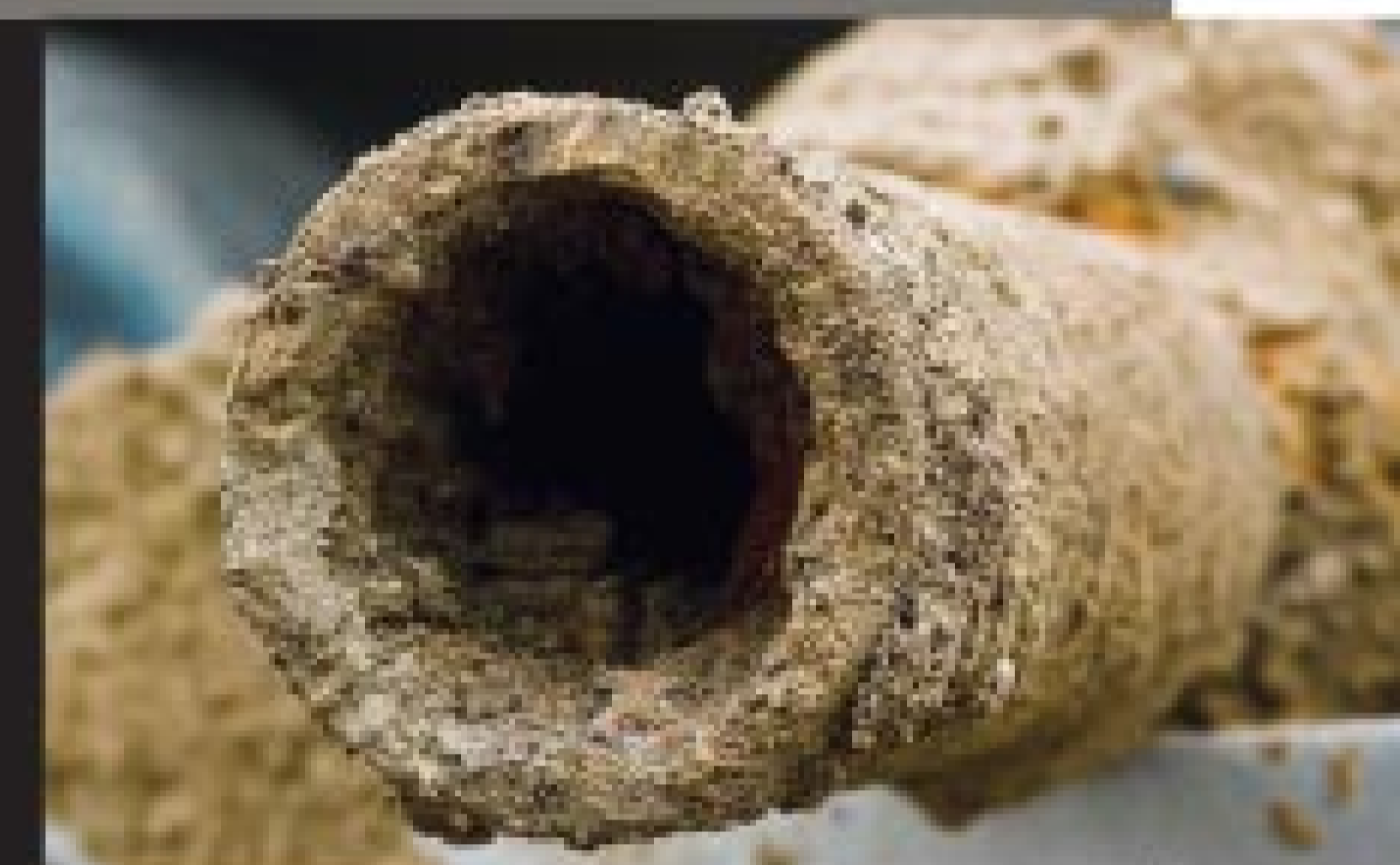
A section of old 4-inch cast iron pipe installed in 1916.
