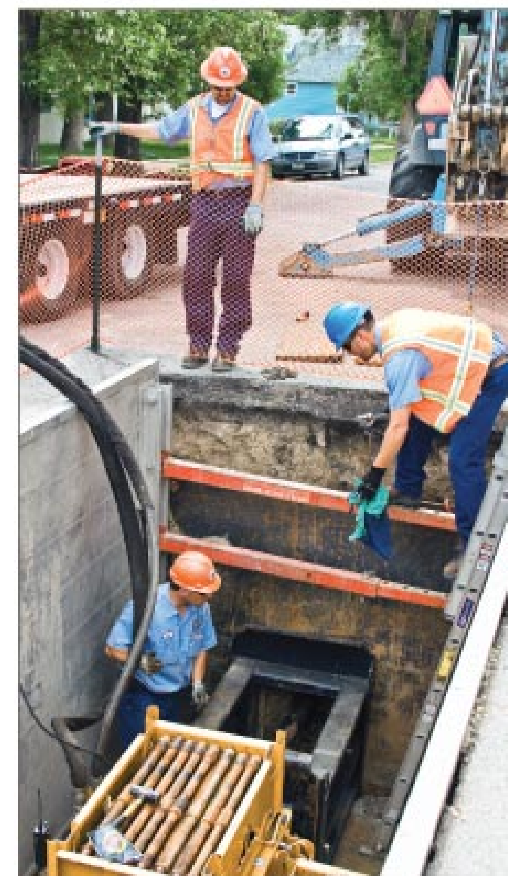
J.R. Fox (in excavation) realigns the HammerHead pulling unit while Scott Haynes (right) and Ryan Skillestad assist.
