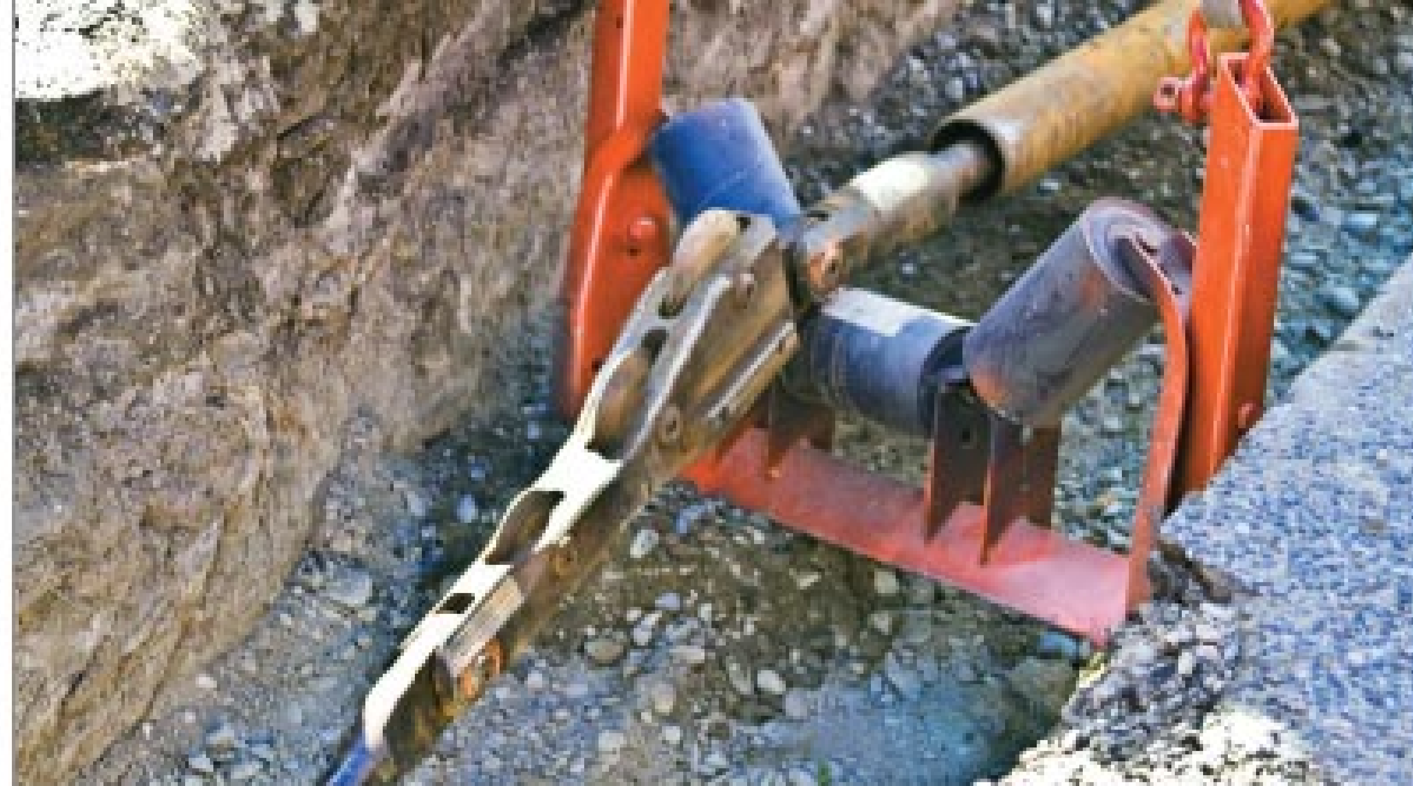
The slitter section of the pipe bursting system.
