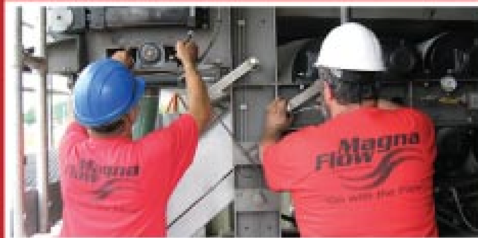
Belt Press Repair & Maintenance
