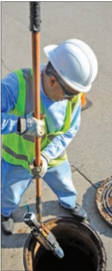
Maintenance worker Alejandro Escobar lowers a camera into a sewer line for an inspection. Fort Worth operates nine camera vans.
