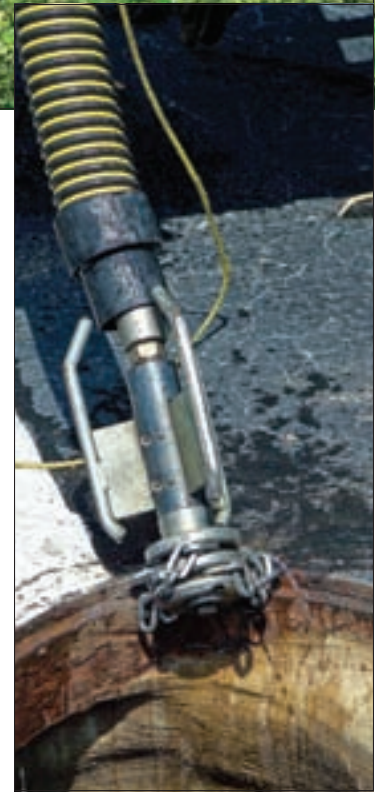
A root cutter tool being removed from a sewer line.
