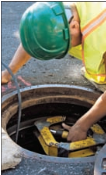
A tool is used to tighten the steel bands on the chimney seal.
