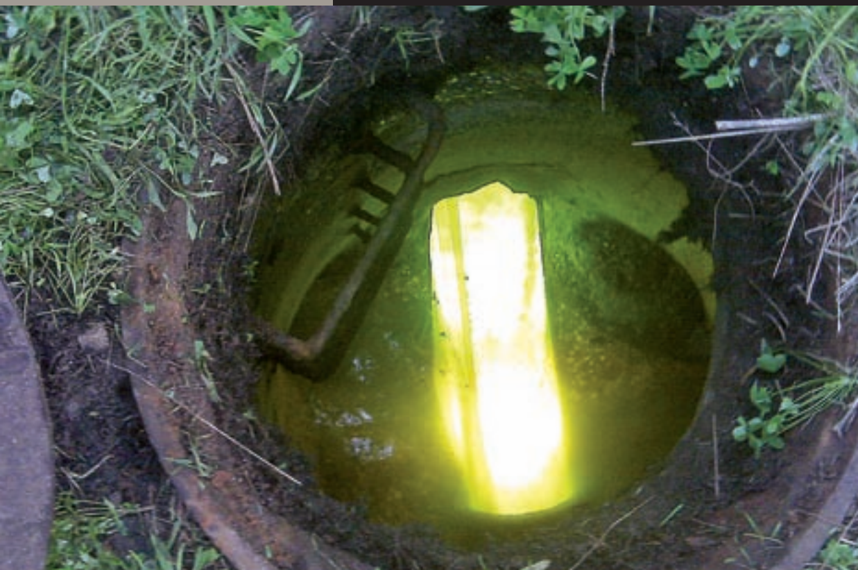
The UV light train cures a segment of 12-inch liner. (Photos courtesy of Dexal Construction)
