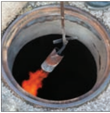
Left, a torch is used to dry the surface before priming of the manhole in preparation for sealing. Right, the manhole surface with the topcoat in place.
