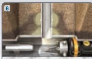
Grout collar stops infiltration
