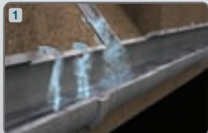
Leaking lateral
