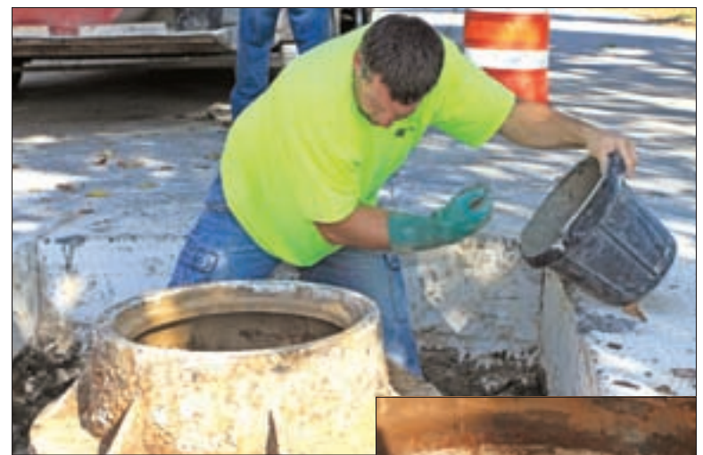
Mason Ryan Vandergalien applies mortar inside the rebuilt manhole chimney. (Photo by David Hoel)
