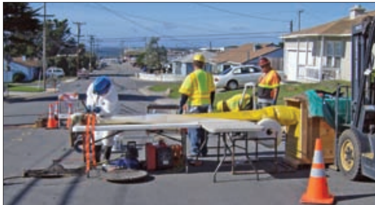
Rory Simon, a LightStream consultant, tightens the straps that hold the folded-back liner nose together.
