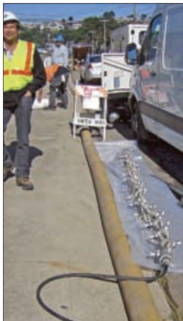
The 13-foot-long light train includes eight UV lights. Joe Kauwe from the North Marin Water District in Novato, Calif., watches the liner installation.
