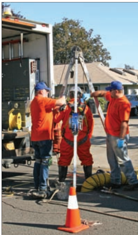
Flow monitoring technician Archie Richardson prepares to enter a manhole to do urethane grouting. Maintenance operators Jay Smith, left, and Randy Tadlock assist.
