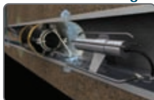
Leaking joint in mainline sewer
