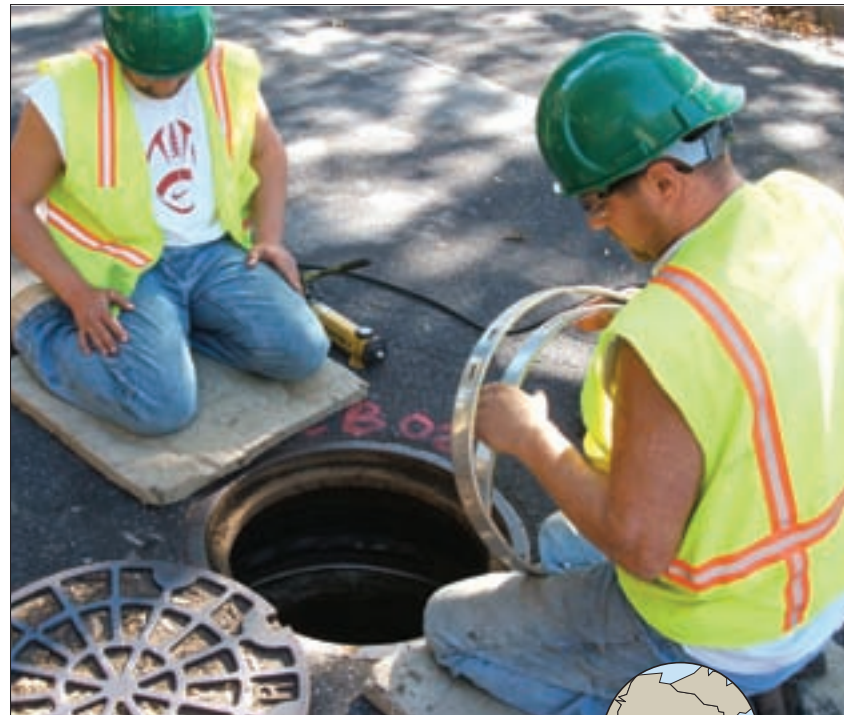
City crew members Wayne Zwicker (left) and Brandon Ottson prepare to install a second set of compression bands on a manhole chimney seal from Cretex Specialty Products. (Photography by Erik Gunn)
