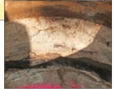
An example of deterioration in a manhole needing rehabilitation.
