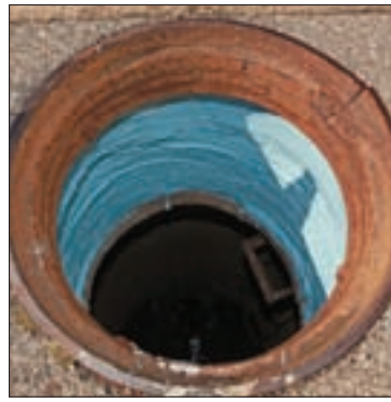
Left, a torch is used to dry the surface before priming of the manhole in preparation for sealing. Right, the manhole surface with the topcoat in place.
