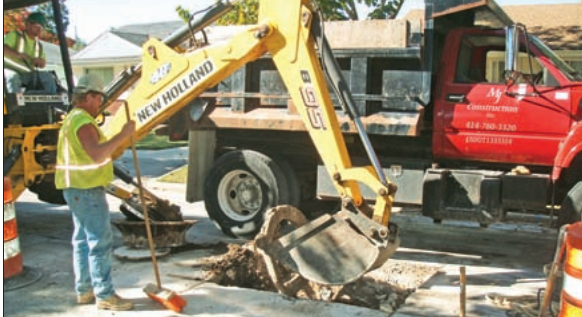
John Fuller, operating a backhoe, removes the frame and chimney rubble from the manhole area.
