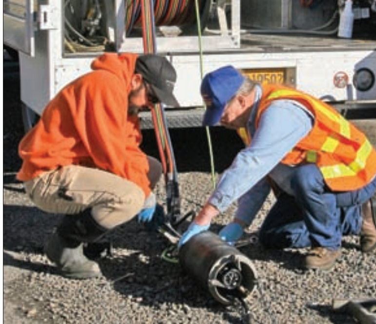
Maintenance operator Shawn Bernards, left, and sewer instrument technician Ric Hines prepare to lower the Logiball 2001JS mainline grout packer into a manhole.
