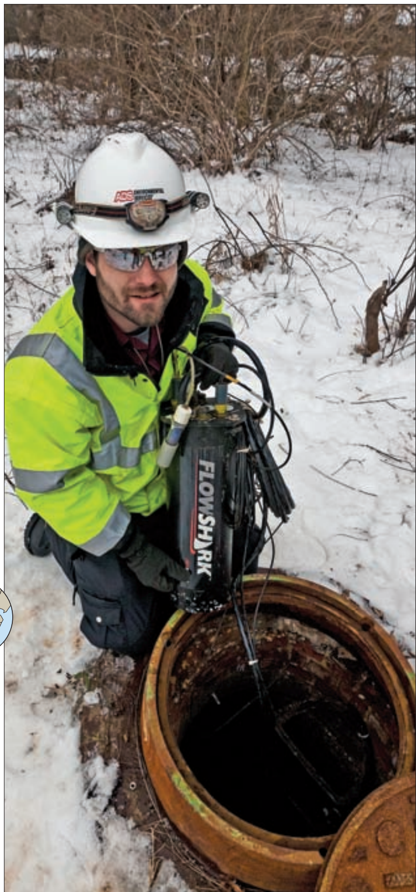
ADS Environmental Services field representative Jacob Deaner prepares a FlowShark sensor for attachment to a manhole. The sensors are a key part of WSSC's effort to optimize capacity and reduce SSOs. (Photography by Andrew Lightman)
