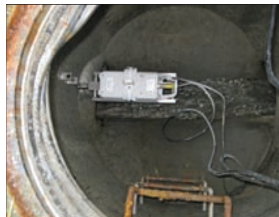
A non-contact Flo-Dar area velocity sensor in a 16-inch sanitary sewer line.
