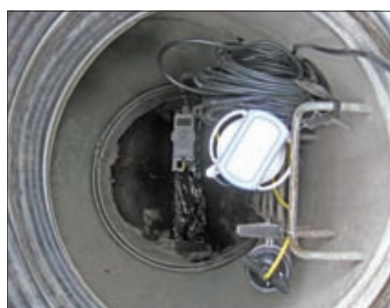
A Flo-Dar sensor is installed with cellular-equipped logger and long life battery pack.
