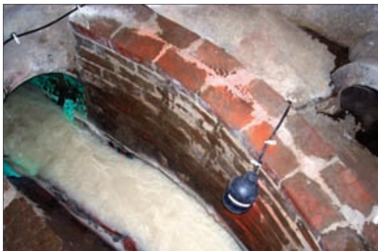
A FlowAlert pressure level sensor is installed in the flow, and the float alarm switch is on the weir wall.
