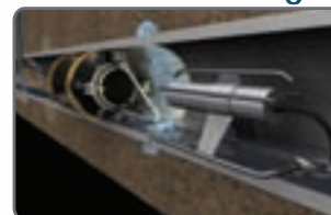
Leaking joint in mainline sewer
