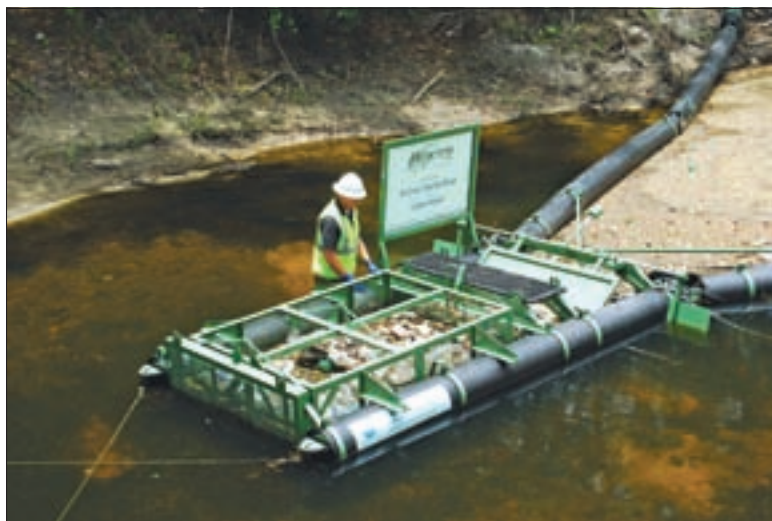
A Bandalong Litter Trap is installed on the main city drainage canal below the last confluence point before discharge to the Satilla River. Will Corbett closes the trap gate in preparation for removing the basket.
