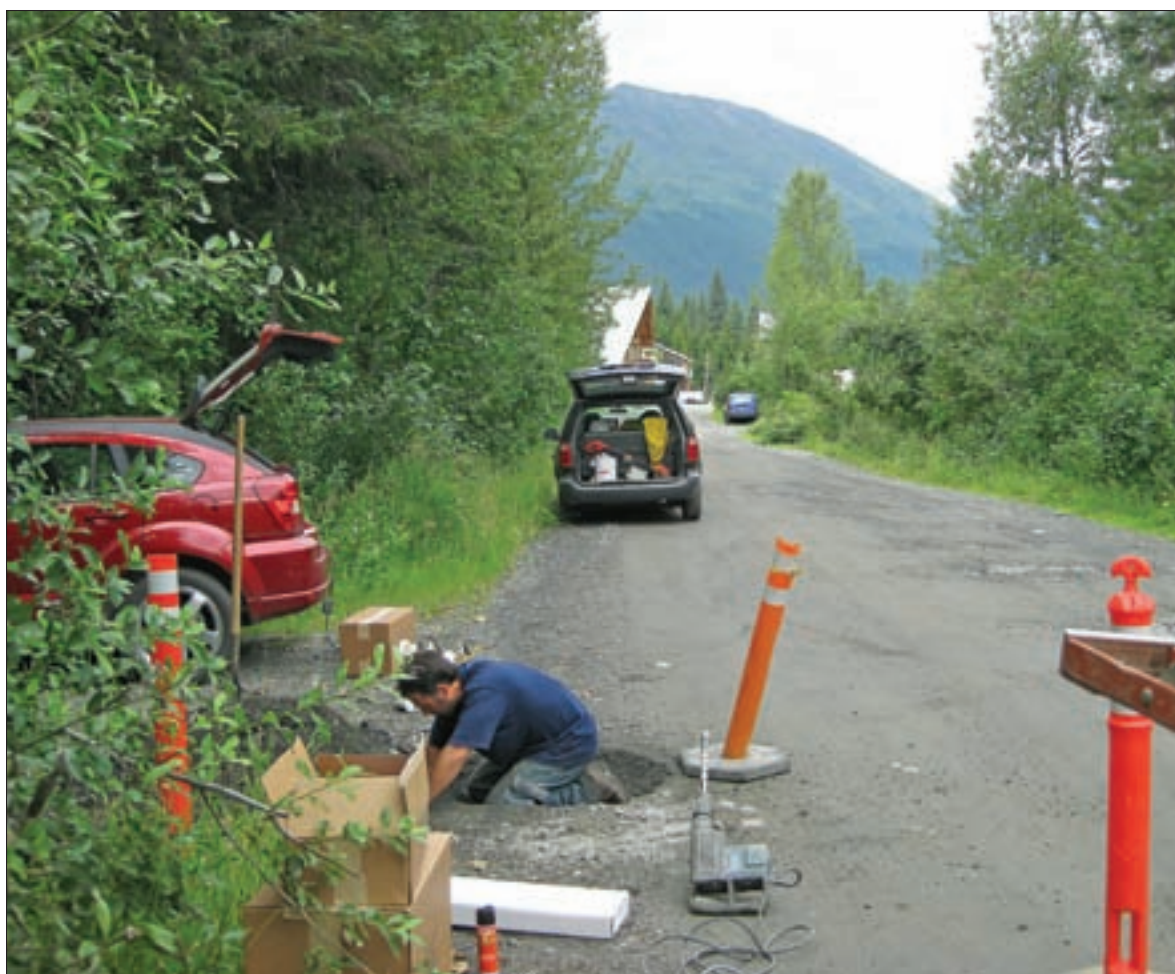
An employee of Frawner Corporation installs a Flo-Dar system.
