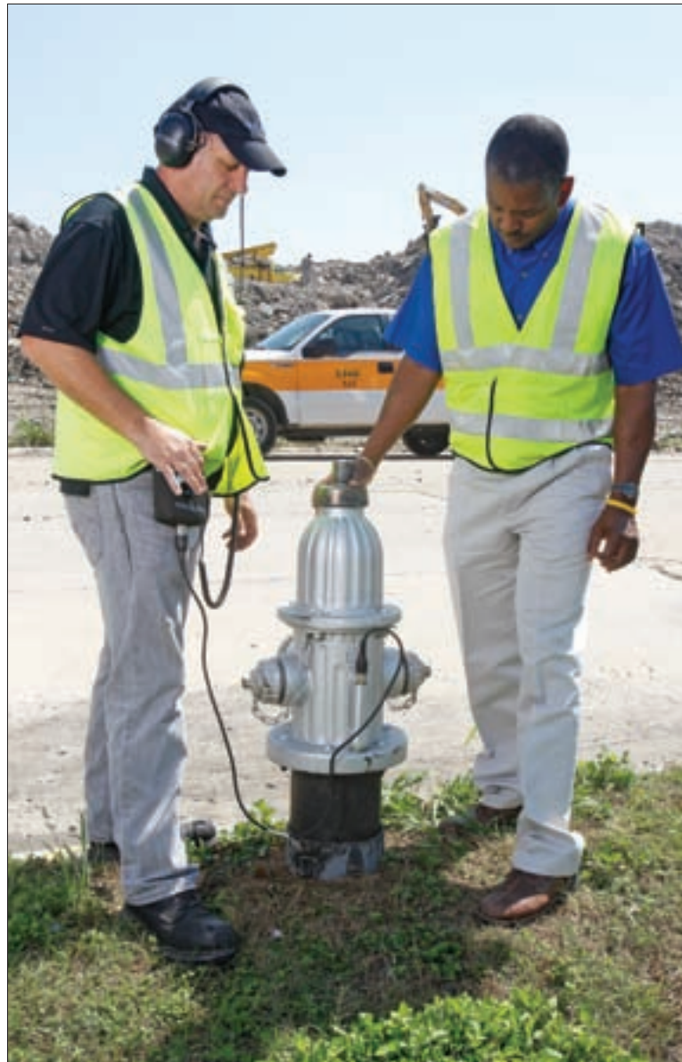
Frank Hobbs (left) and Rudy August listen for leaks.
