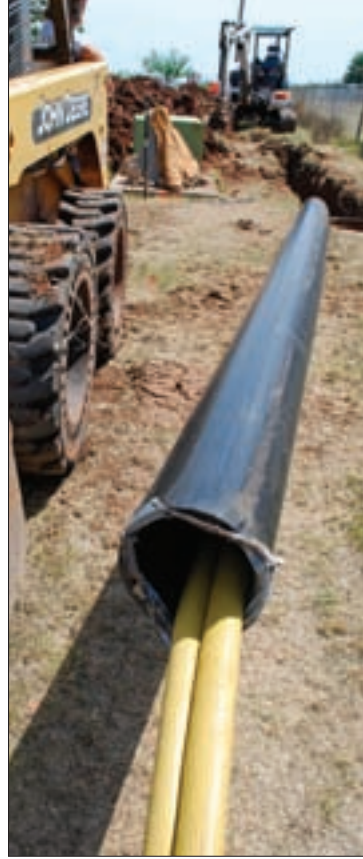
Lengths of 8-inch HDPE pipe are pulled into a trench.
