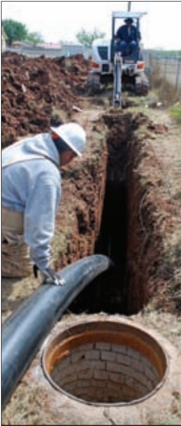
Lengths of 8-inch HDPE pipe are pulled into a trench.
