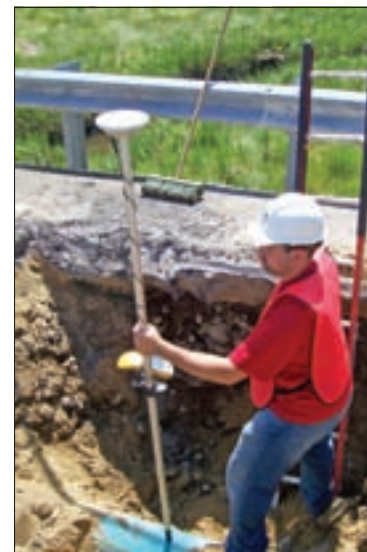
Resident engineers maintained written field notes that located critical components of the distribution system, such as valves, fittings and couplings. Crews also used a Trimble handheld real-time GPS device to collect as-built information.
