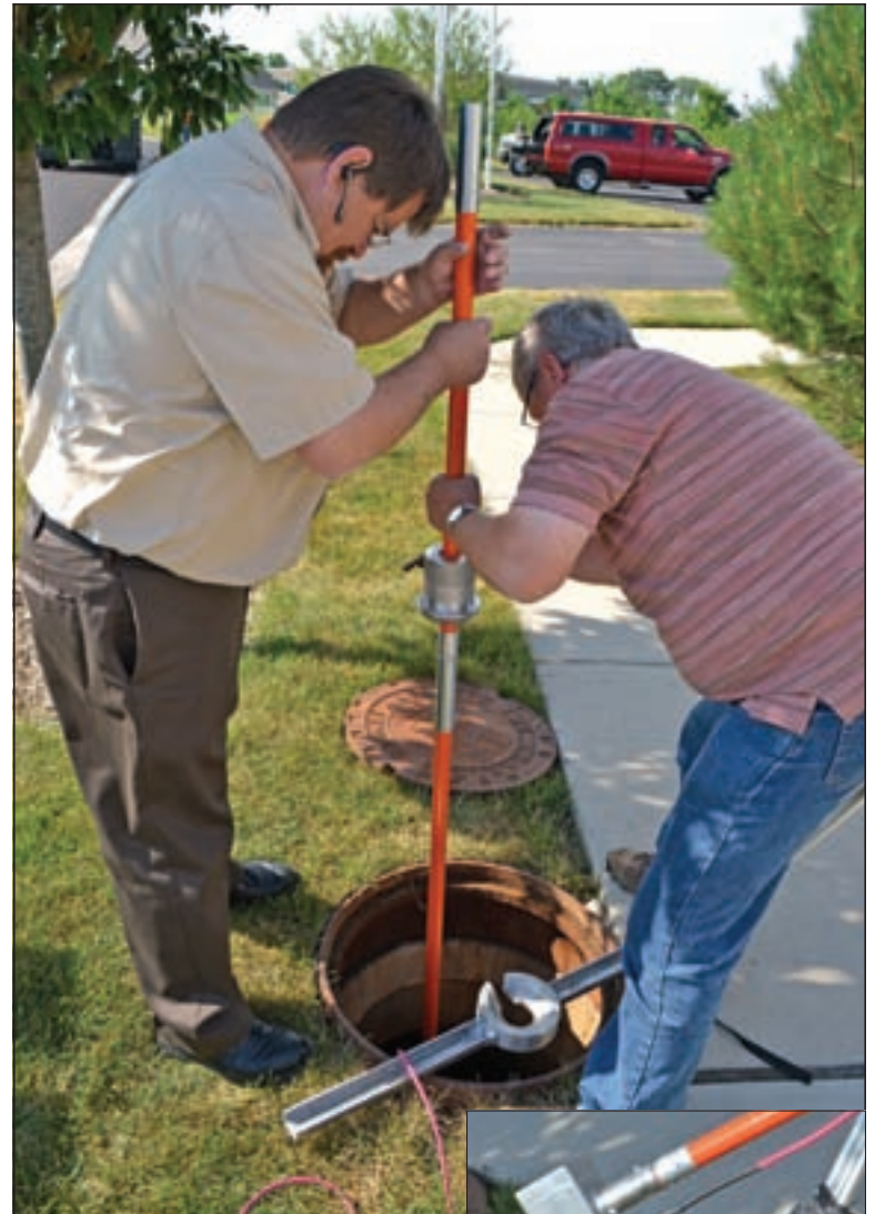
Dan Story (left) and Guenter Schaarschmidt position the pole inside a collar that holds the pole for the wireless receiver.
