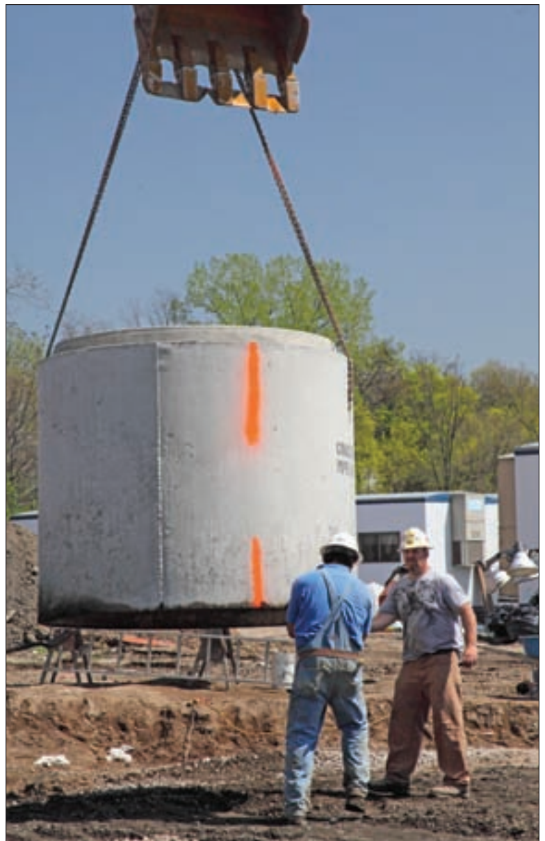
By 2014, the district will add another 10,000 residents, along with 19 miles of sewer line and five more pump stations from the Village of Great Neck, just to the north. This treatment plant expansion will handle the additional load.
