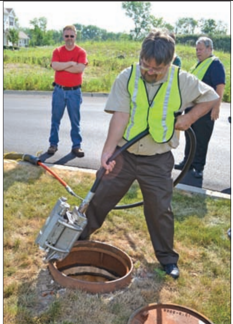
Dan Story lowers the 65-pound Kleen-Vue unit into the manhole.
