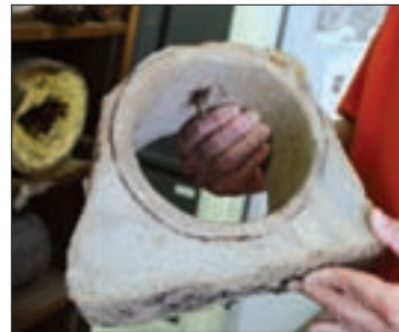
An old piece of wooden pipe that the city Public Works Department keeps on display in the office.
