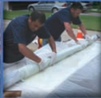
Sectional Main Line Point Repair™
