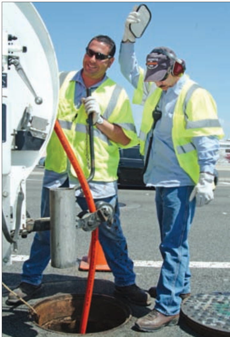
Mechanic Bryan Blair, left, and lead mechanic Peter Cheffs use the Vector 2100 to jet a manhole. Cheffs holds a mirror to assess the progress.
