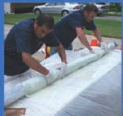
Sectional Main Line Point Repair™
