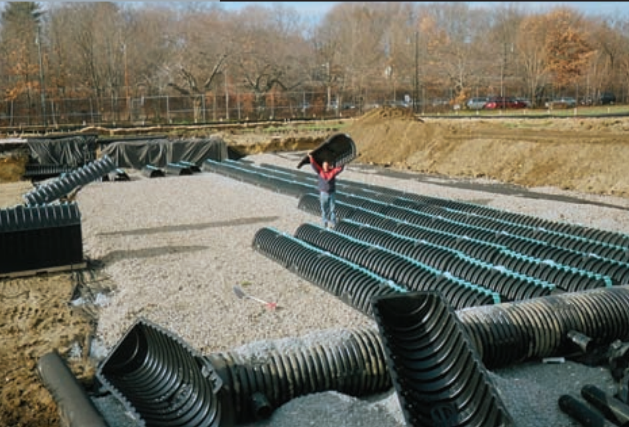
At 18.5 inches high, Recharger 150HD lower-profile chambers are used for sites with depth restrictions or when larger infiltrative areas are required. (Photo courtesy of CULTEC)
