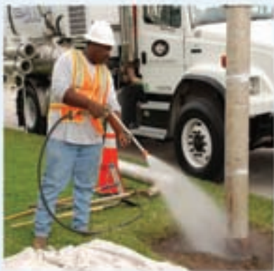
No Open Trenches
