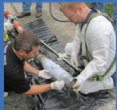
InnerSeal™ Innerwrap™ Lateral Connection Seal
