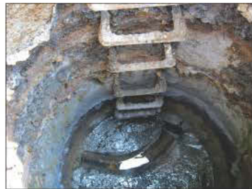
LEFT: Hydrogen sulfide ate through an epoxy lining and attacked the concrete manhole. RIGHT: Hydrogen sulfide corrosion in a 6-inch force main. A worker's shovel went straight through the main during excavation.
