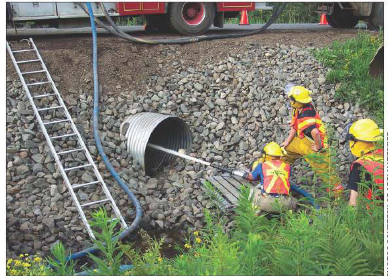
The township of O'Connor Fire Department assisted the Ontario Ministry of Transportation in clearing the culvert with an experimental high-pressure water method using a fire engine.
