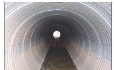
The culvert after high-pressure water cleaning.
