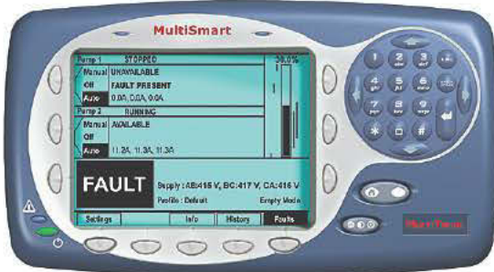
Screen readout on the MultiSmart control when a fault occurs.
