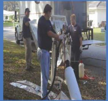
Perma-Main™ Continuous Air Inversion
