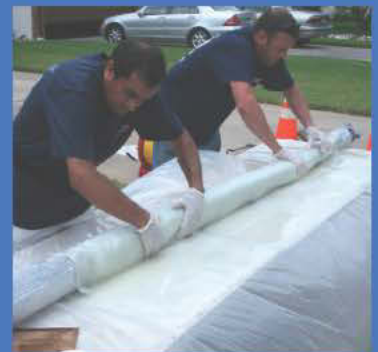
Sectional Main Line Point Repair™
