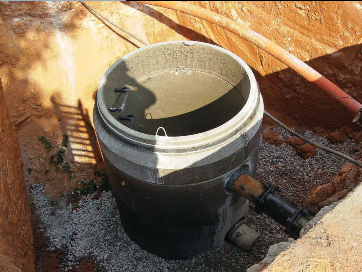
A composite manhole replaces a manhole approaching failure in a lightly used turn lane. (Photos courtesy of Gwinnett County Public Utilities)
