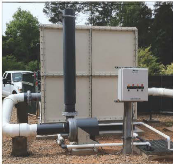
The custom-built, pre-engineered Mönashell bio-filtration system from Anua is 8.5 feet square and weighs 20,000 pounds with seashells.
