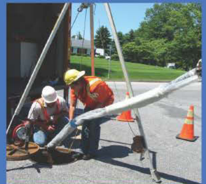
Sectional Main Line Point Repair™
