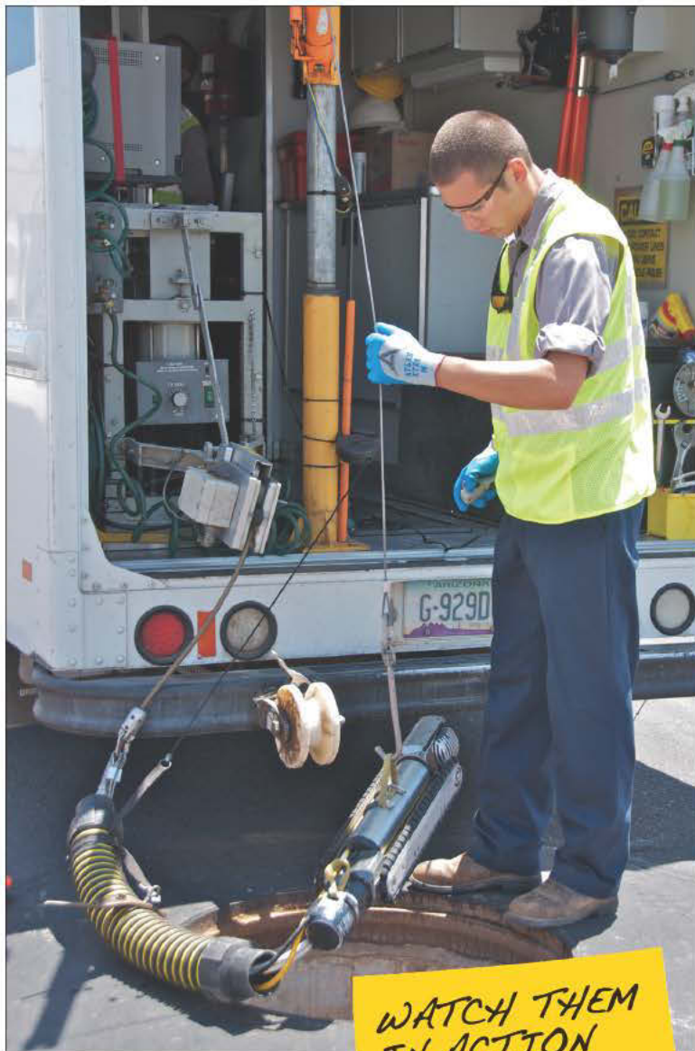
Angelo Valdez lowers the CUES camera into a manhole for inspection.
