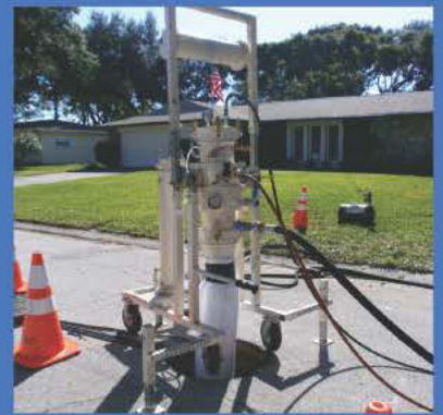
Perma-Main™ Continuous Air Inversion
