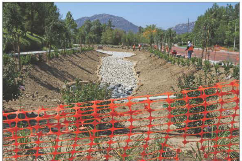
An infiltration basin in a new residential development in Temecula collects stormwater and filters it through layers of rock and sand into the ground, helping to replenish the groundwater aquifer.
