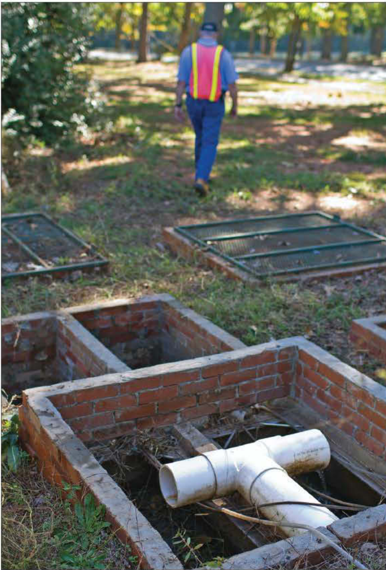
A technician heads downstream for a stormwater sample. One of the city's modified Delaware sand filters is in the foreground.
