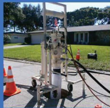
Perma-Main™ Continuous Air Inversion
