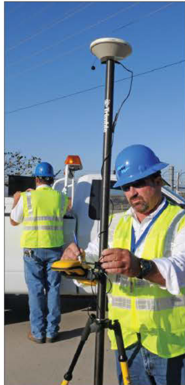
Senior operations technicians Chuck Hunt, left, and Todd Fielding use a laptop and Trimble GPS unit to gather coordinates for the location of pipes or valves. The antenna gathers data from different satellites and gives the operator the coordinates.
