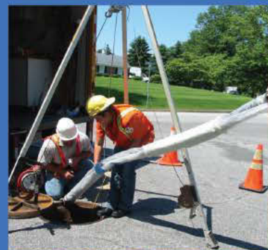
Sectional Main Line Point Repair™
