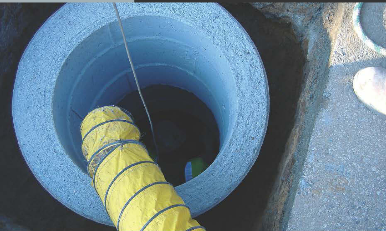
A manhole in Waupaca, Wis., after structural rehabilitation with the Monoform system. (Photos courtesy of Infratech Infrastructure Technologies)
