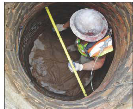
Infratech project manager Ed Brown measures the diameter of a manhole to select the proper-size forms.
