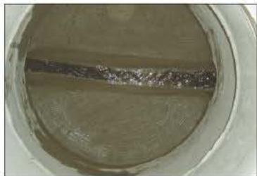
A bench with flow channel is constructed one inch above the crown of the pipe.
