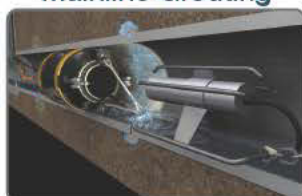
Leaking joint in mainline sewer
