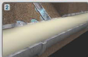
Liner installed
