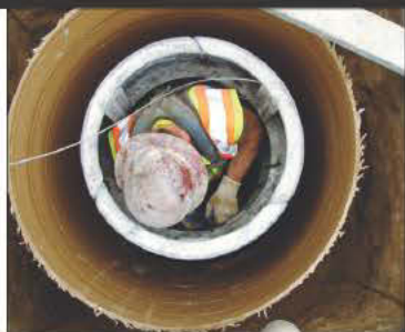
The custom-made Monoform sections are fastened with C-clamps.
