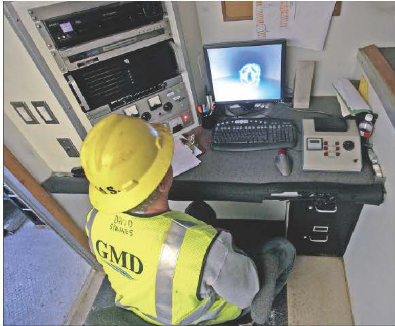
Camera operator David Symmes watches the lining of a sewer from a PowerVision camera (Power Equipment Mfg. Inc.) that is attached to a remote vehicle inside of the sewer system.
