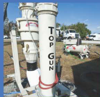
Perma-Main™ Continuous Air Inversion
