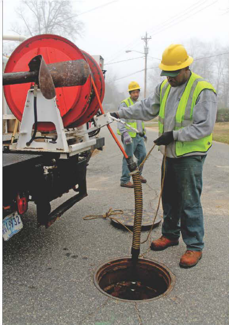
Crew members Vernon Griffin, background, and Marvin Adams use a jetter from US Jetting to clean a residential sewer line.
