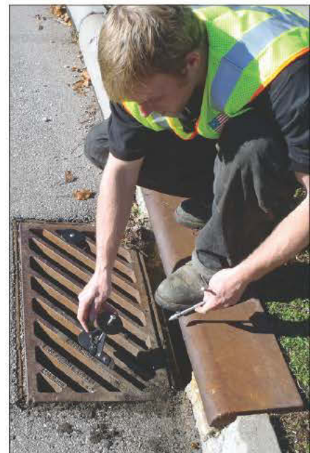
The grate lock design is based loosely on a C-clamp (a demonstration video can be viewed at www.mattlocksusa.com ). The user positions the device in the storm grate and uses a special wrench to turn a tamper-proof bolt and tighten it down.
