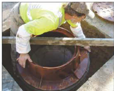
Ed Brown installs the new manhole frame and lid.
