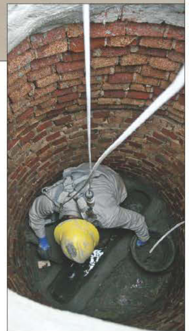
Crew member Mathew Overstreet repairs the inside of a manhole with Quadex sewer rehabilitation products.
