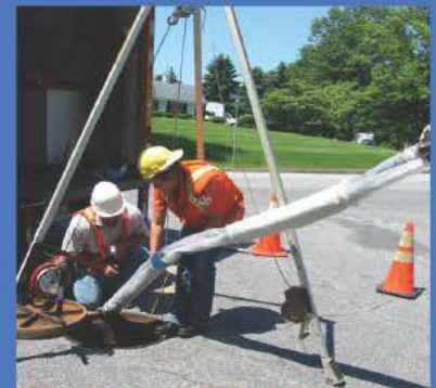
Sectional Main Line Point Repair™
