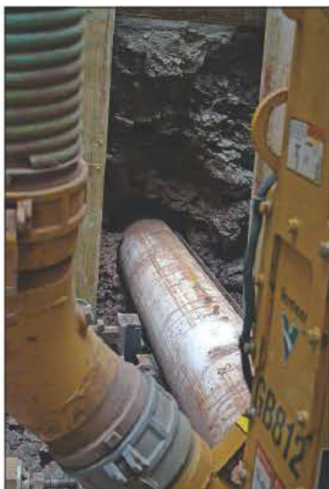
A closer look at the auger boring into the underground rock.
