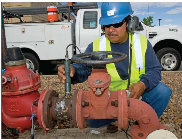
Water maintenance mechanic Hector Razo uses a Fluid Conservation Systems digital correlator with a microphone to listen for leaks.
