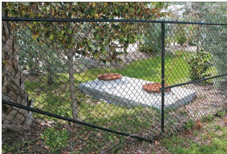
ABOVE: Portions of Marathon's wastewater infrastructure, including vacuum pits, are visible in residential areas. RIGHT: "Candy cane" risers allow the vacuum system to pull in air.
