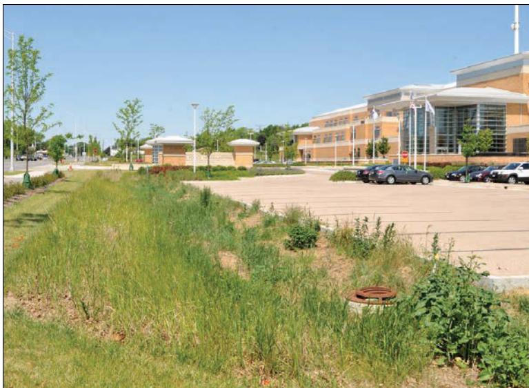
The new Aurora Police Department building has earned awards for its green features, including this stormwater drainage project.
