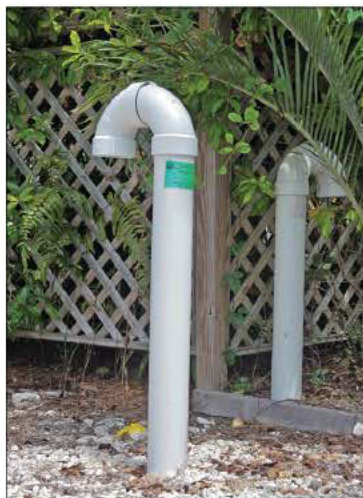
ABOVE: Portions of Marathon's wastewater infrastructure, including vacuum pits, are visible in residential areas. RIGHT: "Candy cane" risers allow the vacuum system to pull in air.
