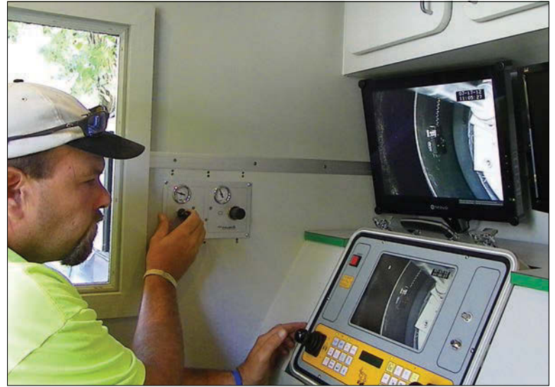
Rausch USA’s Jeff Rager monitors progress from the control cab as he works the pneumatic controls that inflate and deflate the bladder.
