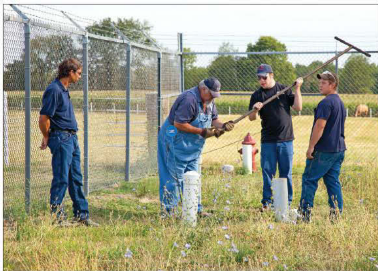
Alliance System manager Jon Rogers, left, oversees as foreman Roger Nichols and employees Tyler Stuhman and Devon Muehring clean out and shut off water tower valves.
