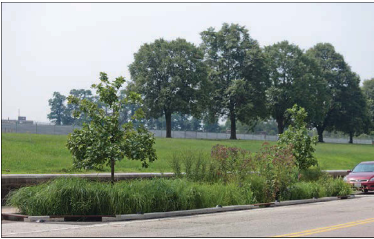
The Philadelphia Water Department's Queens Lane Reservoir includes bump-outs for rainwater reclamation, reservoir banks and the purified water reservoir.
