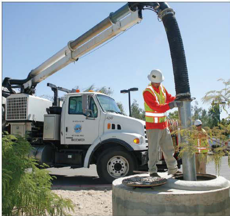
Josh Wehner cleans out a manhole at Rotary Community Park with the vacuum hose from a Vactor truck.
