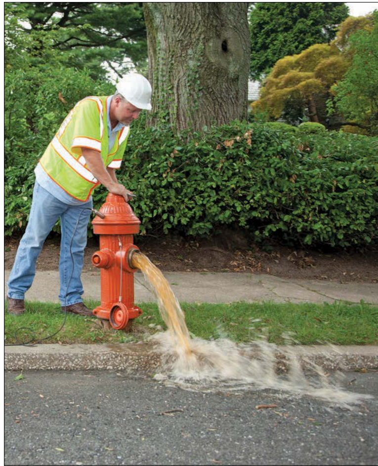
Water conveyance supervisor John Bevan runs a hydrant to find the pressure rating and determine if there is a leak.
