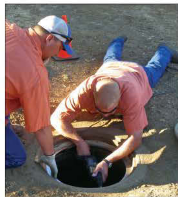
Public Works operator Cody Nissen, left, steadies a SewerLock insert while Jeremy Wachtel uses a roto-hammer drill to bore holes in the concrete manhole cover frame. A portable Honda 2,000-watt generator supplies the power.
