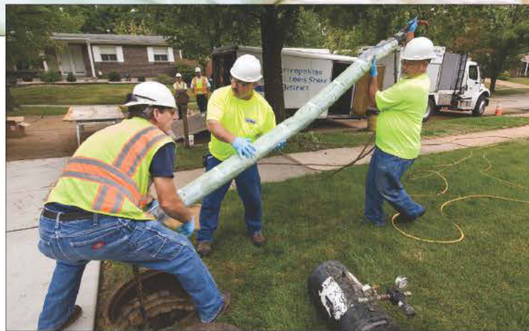
Frank Coleman, left, Dan Kateman and Gregg Hall prepare an Infrastructure Point Repair System liner for a pipeline rehabilitation job. RIGHT: The liner is ready to be lowered into the pipe.
