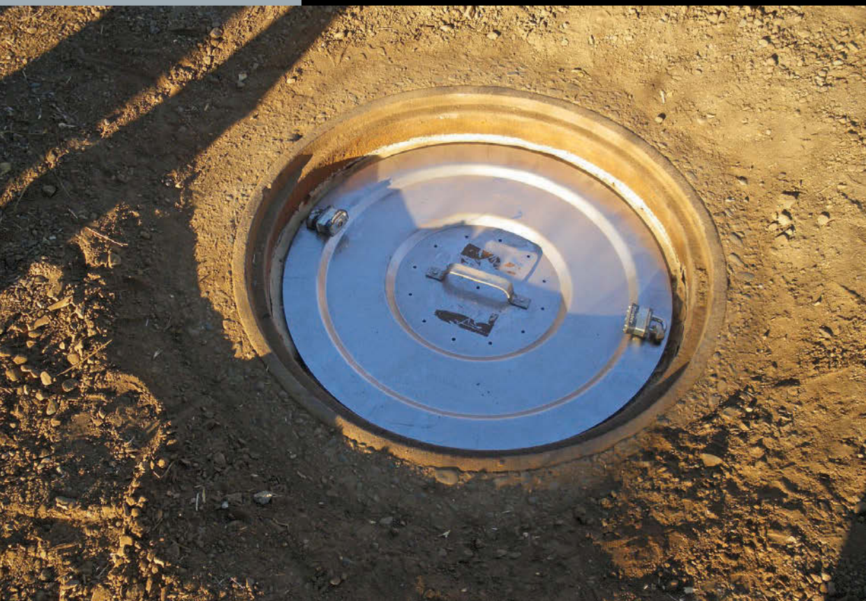
The stainless steel SewerLock cover locks to the insert rim with two laminated, commercial Master Lock keyed padlocks. The entire installation takes about 30 minutes. (Photos courtesy of Rick Walls)
