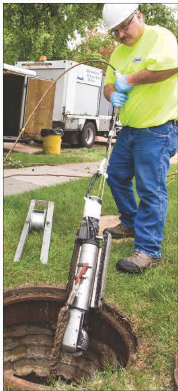
Construction laborer Frank Coleman pulls the CUES inspection camera out of a manhole after inspecting the sewer line.
