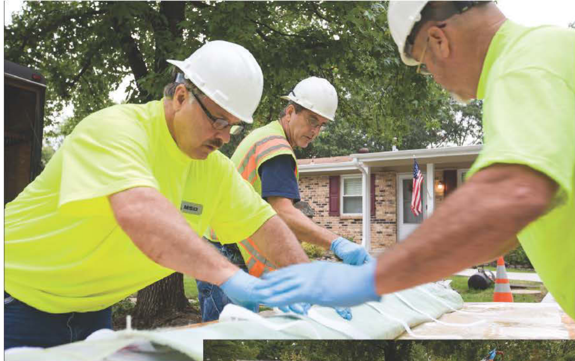
Frank Coleman, left, Dan Kateman and Gregg Hall prepare an Infrastructure Point Repair System liner for a pipeline rehabilitation job. RIGHT: The liner is ready to be lowered into the pipe.
