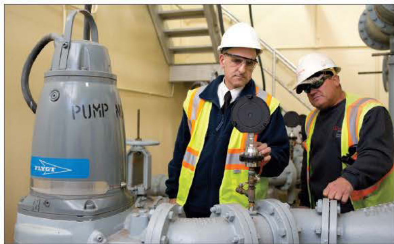
Administrator of community utilities Terry Sullivan, left, and CSO supervisor Alan Levrault check the Flygt dry-weather pumps (Xylem) for normal operation at the pump station.
