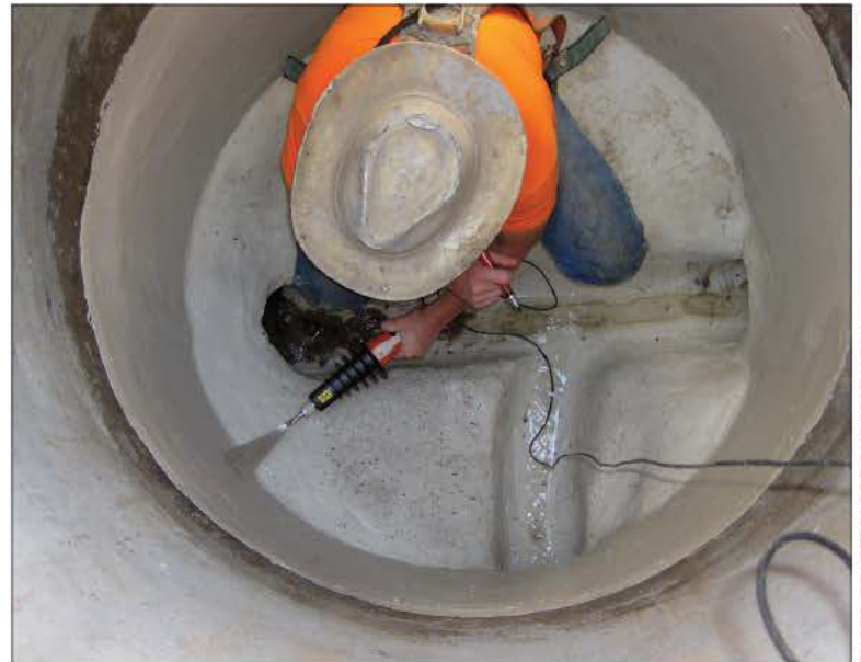
Dale Jarvis from subcontractor K&R Plumbing performs an electro test on an Epoxytec manhole liner.
