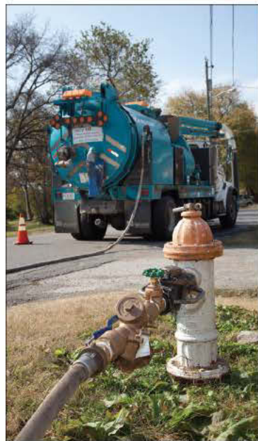
The Vac-Con combo unit is set up for water supply.
