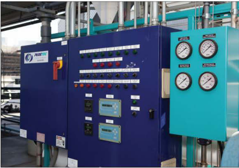
In order to use recycled water to generate power, the water must first be run through a reverse osmosis system. It is then subjected to another demineralization process, making the recycled water more filtered than distilled water (Puretec Industrial Water).
