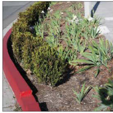
This pocket of greenery along the street allows stormwater to collect and irrigate before flowing into storm drains.
