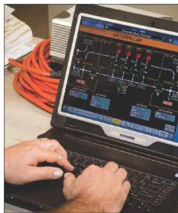
A maintenance employee uses the Caterpillar/ISO generator control system.
