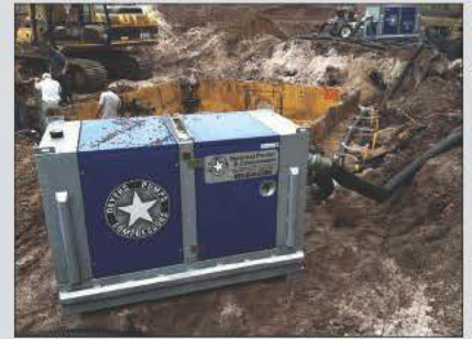
NPC PT-90 wellpoint pump from National Pump & Compressor
