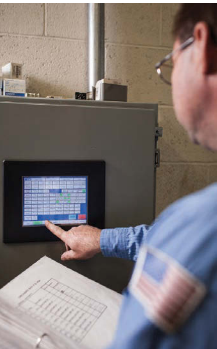
Alan Clanin uses an Automation Direct HMI that runs a SCADApack controller (Schneider Electric) to check the status of one of the 21 wastewater pumping stations.
