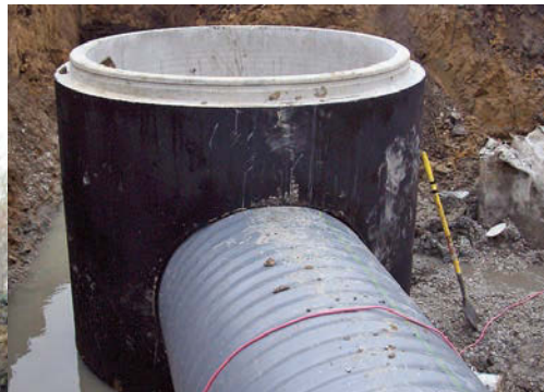
Connecting the triple-wall SaniTite HP pipe to precast concrete manholes was done without grout using an A-LOK mount with no additional adapters.
