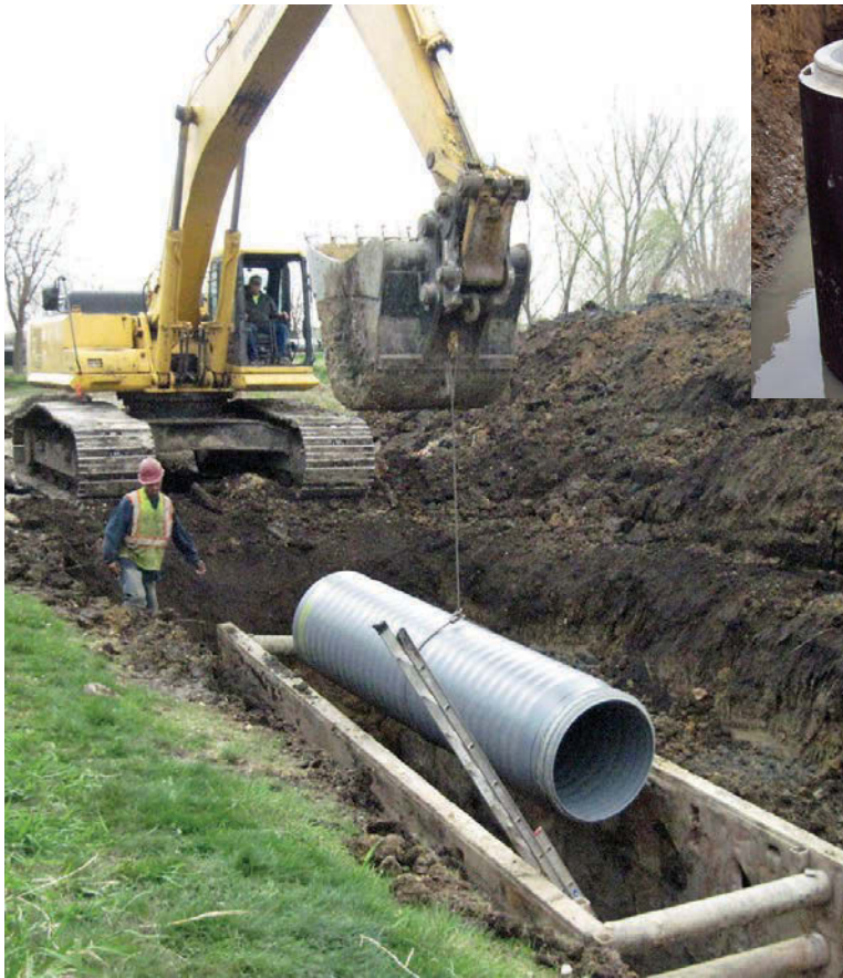
Grimes, Iowa, added a sanitary sewer line due to the overloading of its existing system from heavy rainfall events. Using pipe made from polypropylene reduced project costs and sped up installation.
