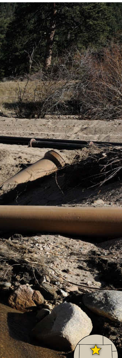
LEFT: New temporary sewer line sections lie ready for connection next to a flood-damaged manhole and a broken section of the original line along Fish Creek. RIGHT: Upper Thompson Sanitation District crew member Dustin Tedder, left, connects a KEG head while Ben Hardendorf holds the line before jetting a section of the original sewer line. (Photography by Eric Lars Bakke)
