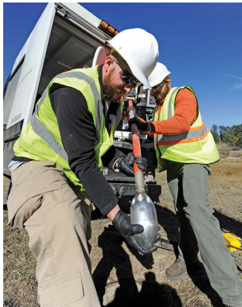
LEFT: New temporary sewer line sections lie ready for connection next to a flood-damaged manhole and a broken section of the original line along Fish Creek. RIGHT: Upper Thompson Sanitation District crew member Dustin Tedder, left, connects a KEG head while Ben Hardendorf holds the line before jetting a section of the original sewer line. (Photography by Eric Lars Bakke)
