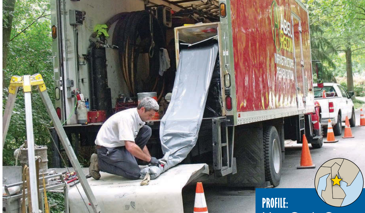
An Abel Recon crew works on a pipe relining project in Wilmington for New Castle County.
