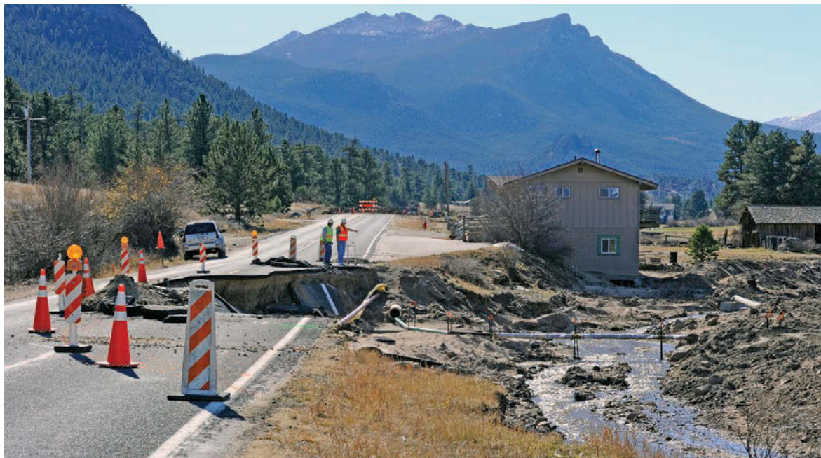
Upper Thompson Sanitation District employees examine the temporary sewer line along Fish Creek.
