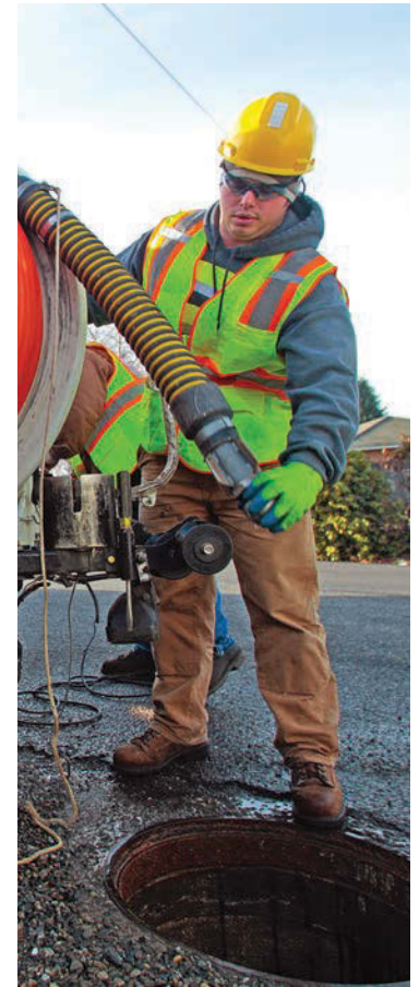
Ryan Hall sets up to clean a sanitary sewer main.
