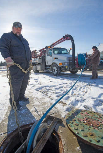
Tom Lafollette, left, and Matt Noe clean a sewer line with the Vector jet/vac combo unit.
