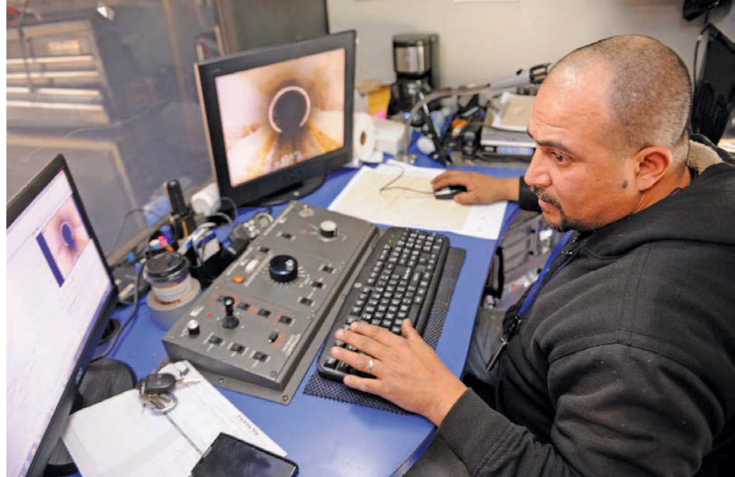
Gerard Cruz, of Compliance Enviro Systems, LLC, out of Baton Rouge, guides a camera through through a pipe inspection from the control room.
