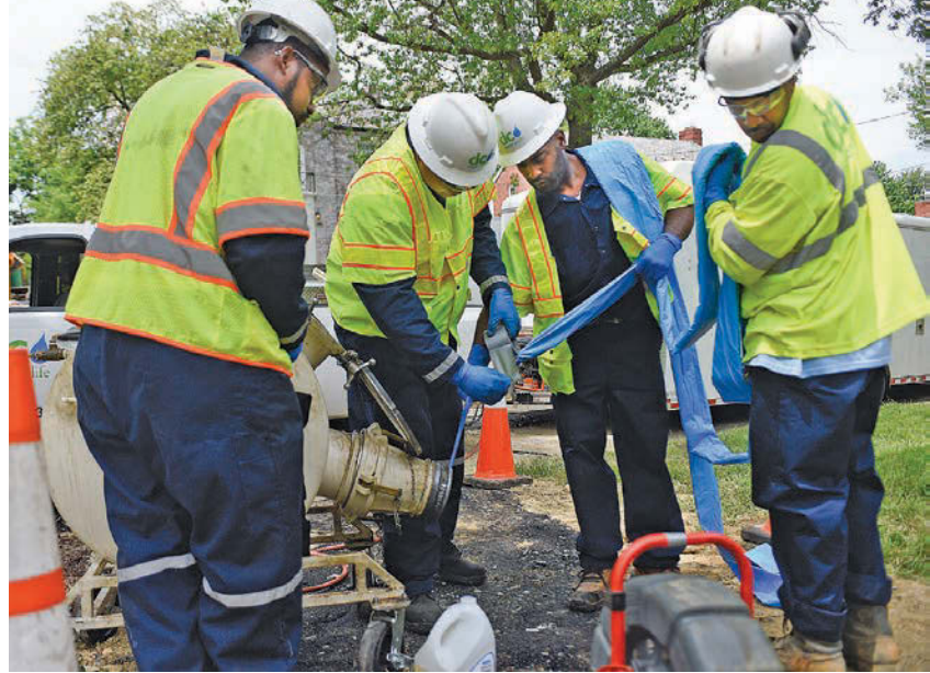
Left: DC Water & Sewer Authority crew member Berone Jones (right) helps pull the calibration tube and liner through the roller, which helps evenly coat the liner with resin before inverting it in the host pipe. Above: Crew members (from left) Jones, Reginald Howell Jr., Tony Lipscombe and Derrick Young prepare a calibration tube and liner for inversion in a lateral line.
