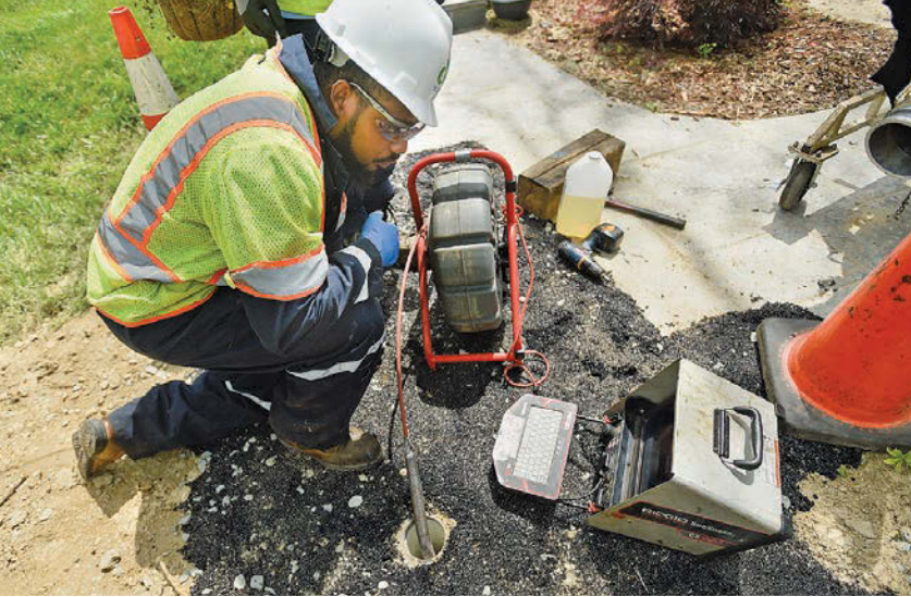
At Left: DC Water & Sewer Authority crew member Berone Jones uses a RIDGID camera system to inspect a lateral before cleaning the line. Above Left: Open-cut lateral replacements were much more common for the utility before it moved to more cured-in-place rehabilitation. Right: An old, rusty pipe is exposed at the start of a residential lateral replacement project.
