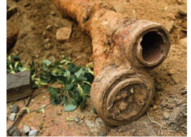
At Left: DC Water & Sewer Authority crew member Berone Jones uses a RIDGID camera system to inspect a lateral before cleaning the line. Above Left: Open-cut lateral replacements were much more common for the utility before it moved to more cured-in-place rehabilitation. Right: An old, rusty pipe is exposed at the start of a residential lateral replacement project.
