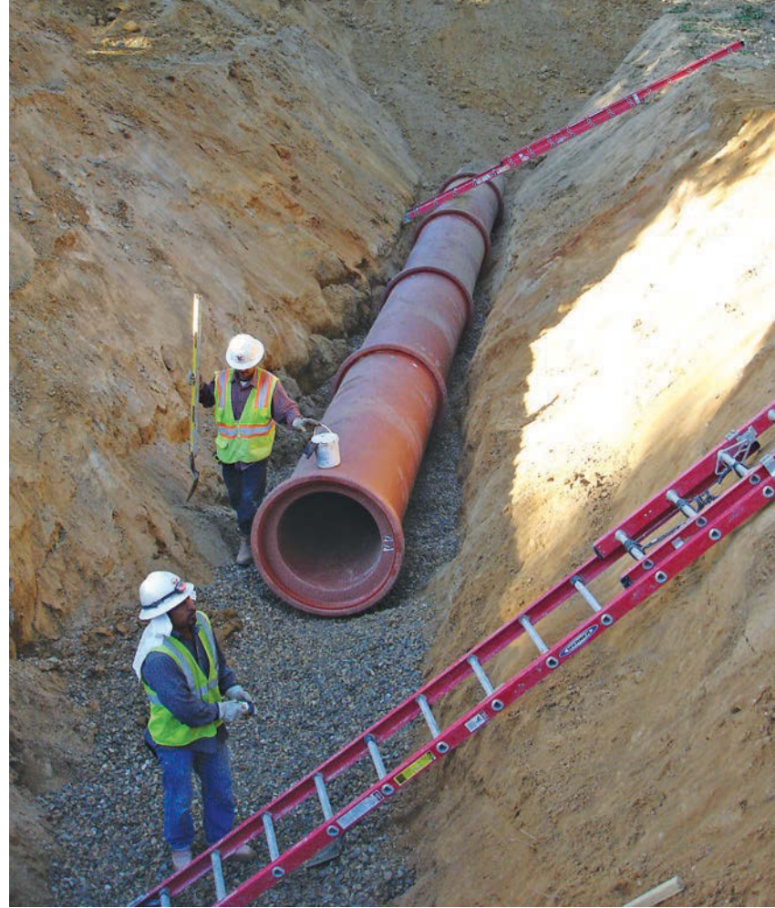
Primarily used in gravity-flow sanitary sewer systems, vitrified clay pipe has improved greatly in recent decades. Computer-controlled kiln firing means the final product is uniform and meets quality standards. (Photo courtesy of National Clay Pipe Institute)
