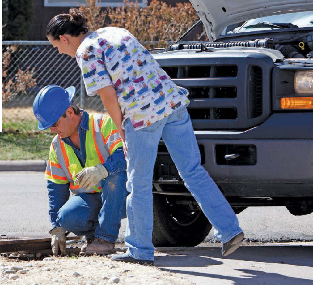
Above: Jeff Romero does a walk-around inspection of the Sycamore Water Tank (capacity 7.75 million gallons). Right: Romero inspects a water meter can with a customer in Los Alamos.
