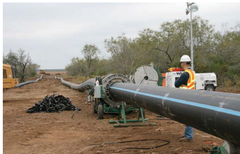
High-density polyethylene pipe has become a popular choice for water and wastewater applications because of its noncorrosive, highly flexible characteristics. And its heat-fused joints mean zero water loss. (Photo courtesy of Plastics Pipe Institute)
