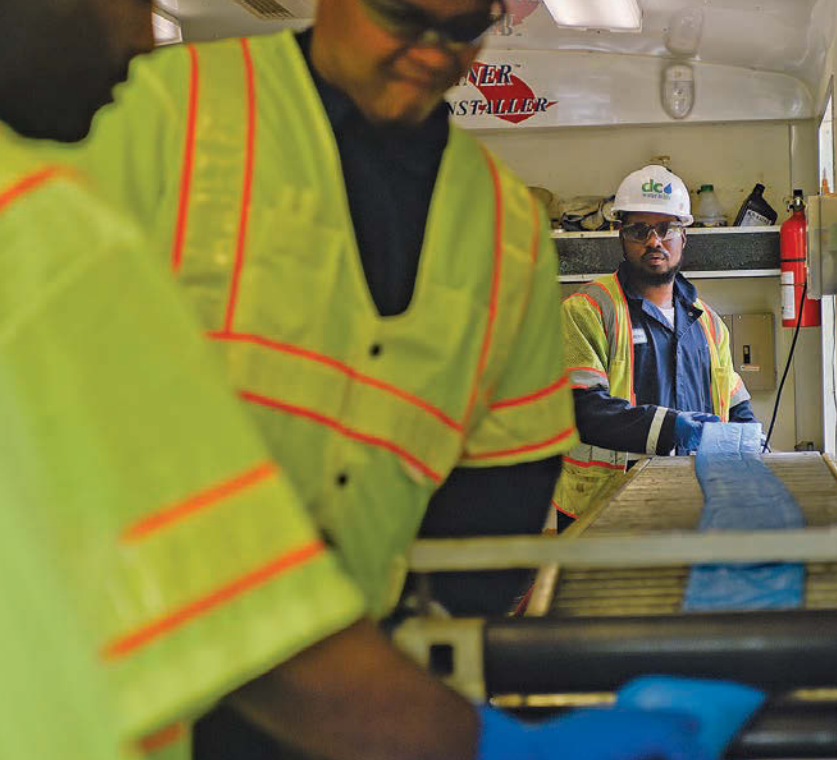
Left: DC Water & Sewer Authority crew member Berone Jones (right) helps pull the calibration tube and liner through the roller, which helps evenly coat the liner with resin before inverting it in the host pipe. Above: Crew members (from left) Jones, Reginald Howell Jr., Tony Lipscombe and Derrick Young prepare a calibration tube and liner for inversion in a lateral line.
