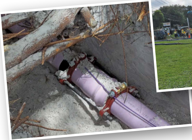
LEFT: This reclaimed water pipe in the City of Altamonte Springs was located under several trees and was found during the Neighborhood Enhancement Program. ABOVE: Public Works and Utilities Department crew members work to repair a force main break. (Photos courtesy City of Altamonte Springs)
