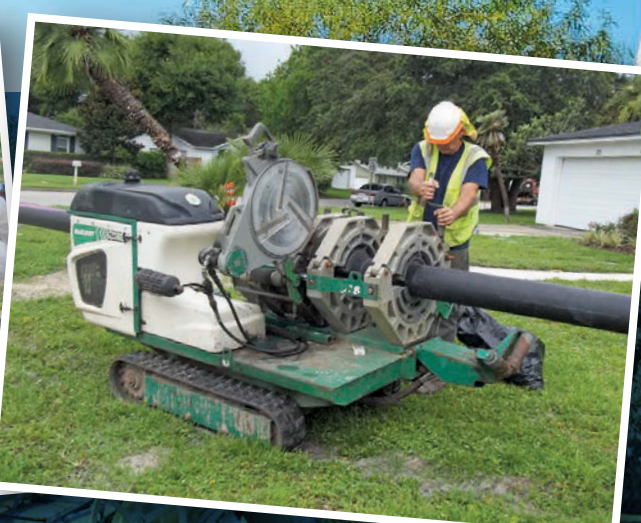
A general view of the water tower near Cranes Roost Park in Altamonte Springs, Fla. Cranes Roost serves as a regional stormwater facility. (Photo by Scott Miller) Far left: A crew from the City of Altamonte Springs Public Works and Utilities Department repairs a broken force main. Left: A crew uses a McElroy fusion machine to join segments of HDPE pipe for a sewer replacement project. (Photos courtesy City of Altamonte Springs)
