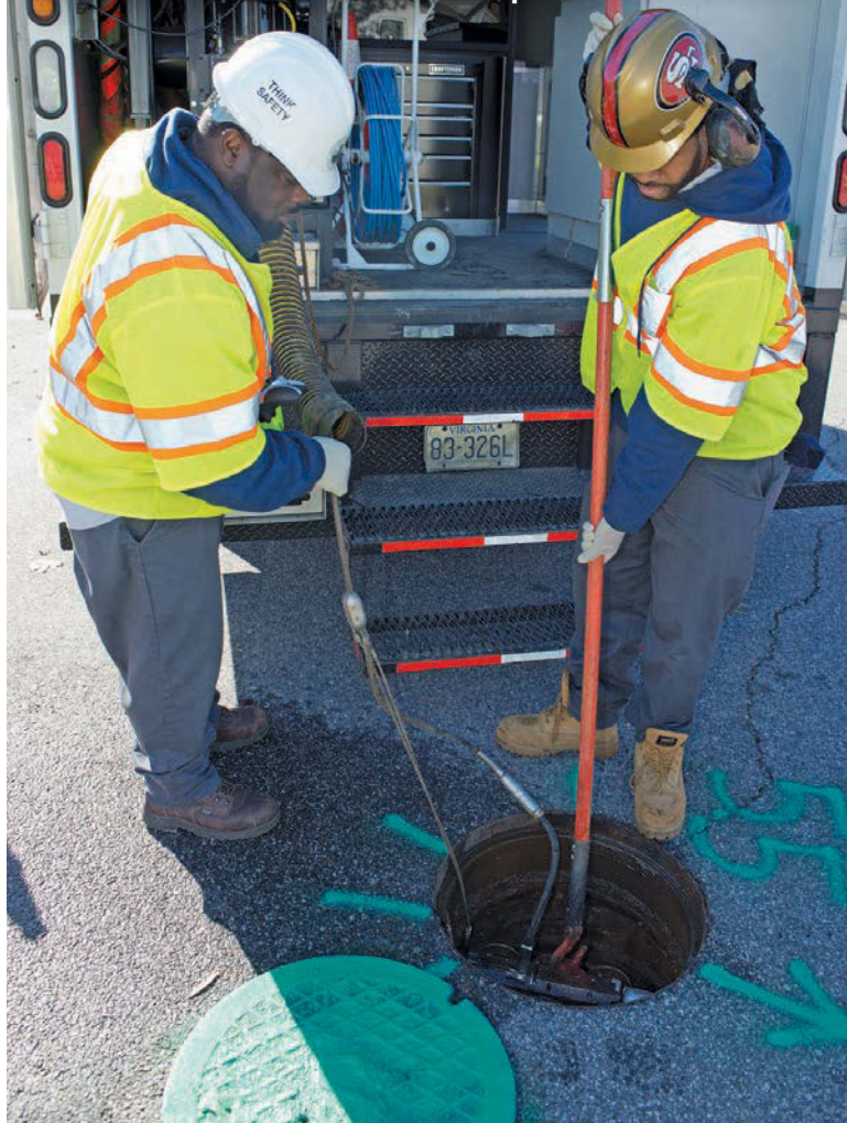
Crew leader Ernest Etheridge (left) and Antwan Young lower a CCTV camera from their CUES-equipped inspection van into a manhole at the start of a sewer line inspection.
